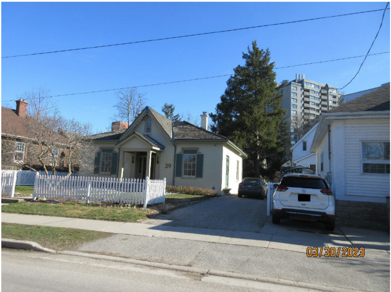
Image 4: Photograph showing the Carfrae Cottage at 39 Carfrae Street.
