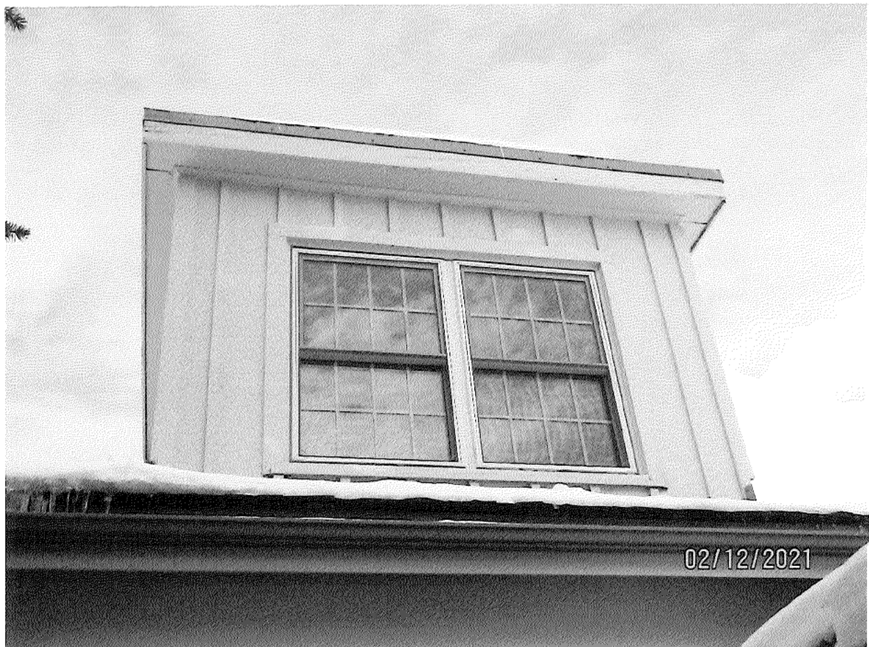
Image 28: Photograph of the shed roof dormer on the south façade of Carrae Cottage.
