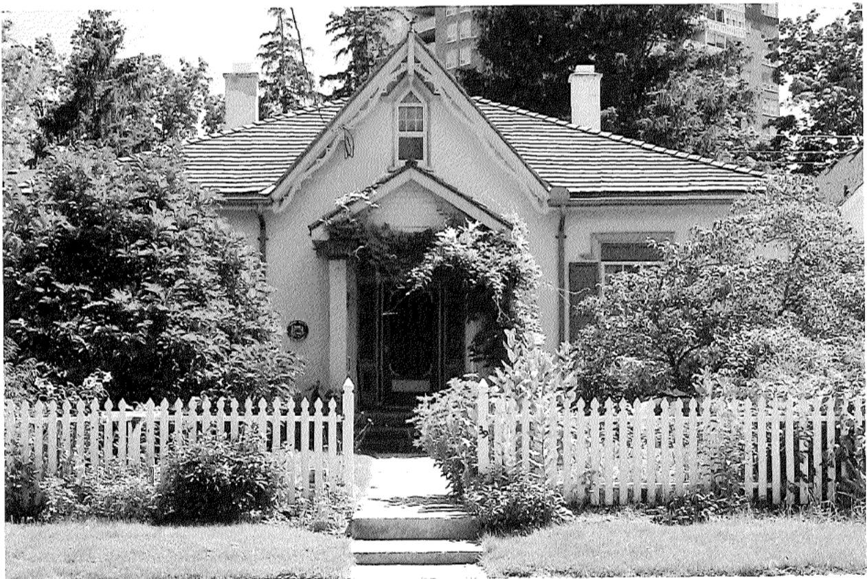
Image 2: Photograph of Carfrae Cottage on July 21, 2015.
