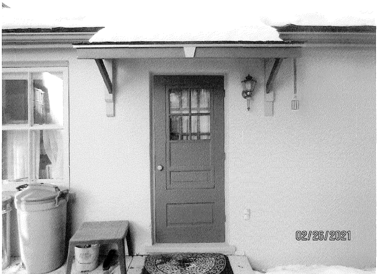
Image 26: Photograph showing the awning over the kitchen doorway as well as the painted storm door.
