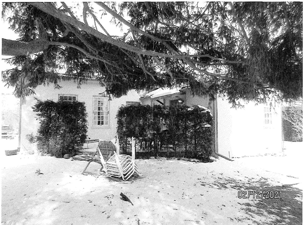
Image 22: View showing the south facade of Carfrae Cottage as well as the kitchen wing.
