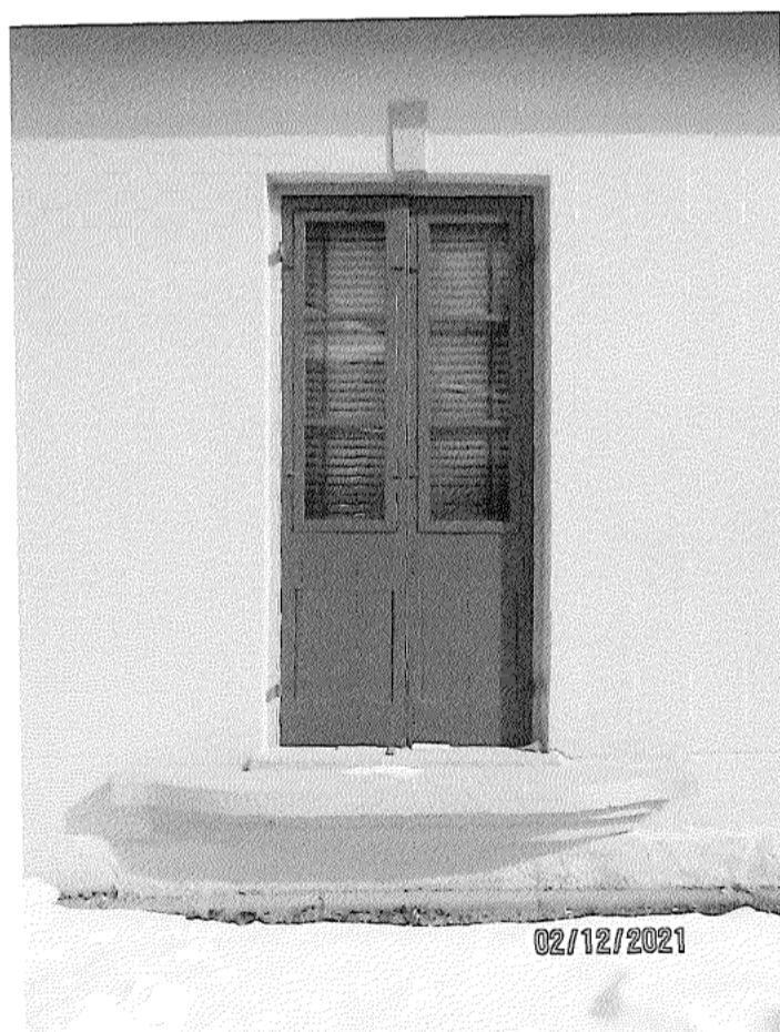
Image 20: Photograph of the painted wood French doors and painted wood storm doors in the northerly opening of the west façade, which retains its cast sill as an indication of the former verandah of Carfrae Cottage. The doorway has a keystone in the parging.
