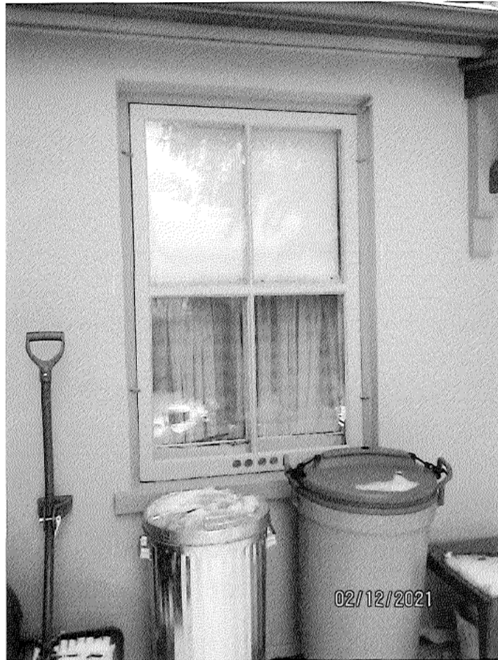
Image 25: Photograph showing the two-over-two painted wood window and storm window in the kitchen wing.
