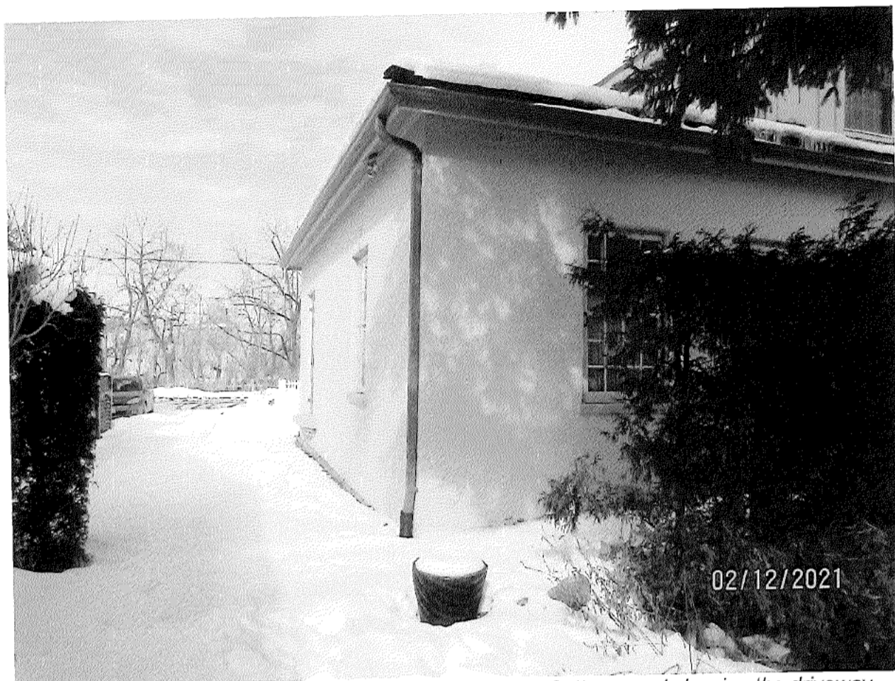
Image 19: View of the west and south facades of Carfrae Cottage, and showing the driveway along the westerly property boundary.
