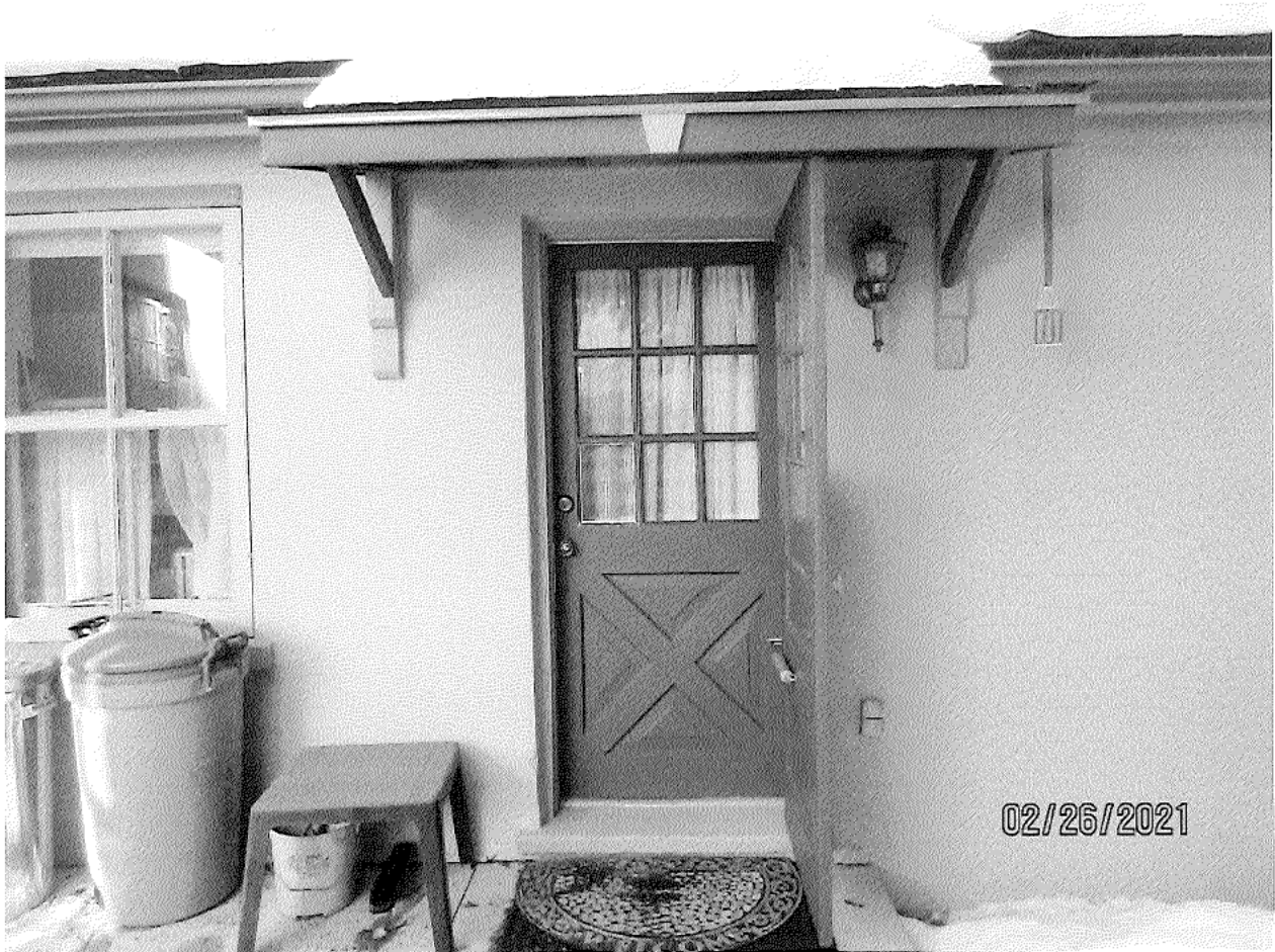
Image 27: Photograph showing the painted wood kitchen door, with nine lites and X-pattern panelling below.
