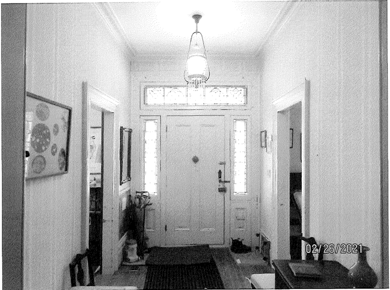
Image 35: Photograph showing the Centre hall, looking towards the front doorway of Carfrae Cottage. Note the baseboards, casing, and crown moulding.
