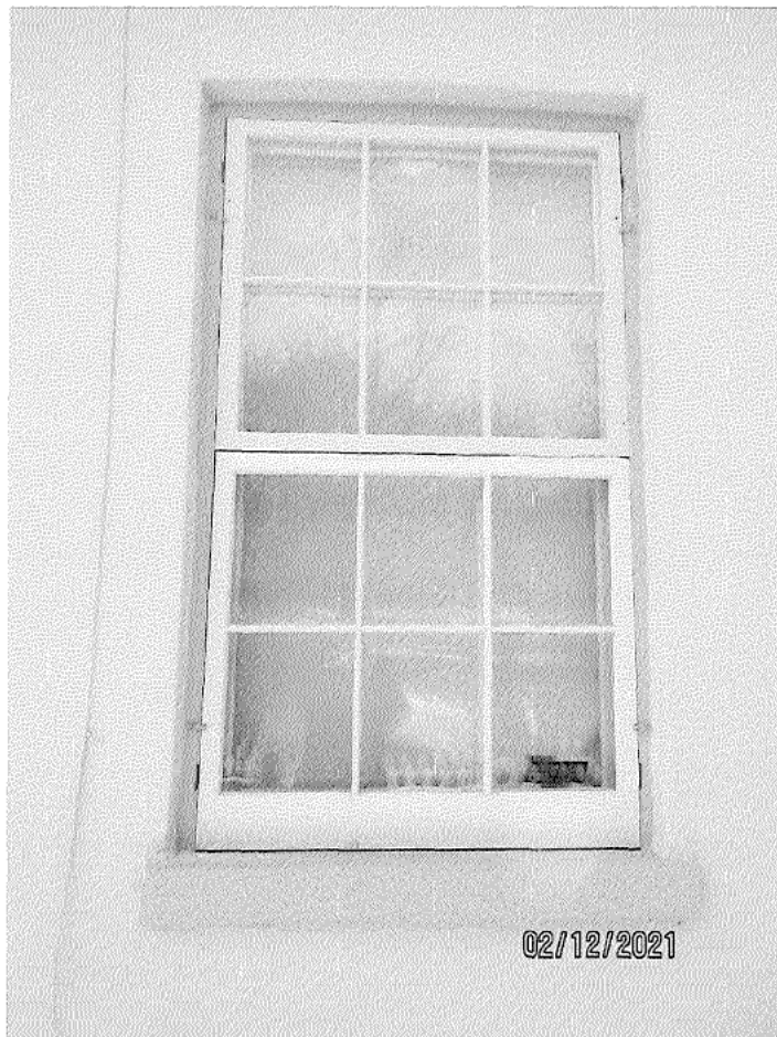
Image 33: Photograph of the six-over-six painted wood window with matching storm windows and an aluminum-clad sill.
