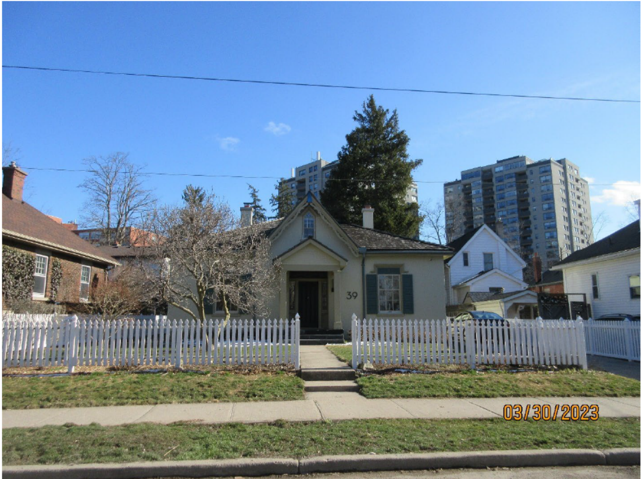
Image 3: Photograph showing the Carfrae Cottage at 39 Carfrae Street.
