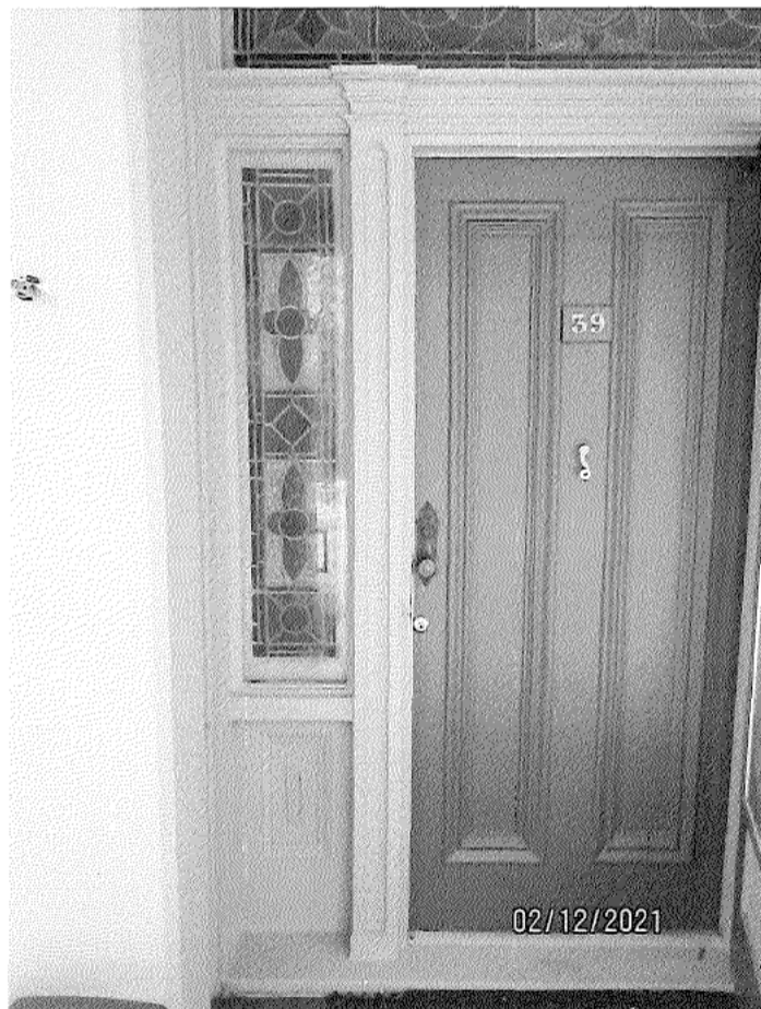
Image 12: Photograph showing the front doorway with single leaf, painted wood door with two long panels (which is believed to be original to the house), set in a rectangular opening with rectangular sidelights to both sides, a panelled dado below, and a rectangular transom. The sidelights and transom feature stained glass in repetitive geometric patterns with coloured and textured glass. The doorway is recessed in the façade with a plain reveal. The door opening is framed by pilasters with a Gothic point, with entablature supporting the architectural framework of the doorway.
