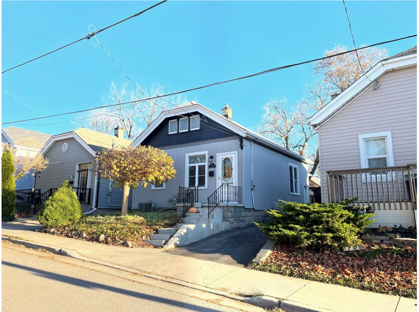
Photograph 14: View of the east elevation of the house and driveway, 3 Kennon Place (AECOM, November 2022)
