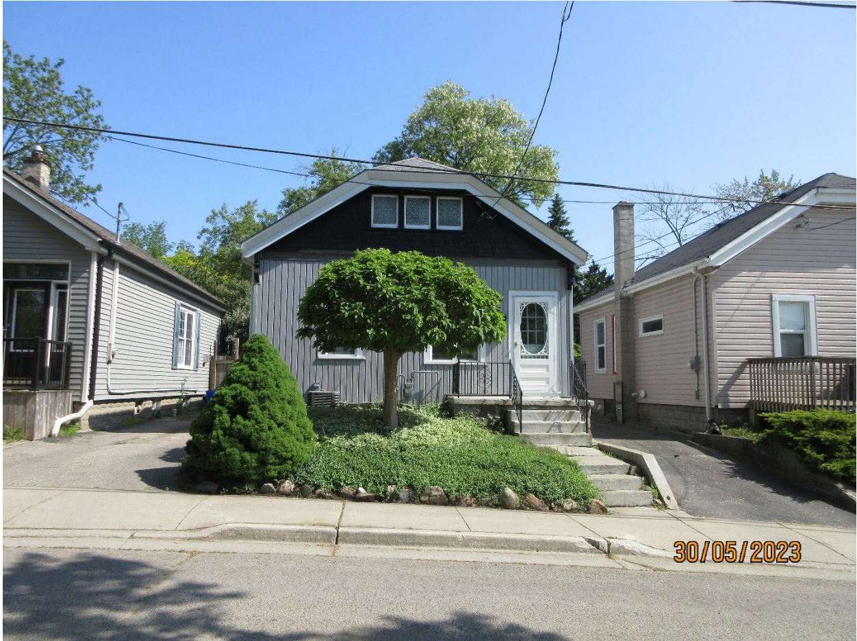
Image 3: Photograph of the dwelling located on the subject property at 3 Kennon Place, May 30, 2023.
