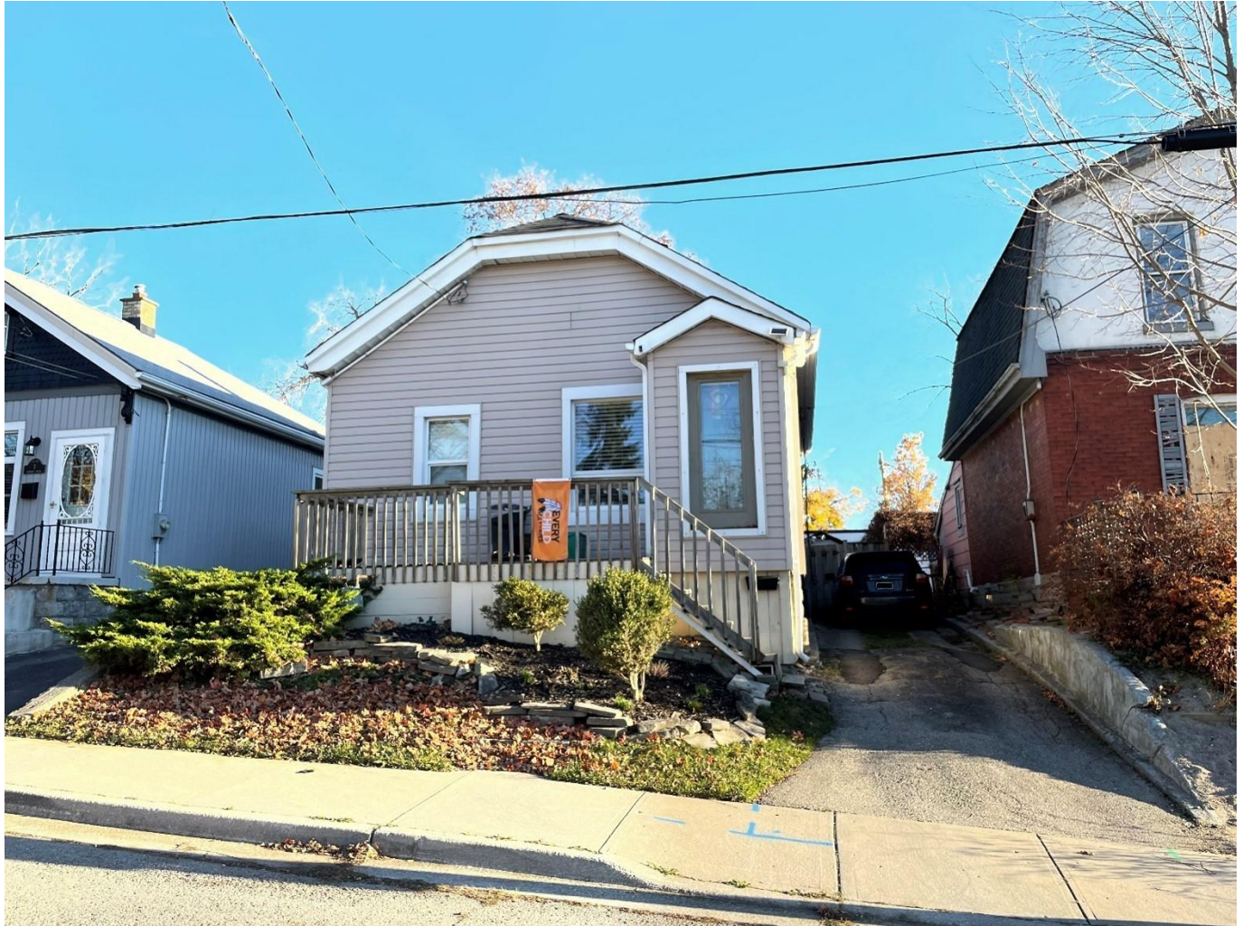
Photograph 5: Front (north) façade, 2 Kennon Place (AECOM, November 2022)
