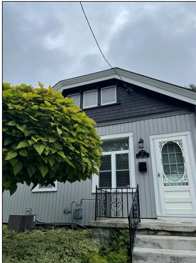
Photograph 9: Detail of 3 Kennon Place showing attic windows and shingle cladding in gable (AECOM, September 2022)
