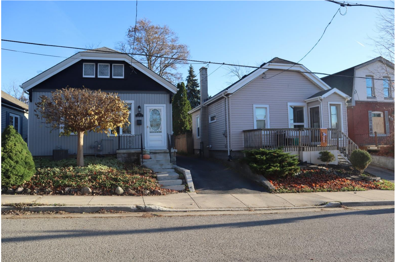
Photograph 1: View of 2 Kennon Place (right) and 3 Kennon Place (left) (AECOM, November 2022)
