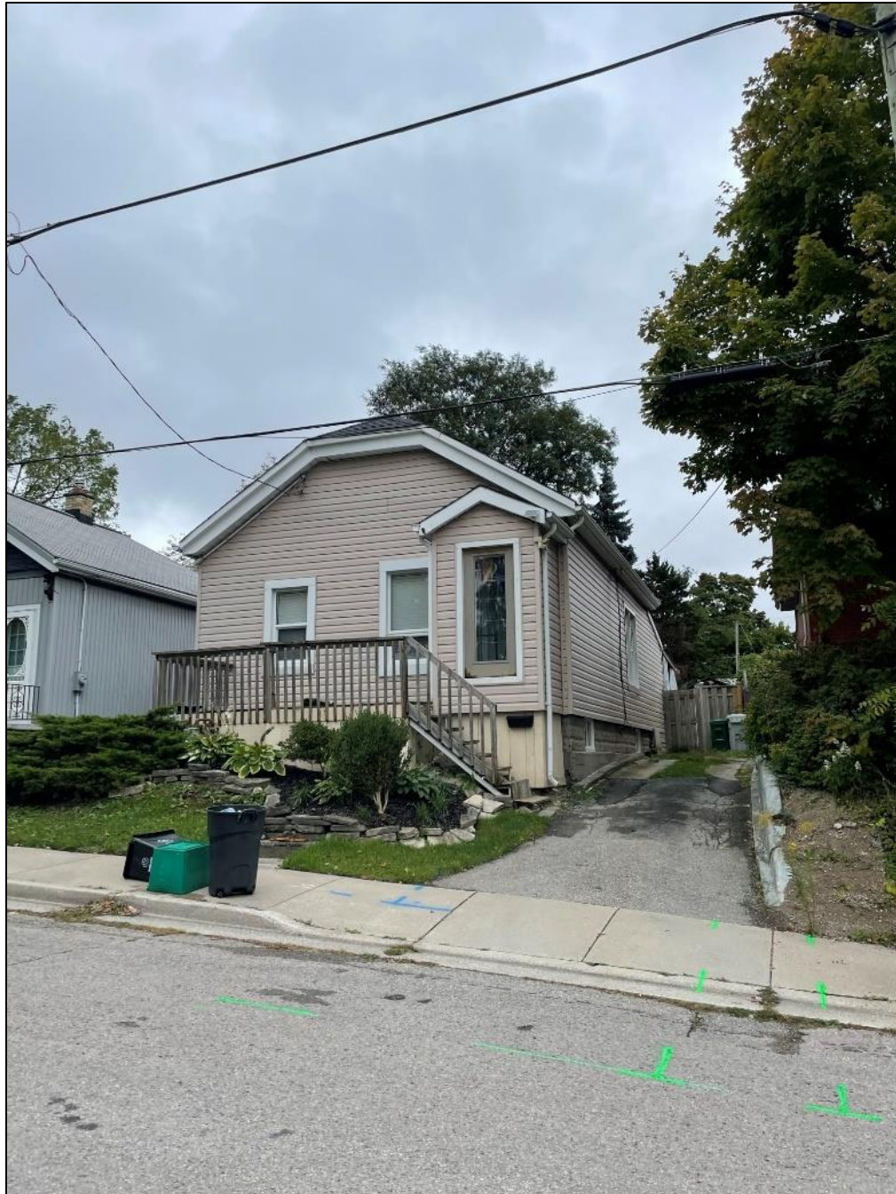
Photograph 6: View showing driveway and west side of house, 2 Kennon Place (AECOM, September 2022)
