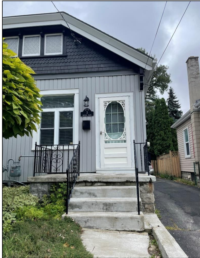
Photograph 12: Porch and front entrance of 3 Kennon Place (AECOM, September 2022)
