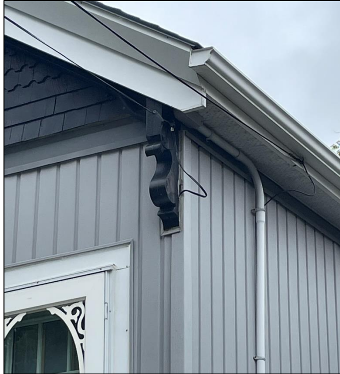
Photograph 11: Detail of decorative bracket, 3 Kennon Place (AECOM, September 2022)
