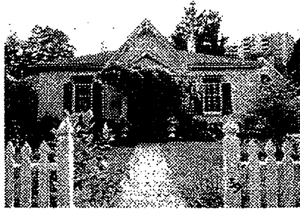
Carfrae Cottage 39 Carfrae Street Built c.1860
