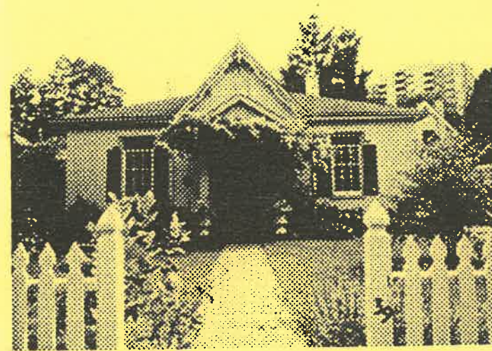
Carfrae Cottage 39 Carfrae Street Built c.1860
