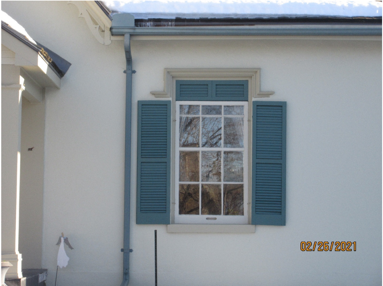
Image 17: Photograph showing the westerly front window, storm window, wood shutters, label, and sill of the front (north) façade of Carfrae Cottage.
