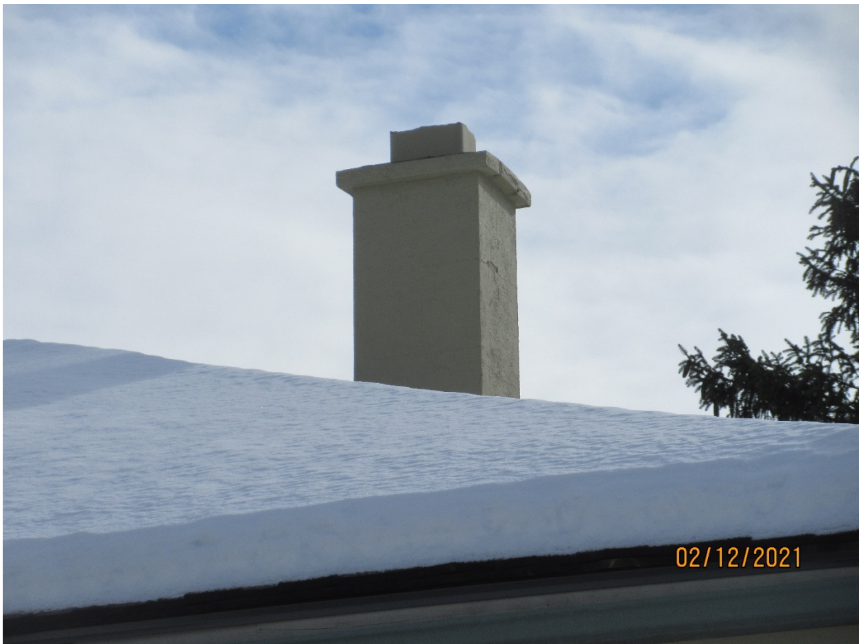
Image 8: Photograph of the west chimney, as seen from Carfrae Street.
