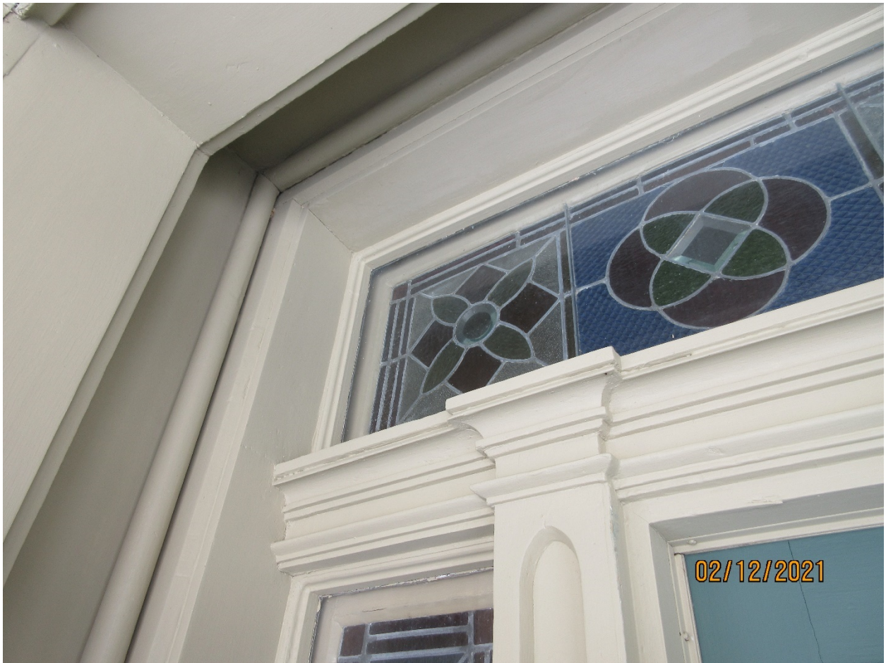
Image 13: Detail photograph showing the entablature of the doorway with Gothic pointed pilaster, as well as a detail of the stained glass transom.
