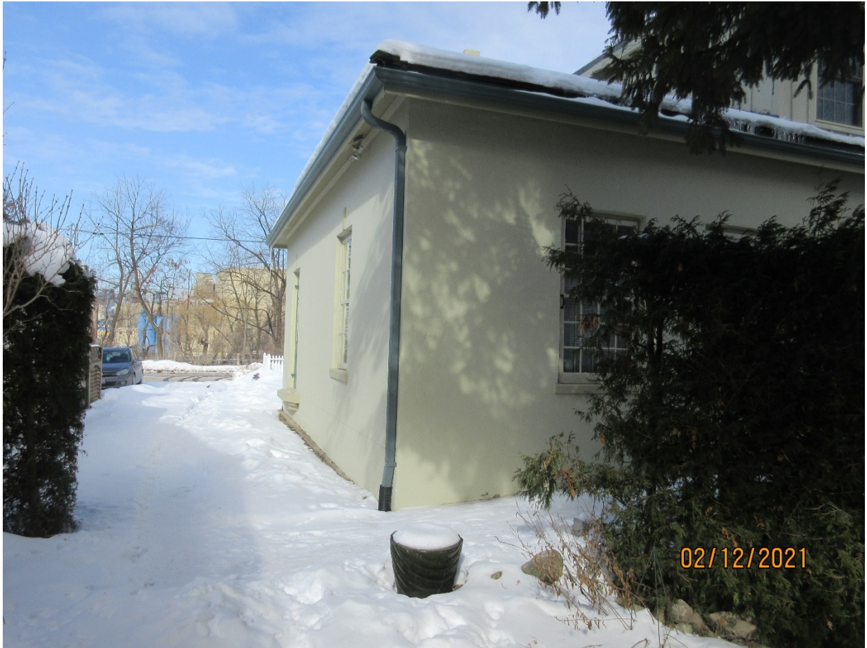
Image 19: View of the west and south facades of Carfrae Cottage, and showing the driveway along the westerly property boundary.
