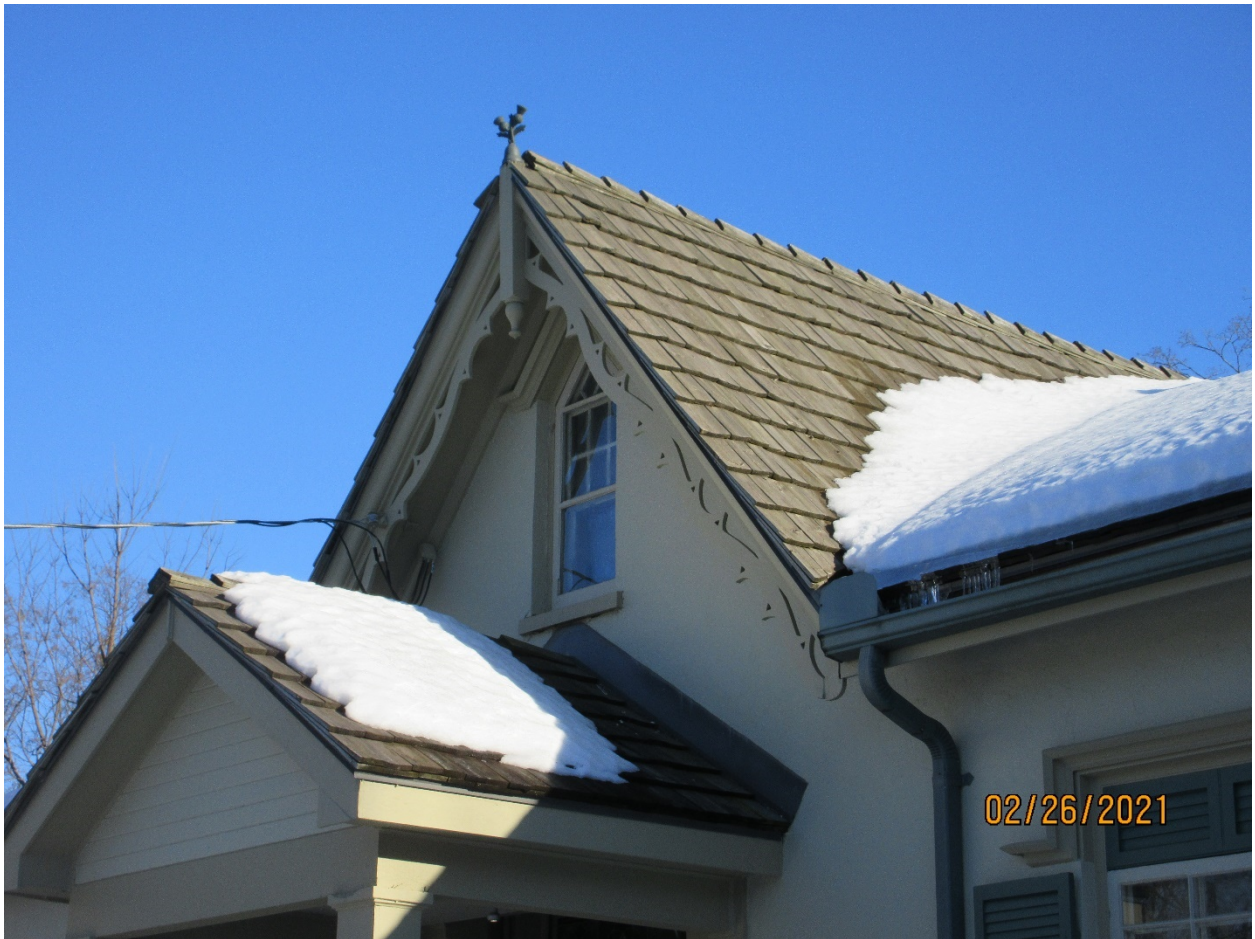
Image 18: View of the central gable dormer on the front (north) facade of Carfrae Cottage with a primitive Gothic pointed wood window and matching storm window. The decorative wood bargeboard of the central gable dormer is also shown, as well as the Scotch thistle.
