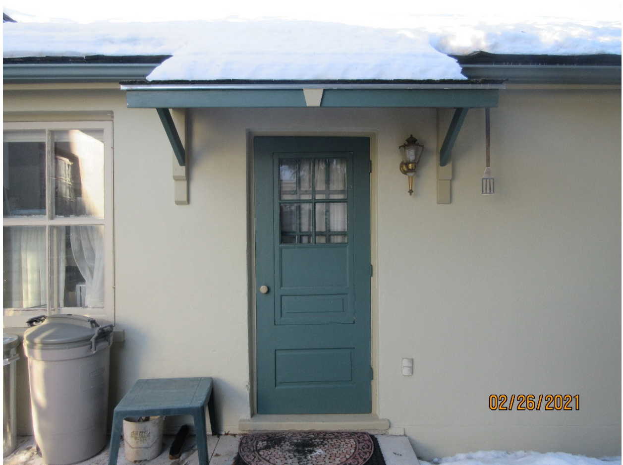
Image 26: Photograph showing the awning over the kitchen doorway as well as the painted storm door.
