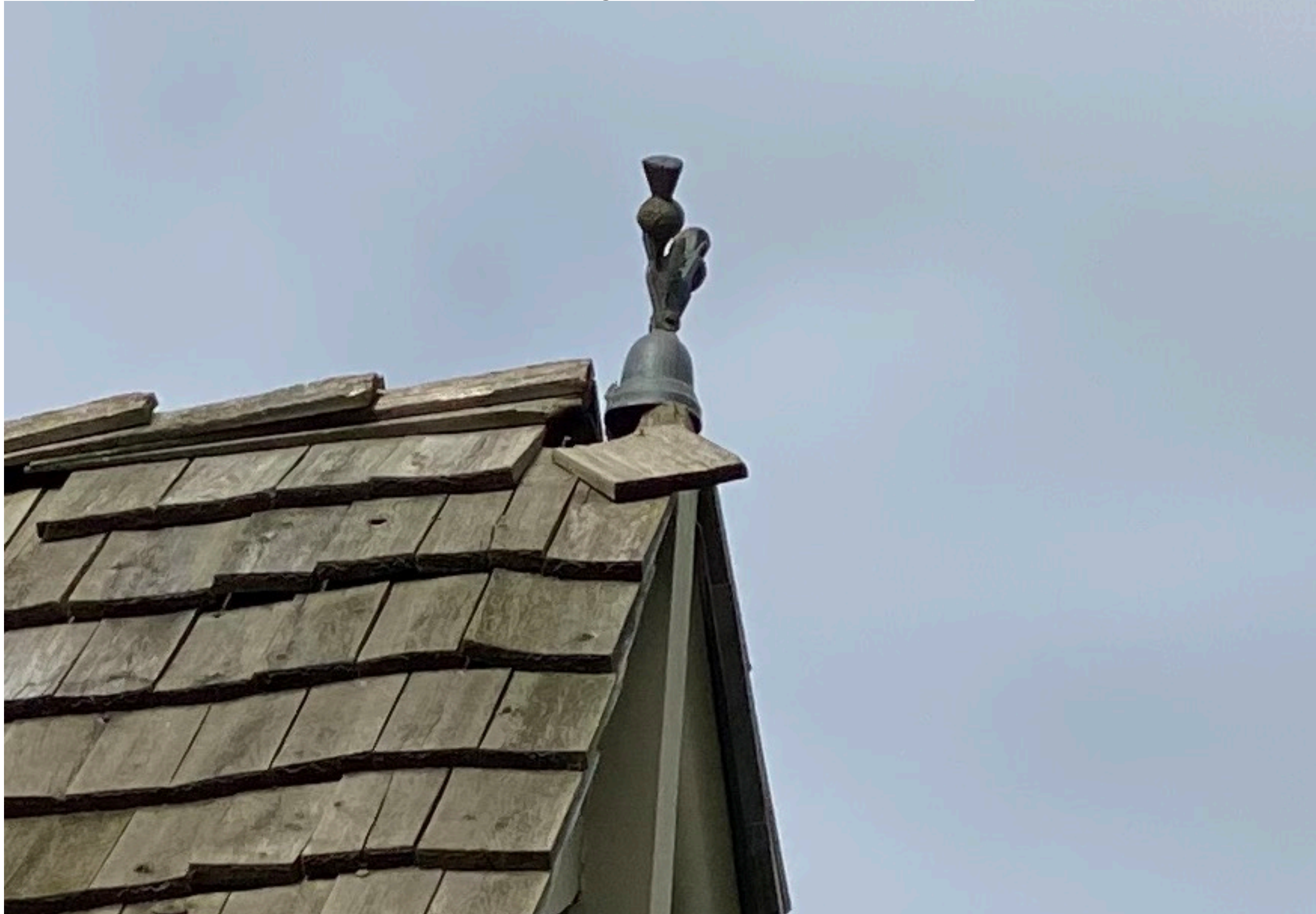
Pine shakes in such bad shape exposing home to the elements
