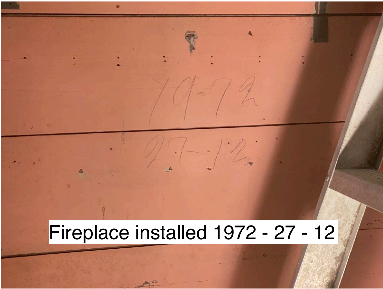
The hearth tiles were installed over wood - does not meet code.
