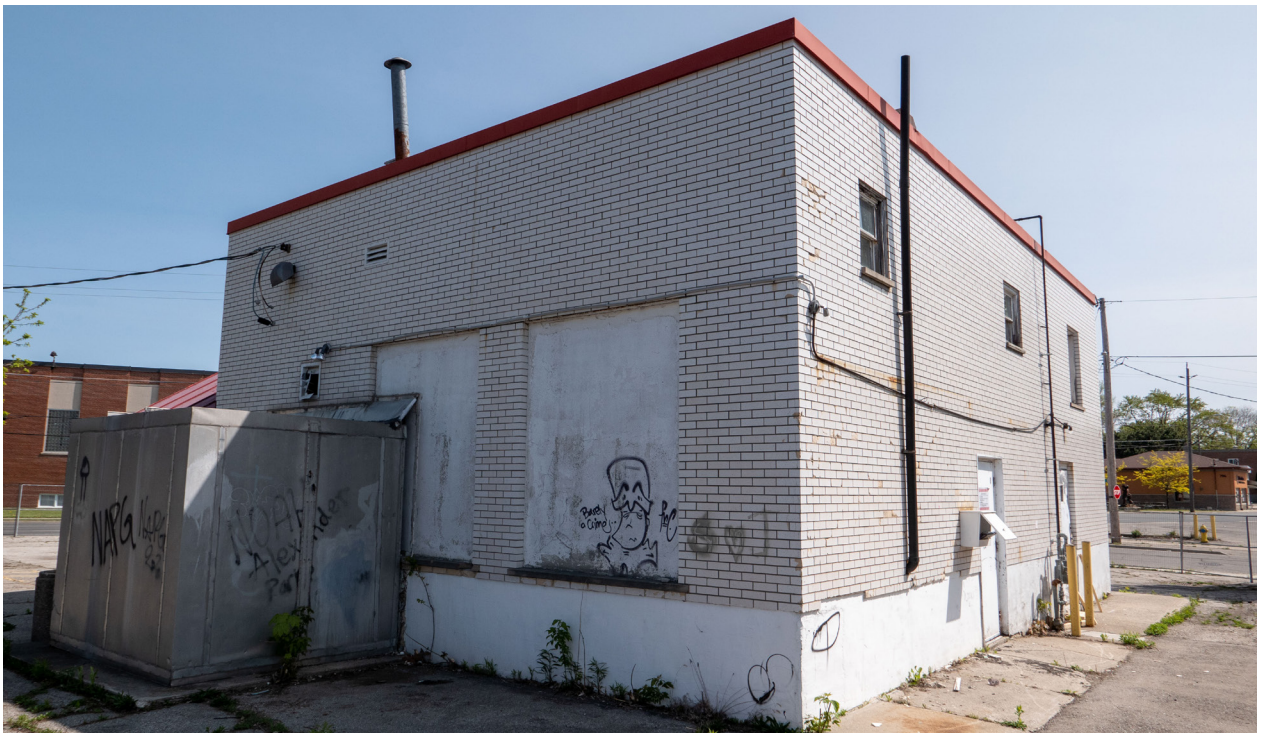
Figure 6: View of the former restaurant's west and south elevations. The blind openings at centre are remnants from the original service centre's steel sash windows (CBCollective 2023).
