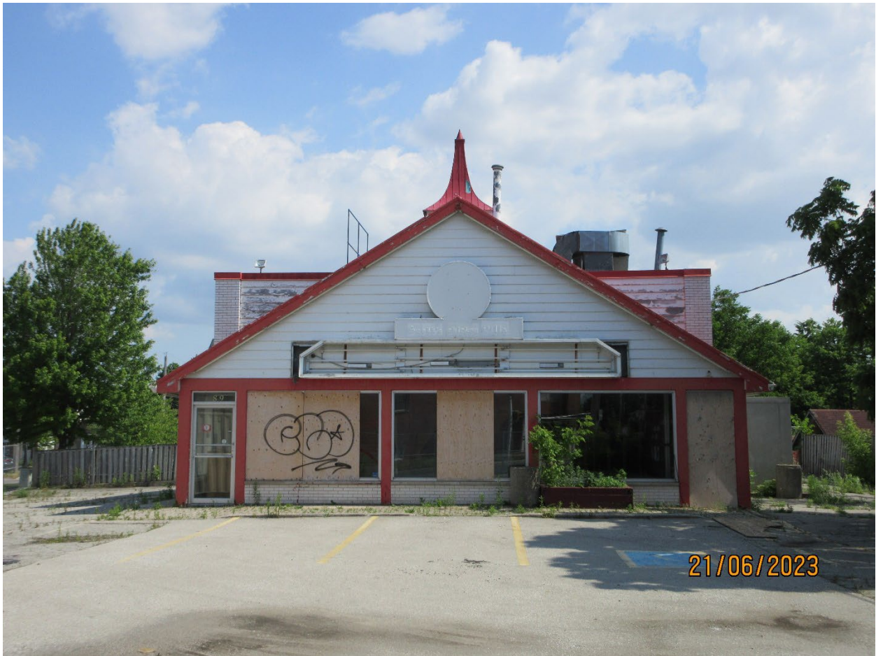
Image 1: North elevation of the building on the subject property at 689 Hamilton Road, June 21, 2023.
