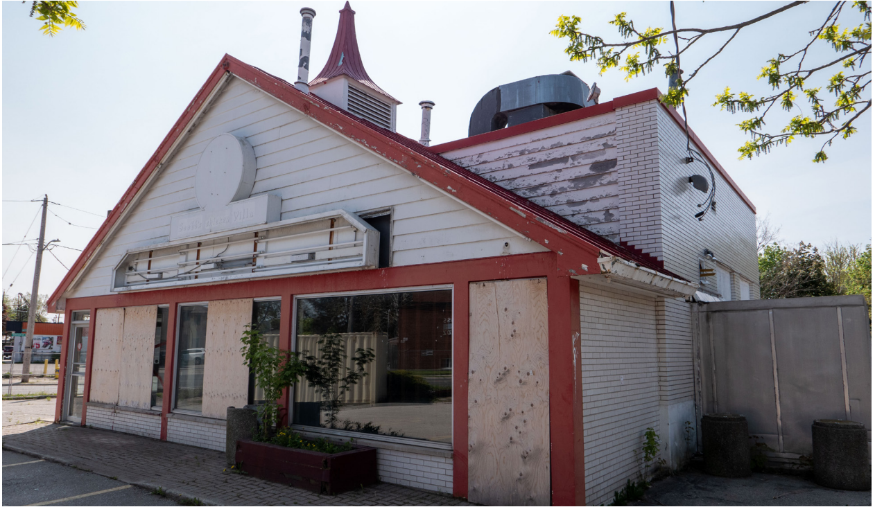
Figure 7: Southwest view of the building's north elevation, including the gabled addition, and siding applied to the original mass (CBCollective 2023).
