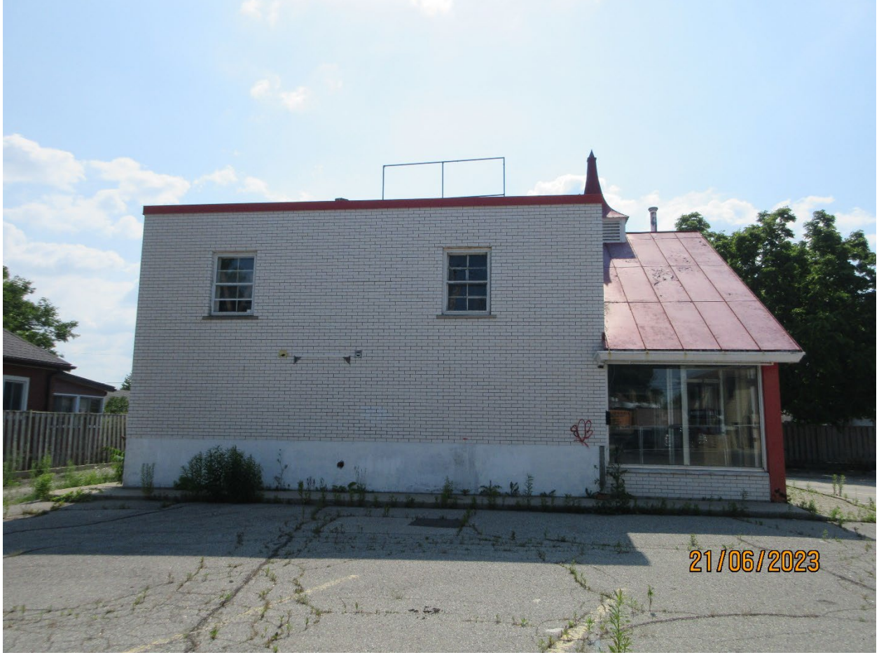
Image 4: East elevation of the building on the subject property at 689 Hamilton Road, June 21, 2023.
