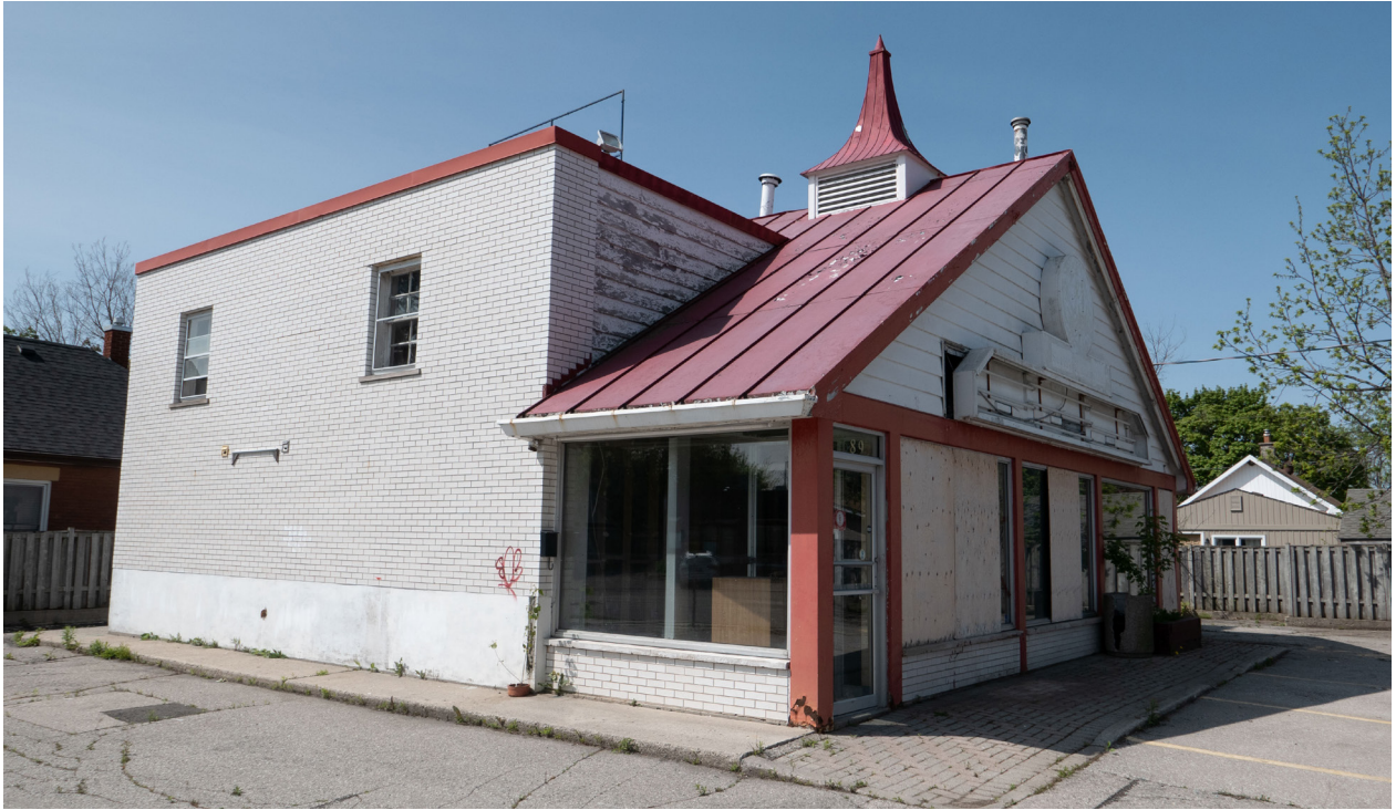
Figure 11: Photograph showing the form and details of the front gable portion, added when the building was converted to a restaurant (CBCollective 2023).
