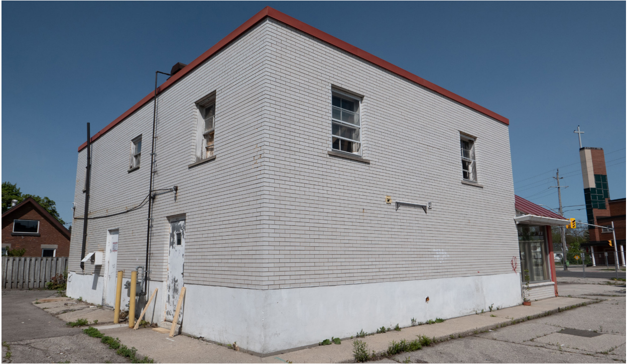
Figure 5: View of the former restaurant's east and south elevations (CBCollective 2023).
