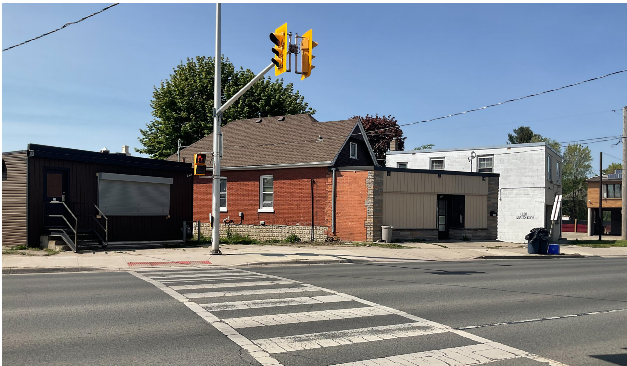
Figure 2: Three modest building located directly east of the subject property (CBCollective 2023).
