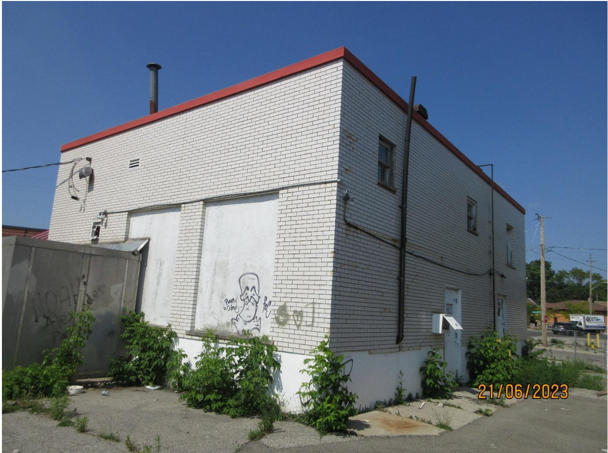
Image 5: West and south elevations of the building on the subject property showing large original window openings on the original 1947 portion of the building, June 21, 2023.
