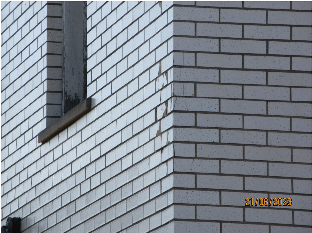
Image 6: Enameled brick showing buff brick material beneath on the original 1947 portion of the building on the subject property at 689 Hamilton Road, June 21, 2023.
