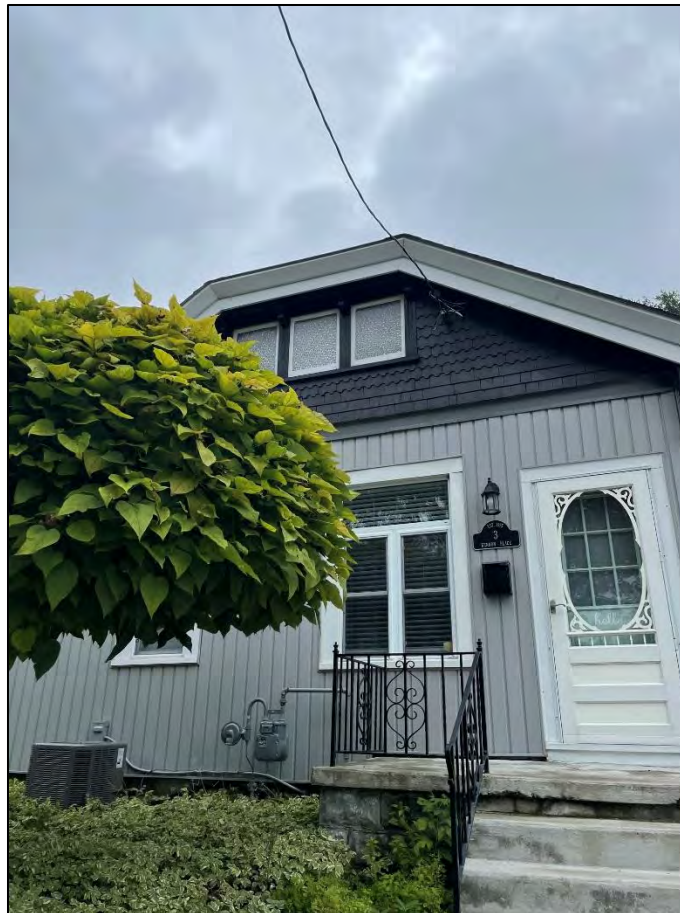
Photograph 9: Detail of 3 Kennon Place showing attic windows and shingle cladding in gable (AECOM, September 2022)
