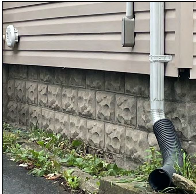
Photograph 3: Detail of rusticated concrete block foundation, 2 Kennon Place (AECOM, September 2022)
