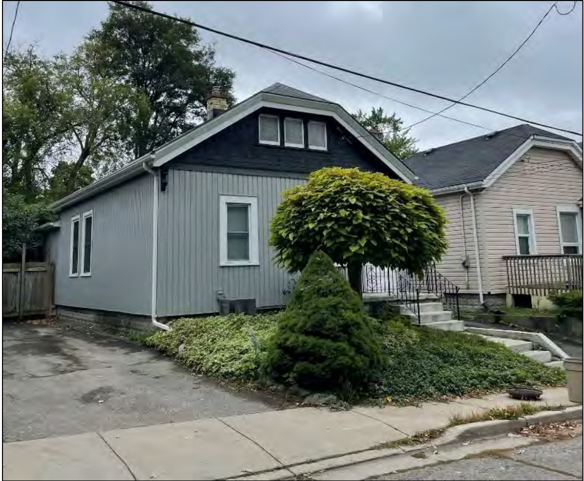
Photograph 13: View showing west elevation of the house, 3 Kennon Place (AECOM, September 2022)
