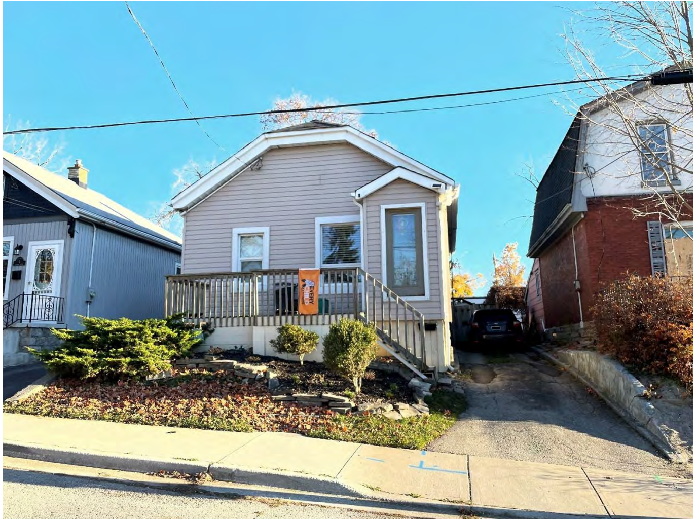
Photograph 5: Front (north) façade, 2 Kennon Place (AECOM, November 2022)
