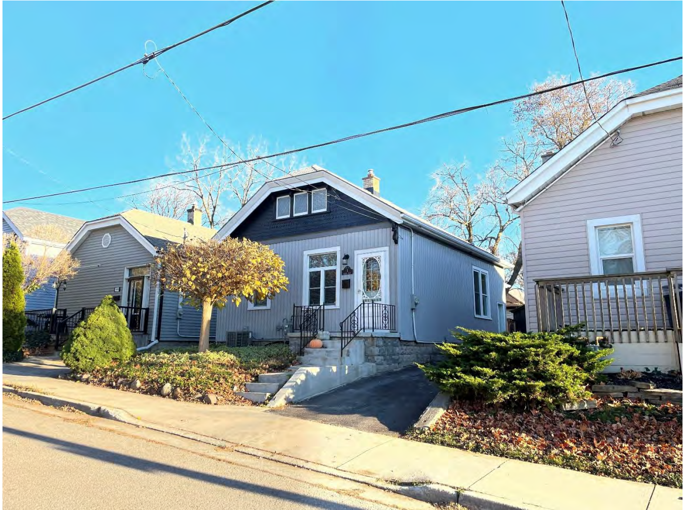
Photograph 14: View of the east elevation of the house and driveway, 3 Kennon Place (AECOM, November 2022)
