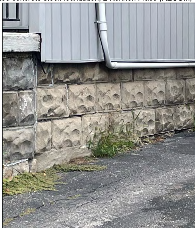
Photograph 4: Detail of rusticated concrete block foundation, 3 Kennon Place (AECOM, September 2022)
