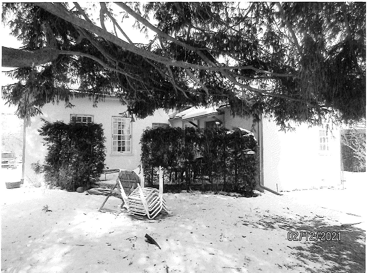
Image 22: View showing the south facade of Carfrae Cottage as well as the kitchen wing.
