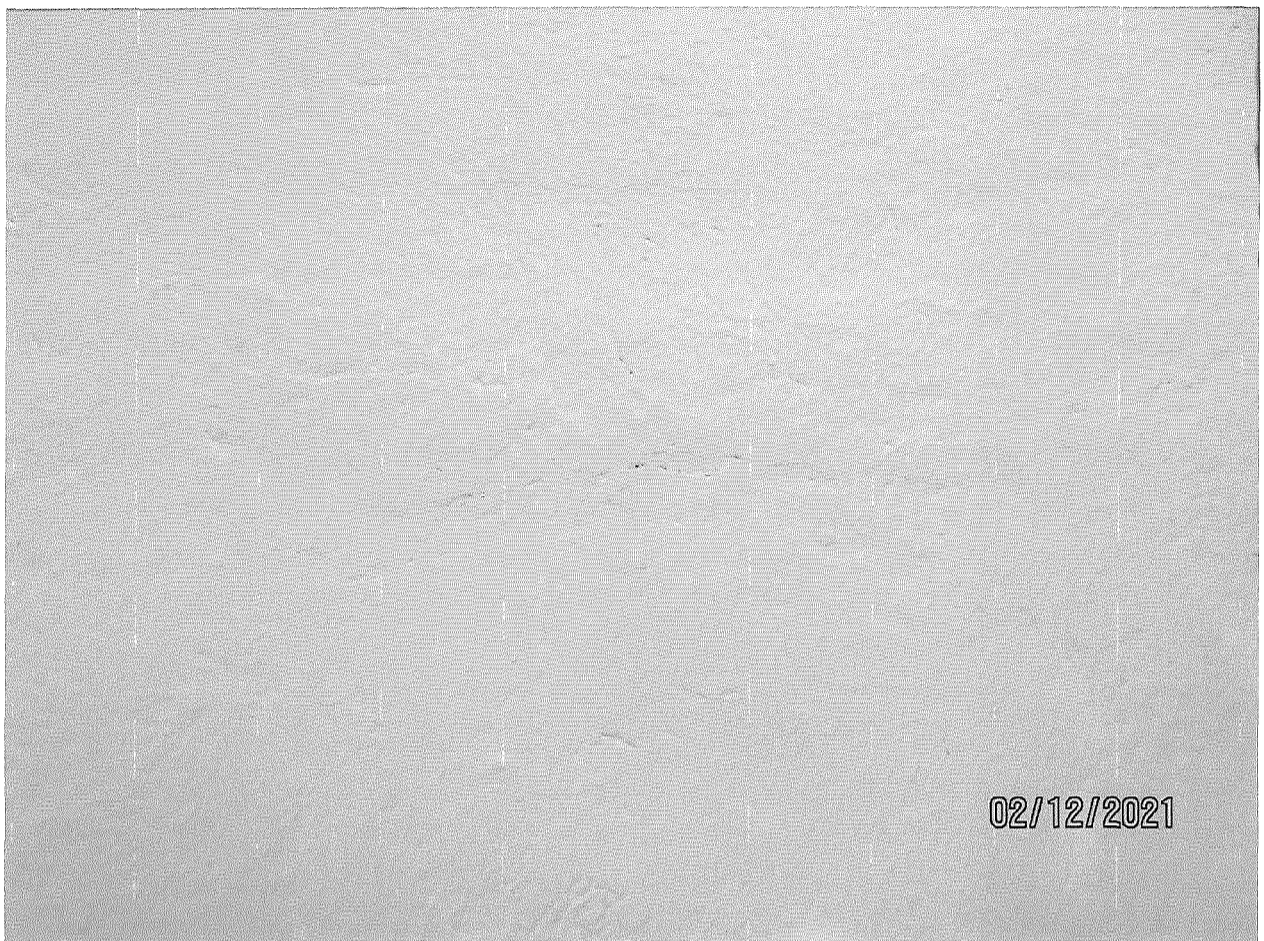
Image 11: Photograph, showing a representative example, of the traditional stucco parging (cementitious smooth textured exterior 'stucco' finish) over the double brick construction of Carfrae Cottage.
