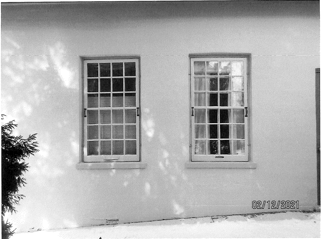
Image 23: Photograph showing the two twelve-over-twelve painted wood windows with storm windows and wooden sills on the south façade of Carfrae Cottage.
