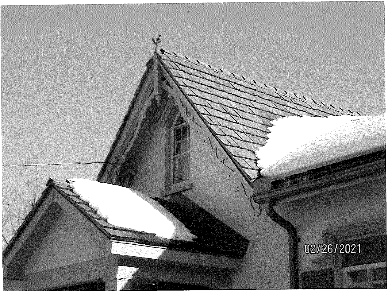
Image 18: View of the central gable dormer on the front (north) façade of Carfrae Cottage with a primitive Gothic pointed wood window and matching storm window. The decorative wood bargeboard of the central gable dormer is also shown, as well as the Scotch thistle.
