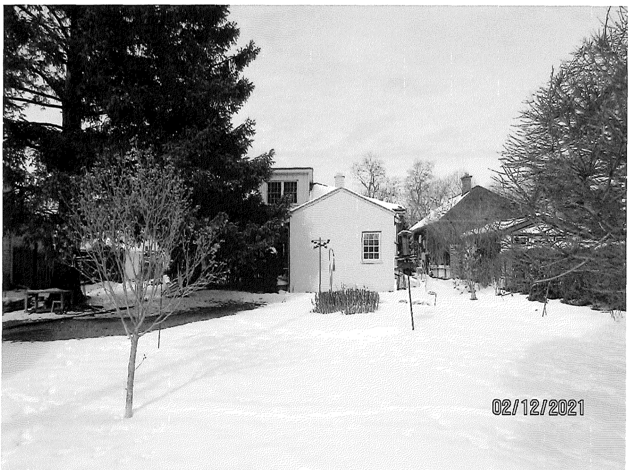
Image 30: View of the south façade of Carfrae Cottage, as seen from the rear (southerly) property boundary along Ardaven Place.
