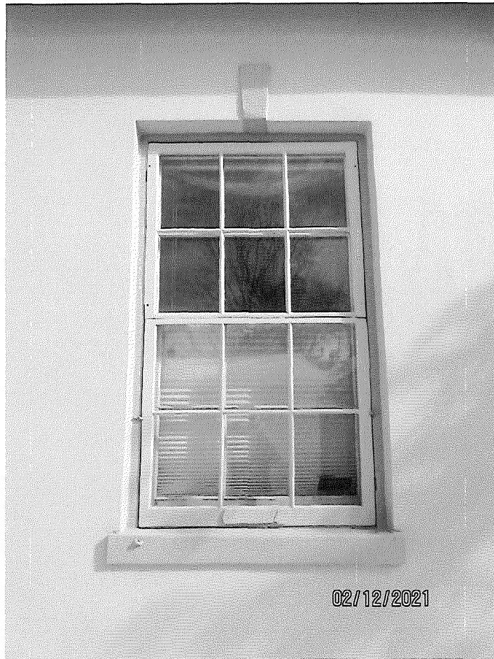
Image 21: Photograph of the painted wood six-over-six shingle hung wood window with storm windows that replicate the six-over-six fenestration. The window opening has a keystone in the parging and a wood sill.
