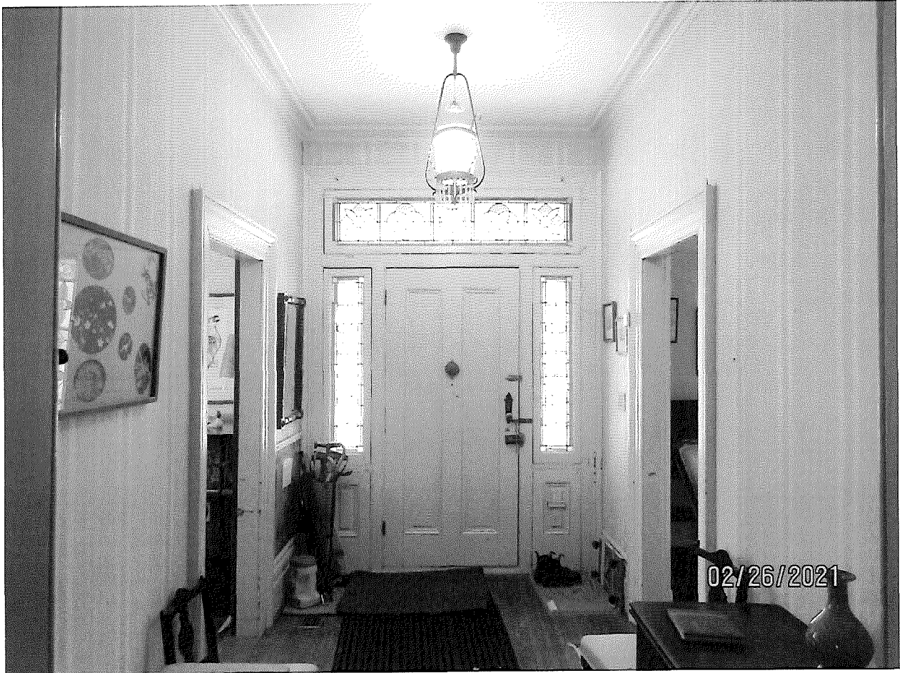
Image 35: Photograph showing the Centre hall, looking towards the front doorway of Carfrae Cottage. Note the baseboards, casing, and crown moulding.
