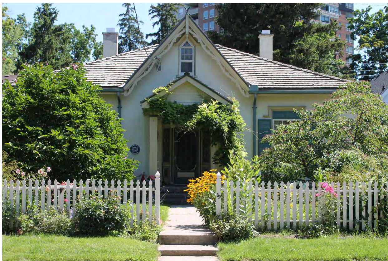
Image 2: Photograph of Carfrae Cottage on July 21, 2015.
