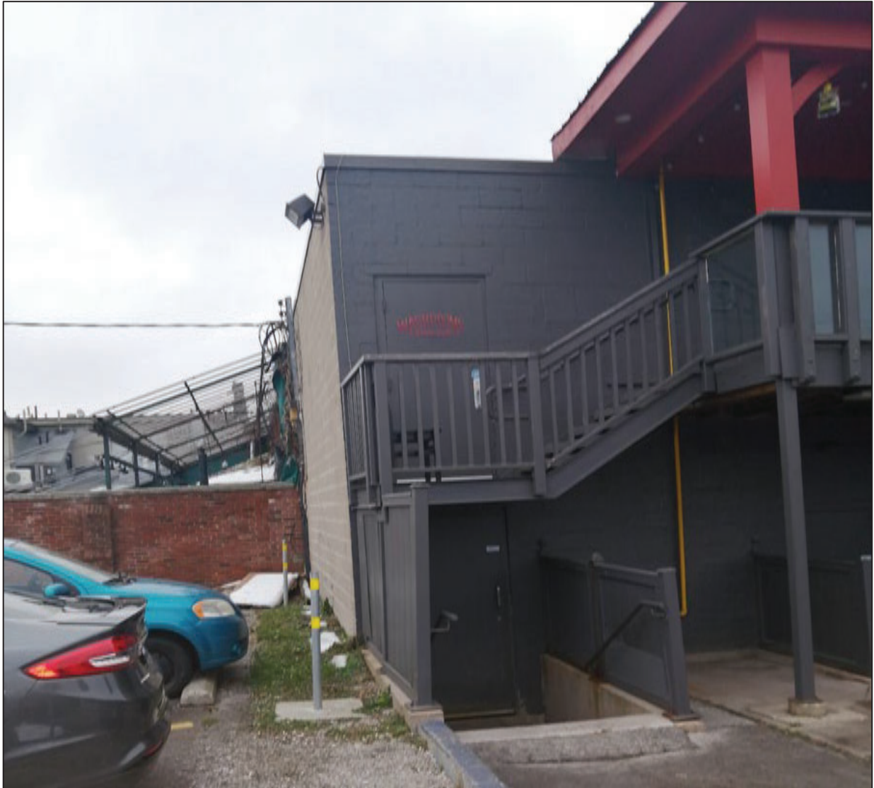
Figure 43: View of north elevation (Source: MHBC, 2020).
