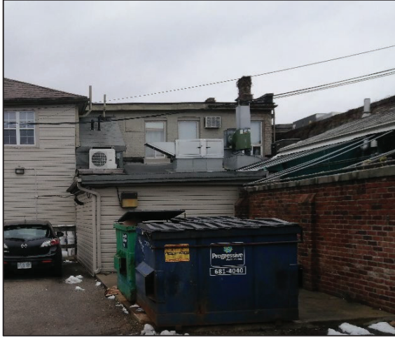
Figure 23: View of west elevation (Source: MHBC, 2020).
