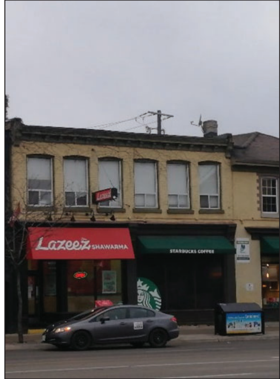
Figure 22: View of front façade From Victoria Park
