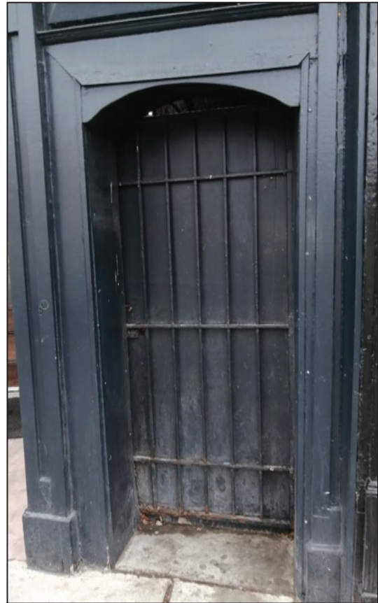
Figure 39: View of door opening/ access that leads to alleyway to brick ancillary structure to the rear of 595 Richmond Street (Source: MHBC, 2020).
