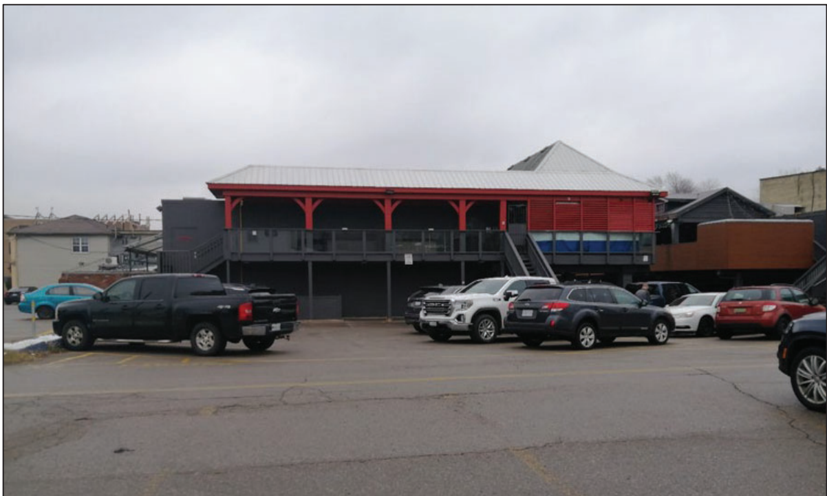
Figure 42: West elevation of 595 Richmond Street including associated parking lot (Source: MHBC, 2020).
