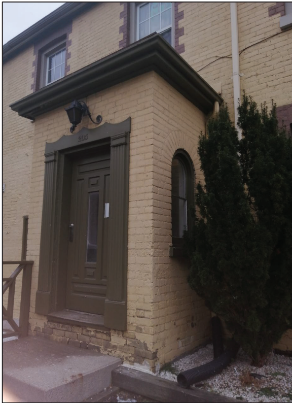
Figure 34: View of enclosed portico looking south-west (Source: MHBC, 2020).
