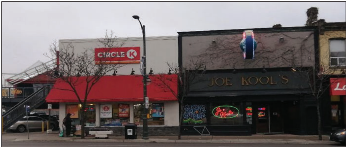
Figure 37: View of front façade of 595 Richmond Street including restaurant “Joe Kool’s” to the north and “Circle K” to the south; red box indicates location of access between 595 and 599 Richmond Street to rear ancillary brick structure (Source: MHBC, 2020).
