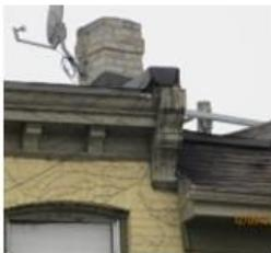
5. Cornice details including a) large corbels on each end of the cornice, and b) smaller band of corbels spanning the entirety of the east cornice.
