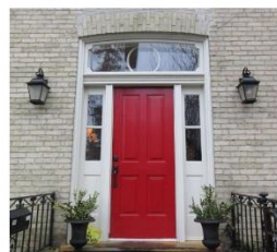
10. Front doorway with a pair of divided sidelights flanking a central door and a transom, with inset oculus
