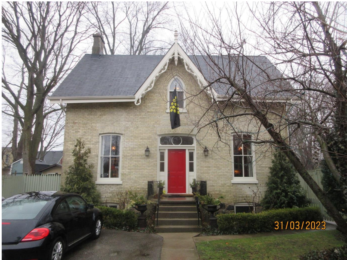
Photograph of the main elevation of the main block of the house.
