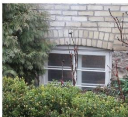
9. Basement window openings
