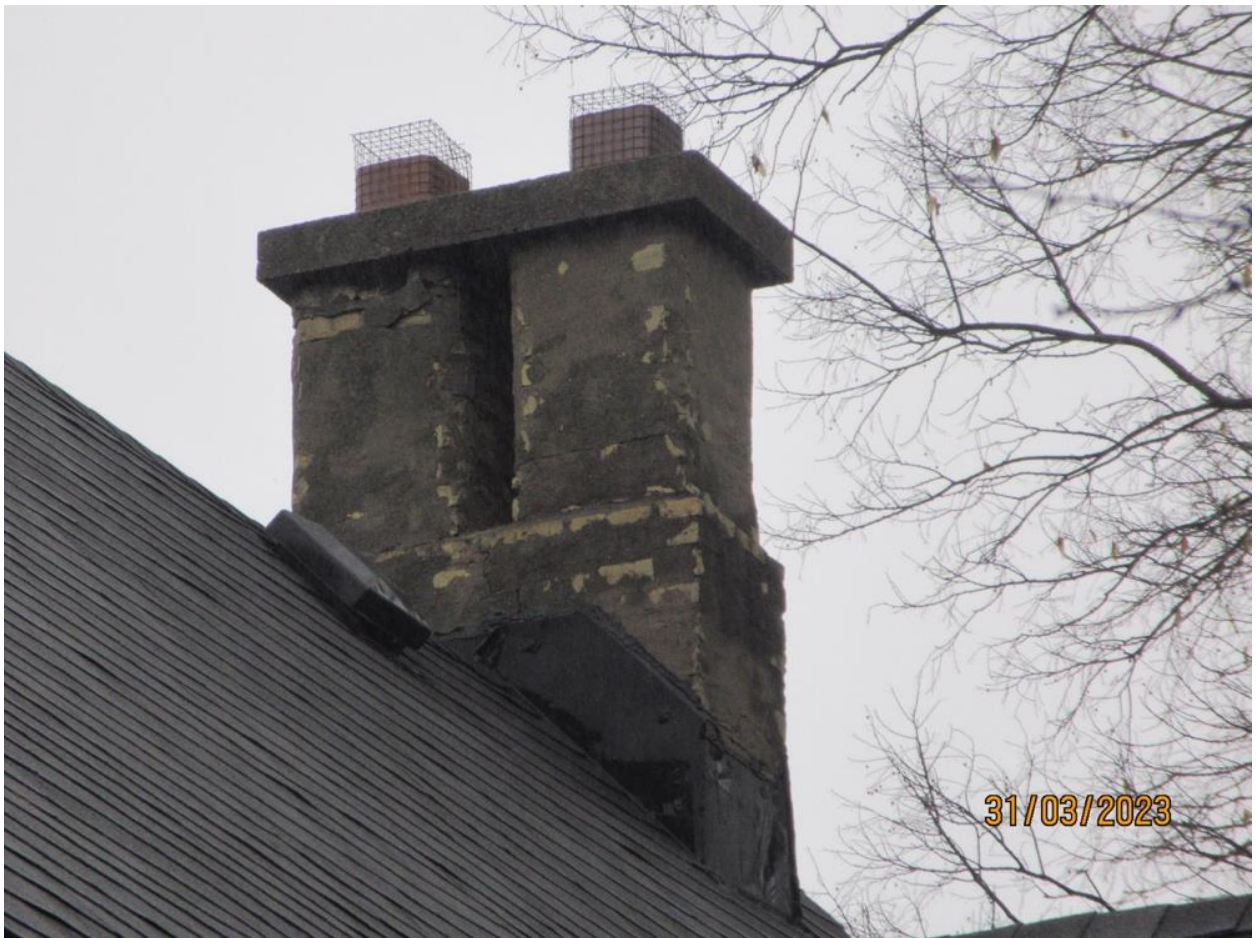
Image 8: Chimney on the north gable.
