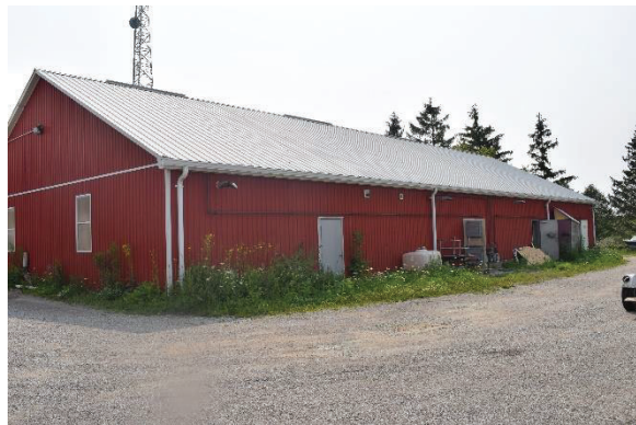
Plate 57: Outbuilding, west and north elevations, looking south
