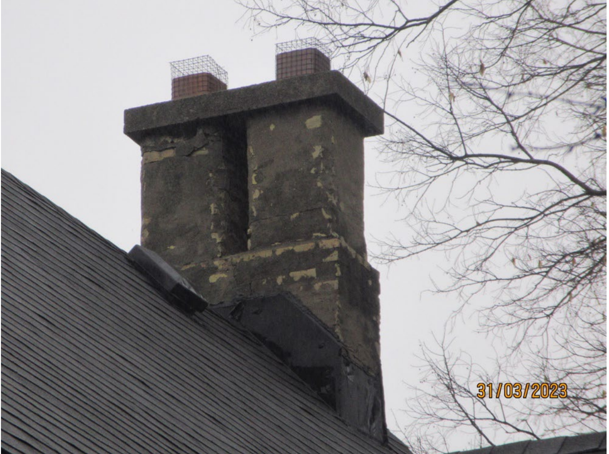
Image 8: Chimney on the north gable.
