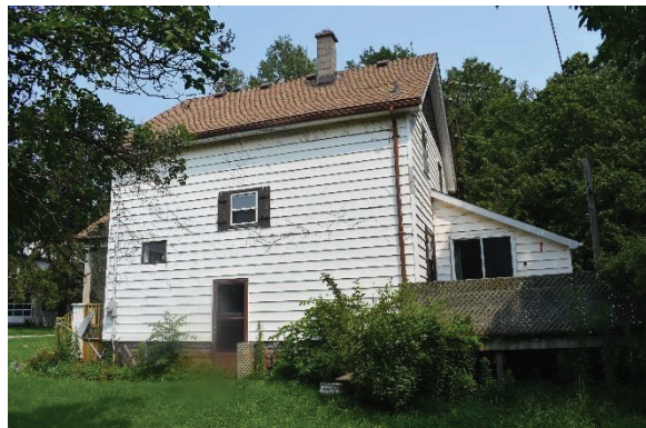
Plate 43: South elevation, looking north
