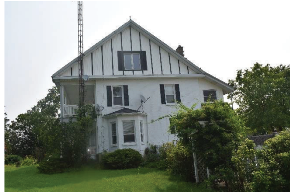
Plate 27: West elevation, looking east
