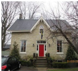
1. The form, scale, and massing of a one-and-one-a-half storey, buff brick dwelling with an unusually broad center cross gable
