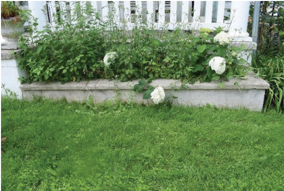
Plate 26: Concrete planter attached to porch, looking south
