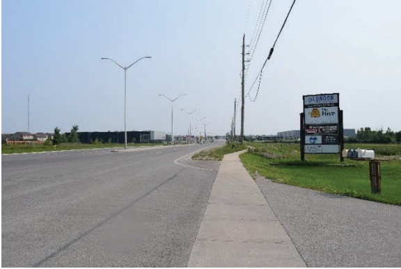
Plate 4: Looking northeast on Wharncliffe Road
