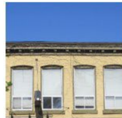
4. Symmetrical row of six arched window openings and stone sills on the second storey of the east façade.
