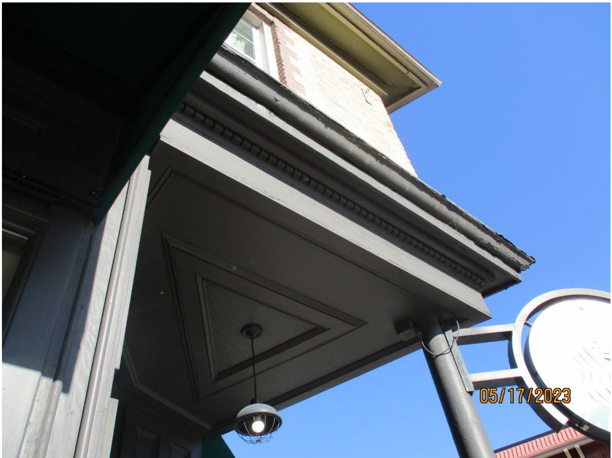
Image 12: Photograph showing the details of the recessed entryway to the building at 601 Richmond Street.
