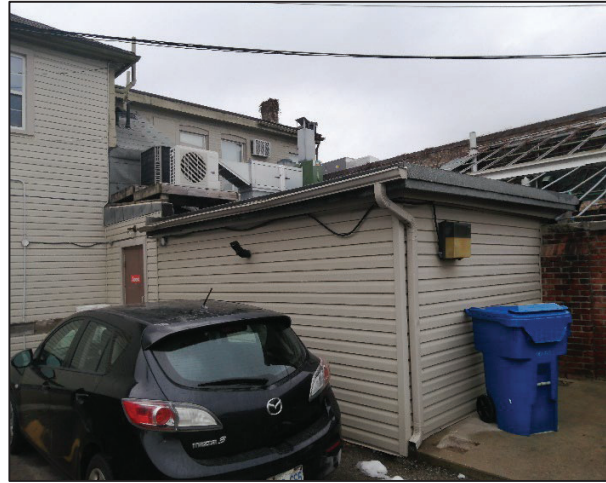
Figure 24: View of west elevation looking south-east (Source: MHBC, 2020).
