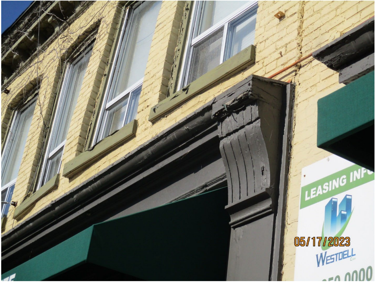
Image 3: Photograph showing corbel and cornice details above storefront on the building at 599 Richmond Street.
