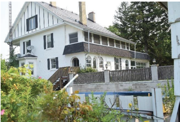
Plate 32: Looking northeast at shed roof addition
