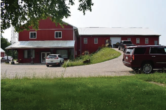
Plate 44: North elevation, looking south
