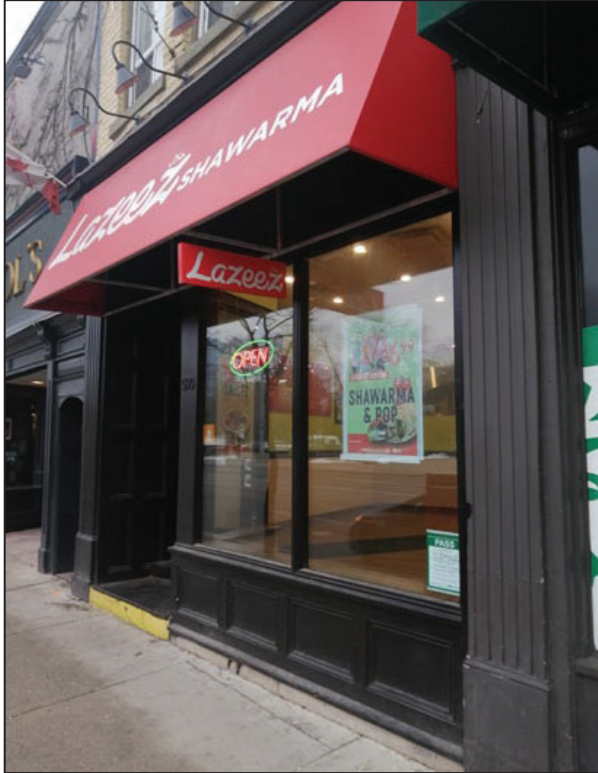
Figure 21: View of left side of front façade looking south-west.
