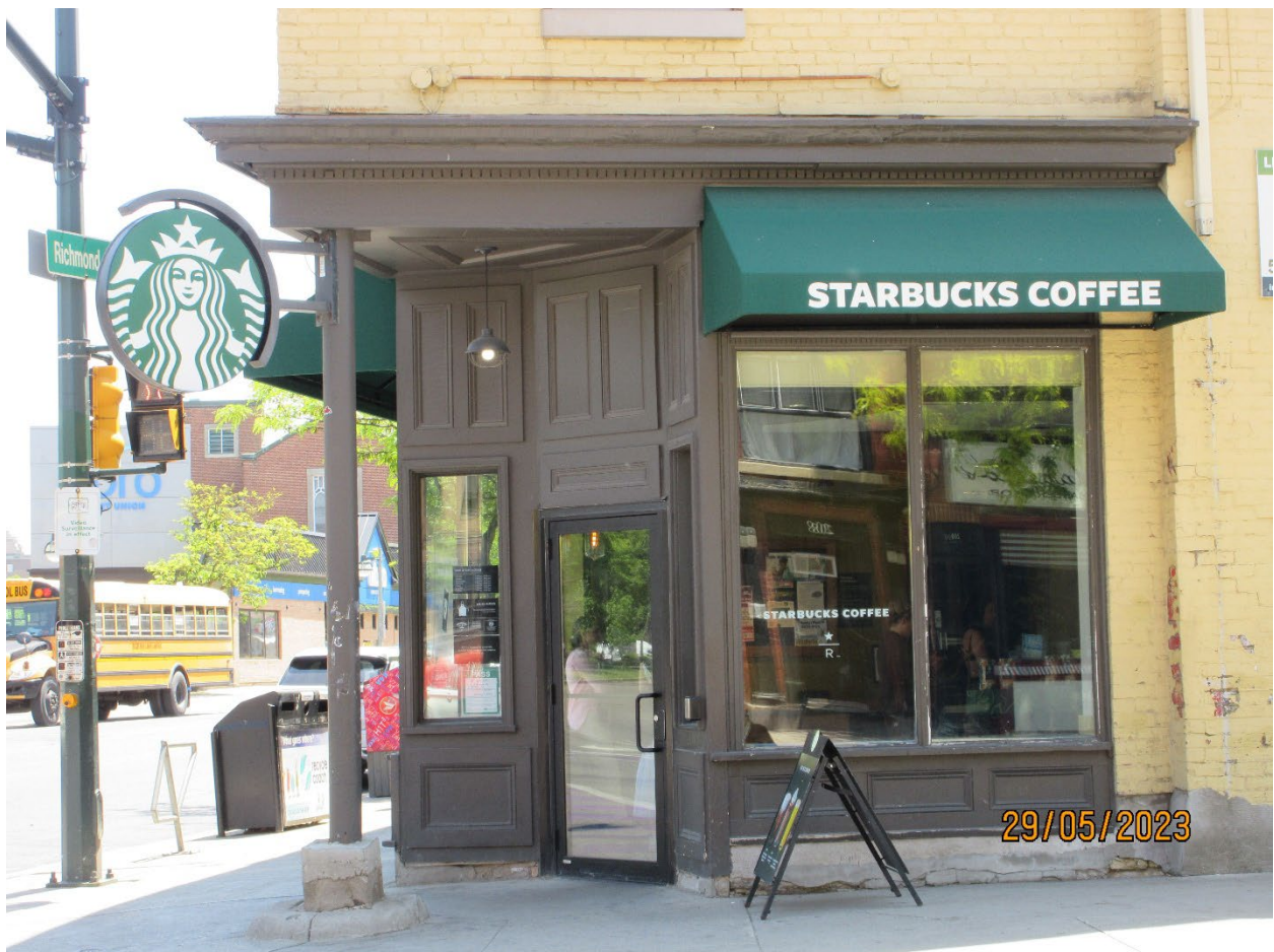
Image 14: Photograph showing recessed storefront entry way to the building at 601 Richmond Street.
