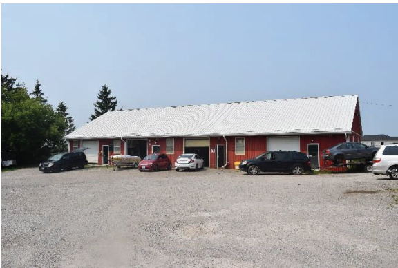
Plate 56: Outbuilding main elevation, looking west
