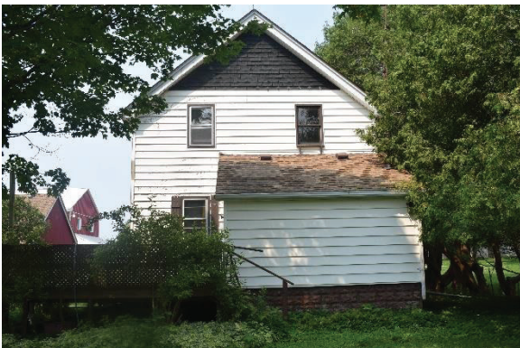
Plate 42: East elevation, looking west
