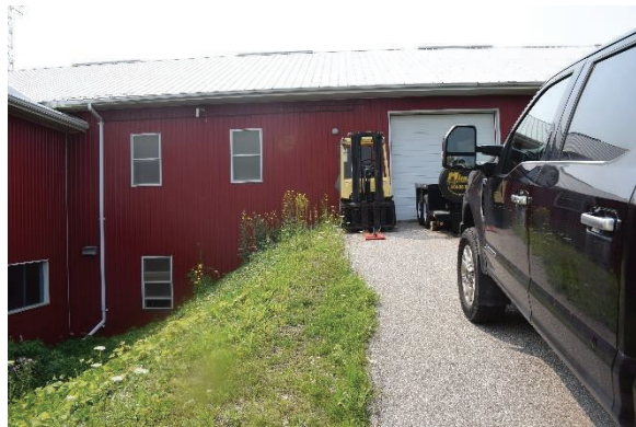
Plate 47: First storey window on south north elevation east-west section, looking south
