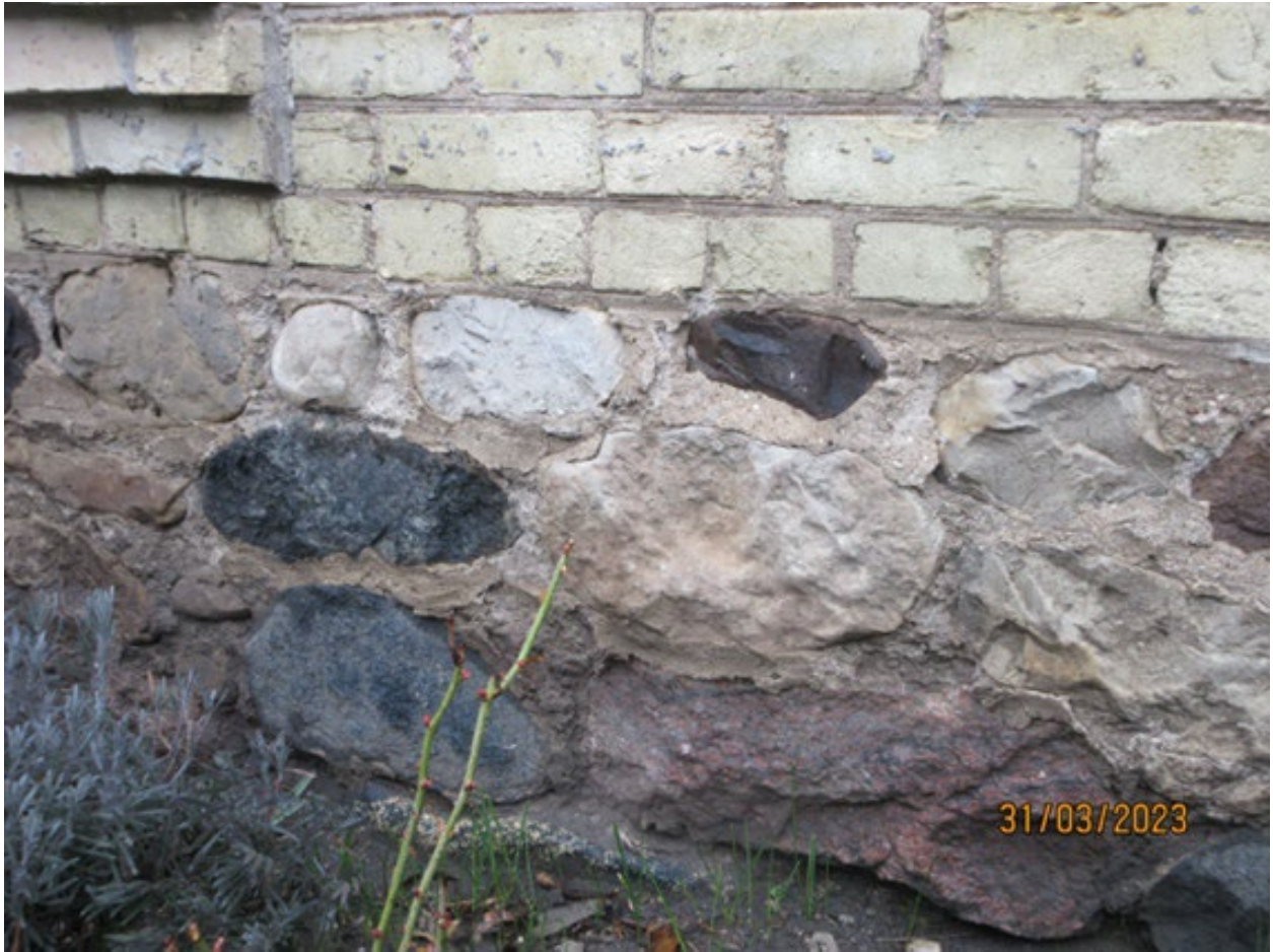
Image 9: Fieldstone foundation wall on the west elevation.
