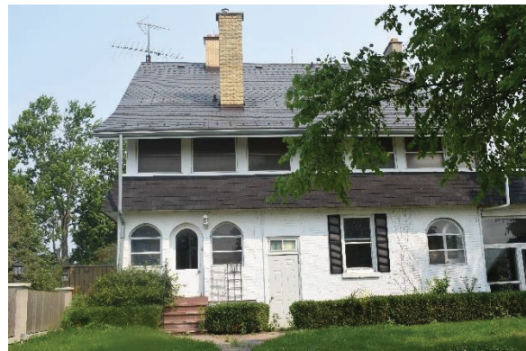
Plate 33: South elevation, looking north
