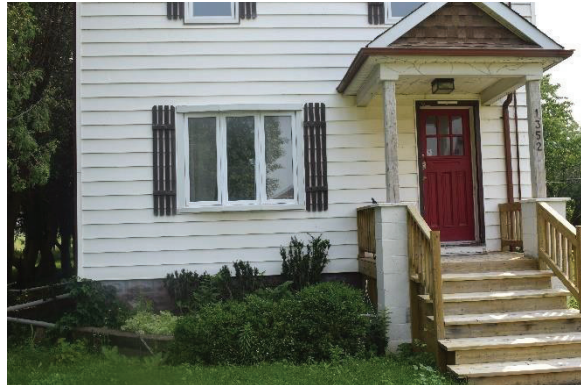
Plate 39: First storey of west elevation, looking east
