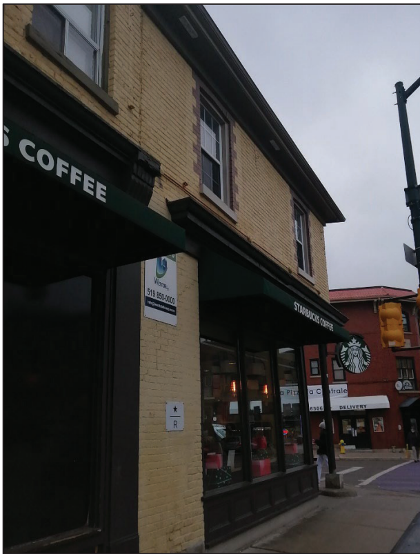
Figure 29: View of front façade looking northwest (Source: MHBC, 2020).
