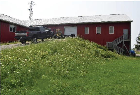
Plate 46: Looking south at bank and second storey
