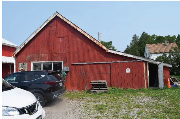
Plate 55: South elevation, looking north
