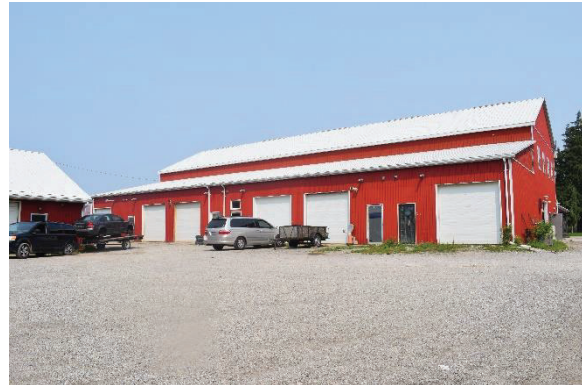
Plate 51: South elevation, looking north
