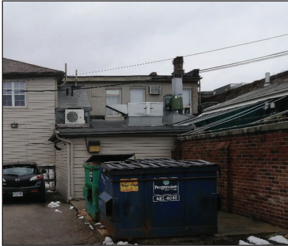
Figure 23: View of west elevation (Source: MHBC, 2020).
