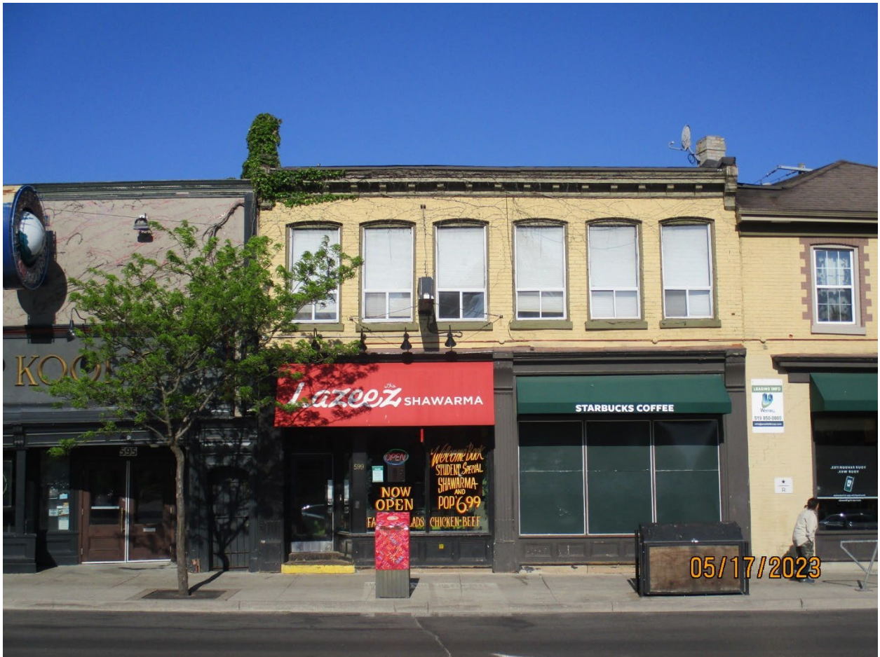
Image 1: Photograph showing the building on the subject property at 599 Richmond Street.
