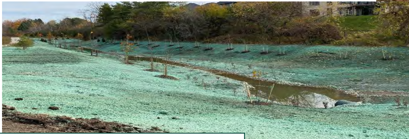
Powell Drain Reconstruction (2020)
