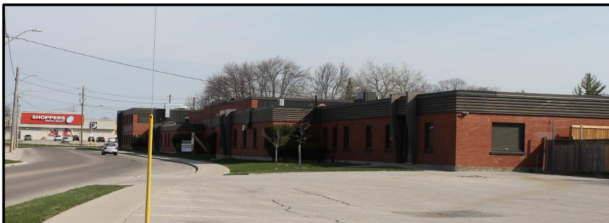
Figure 1: 340-390 Saskatoon Street (East Side) Looking North to Whitney Street
