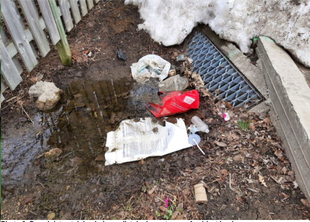
Photo 2. Drop-inlet catch basin immediately downstream of subject lands.
