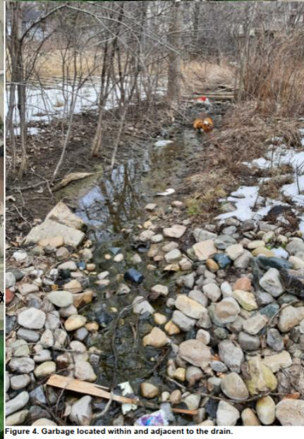
Figure 4. Garbage located within and adjacent to the drain.
