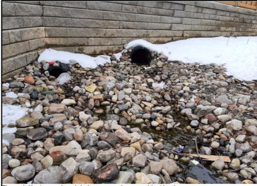
Figure 1. Upstream closed drains converging on subject lands.
