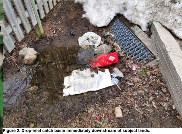
Figure 2. Drop-inlet catch basin immediately downstream of subject lands.
