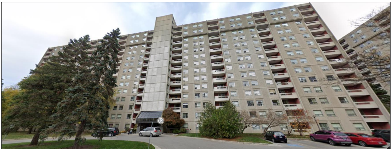
Figure 1: Image of 595 Proudfoot Lane, facing north (Google Image, October 2020)
