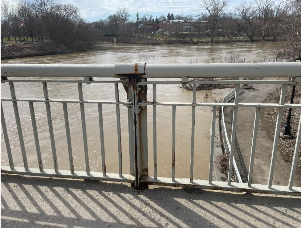
Photograph 14: Handrailing system (AECOM, April 2023)
