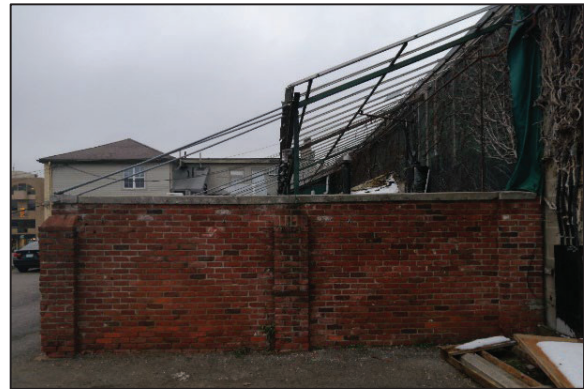
Figure 26: View of west elevation (Source: MHBC, 2020).
