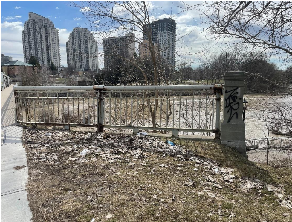
Photograph 9: Southwest concrete post and handrailing (AECOM, April 2023)
