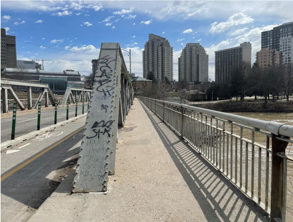
Photograph 6: Sidewalk portal view on south side, looking east (AECOM, April 2023)
