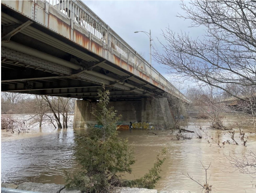
Photograph 24: Oblique view of bridge from the northeast quadrant (AECOM, April 2023)
