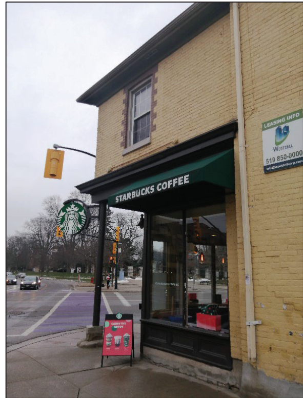
Figure 32: View of front façade looking south, (right) View of entrance at corner of the intersection looking south-east (Source: MHBC, 2020).
