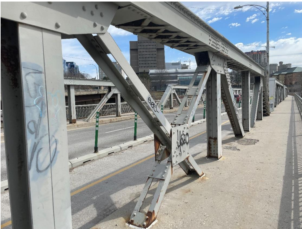
Photograph 15: Intermediate connection viewed from the south sidewalk (AECOM, April 2023)
