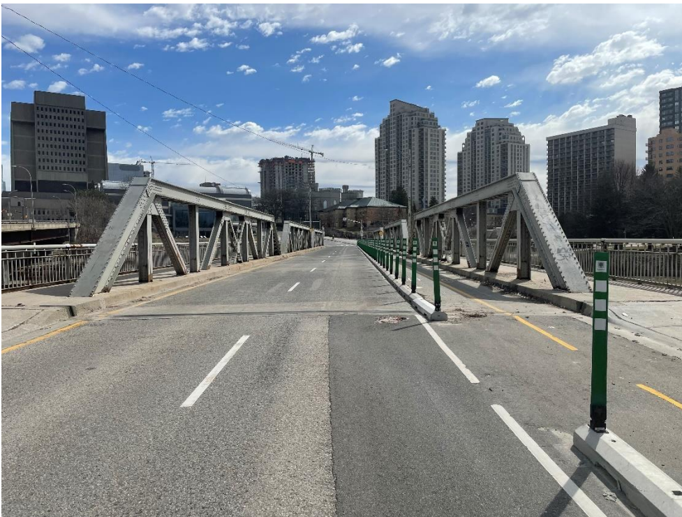
Photograph 3:West end portal view (AECOM, April 2023)
