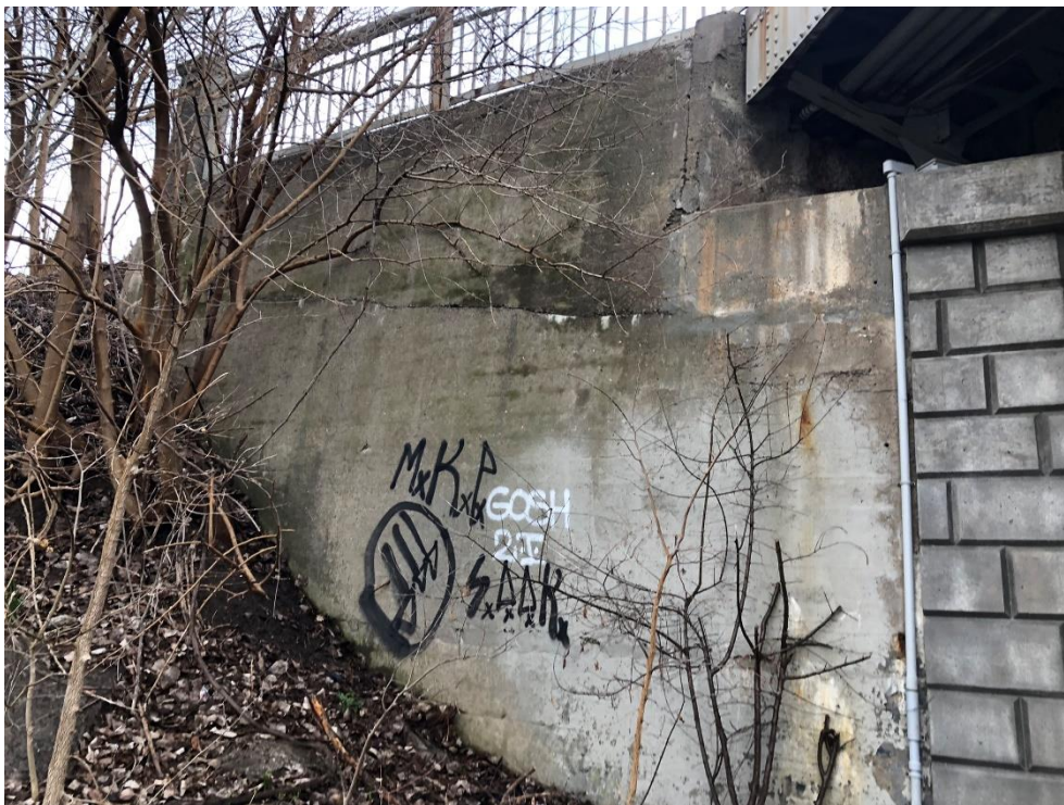
Photograph 29: Southwest wingwall (AECOM, 2022)
