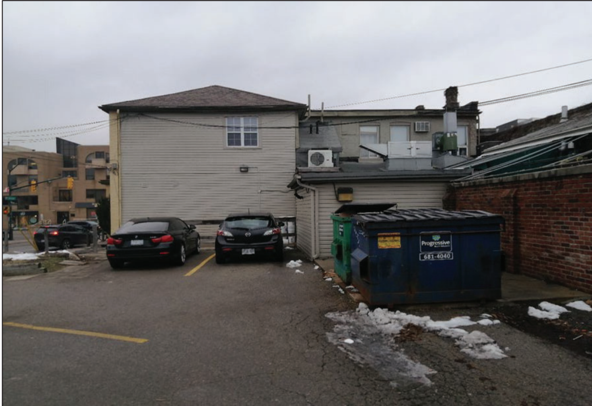
Figure 36: View of west elevation (Source: MHBC, 2020).
