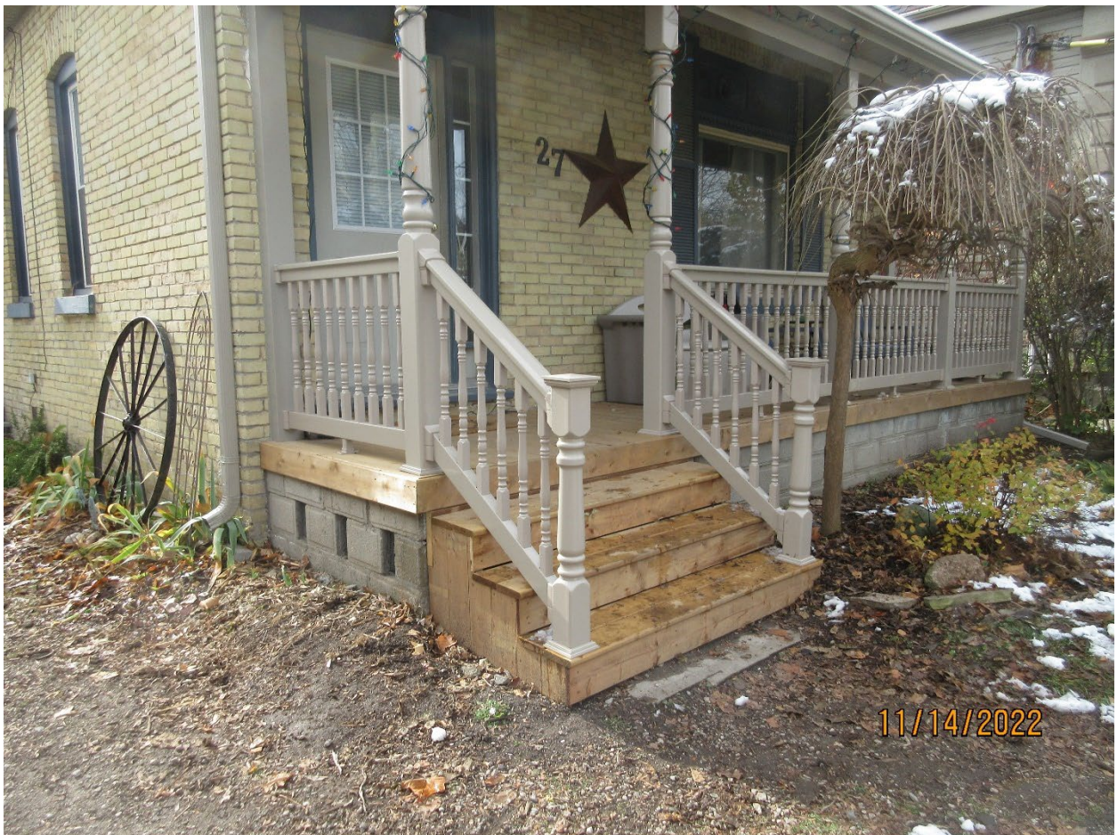
Image 4: Photograph showing detail of the vinyl (plastic) porch materials used for the replacement of the porch at 27 Bruce Street within the Wortley Village-Old South Heritage Conservation District.
