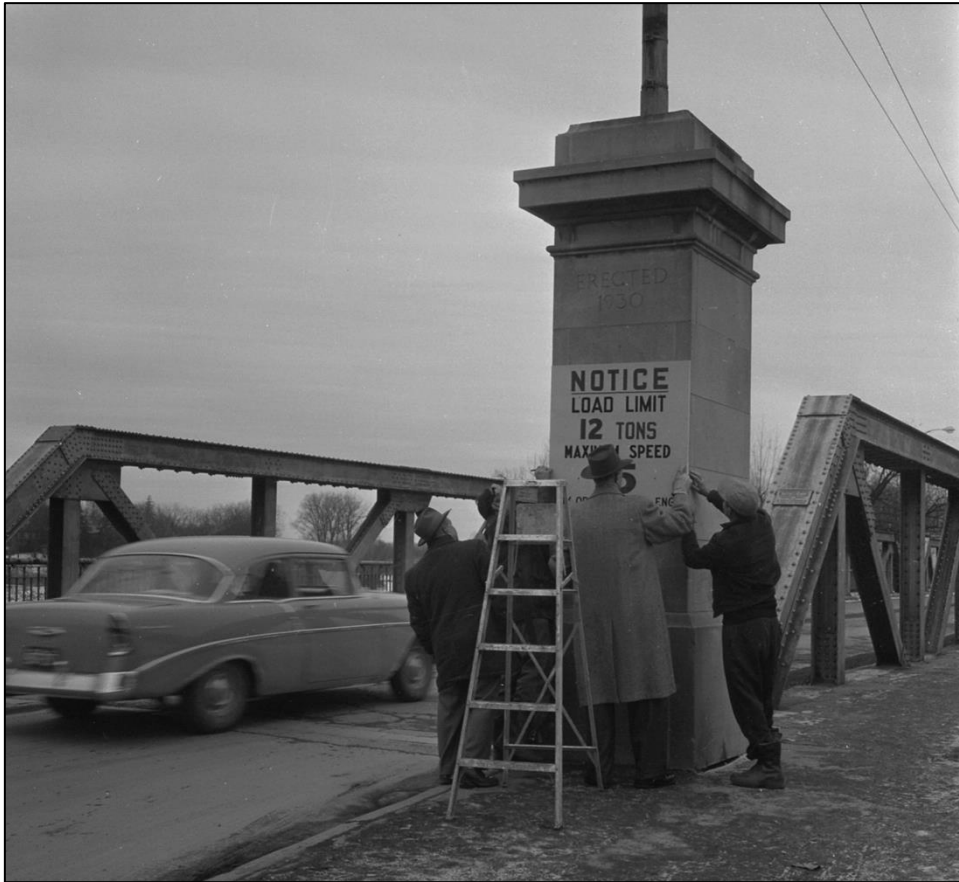
Image 5: Pillar with load limit and a date stone “Erected 1930” (Western University, London Free Press, January 9, 1960)
