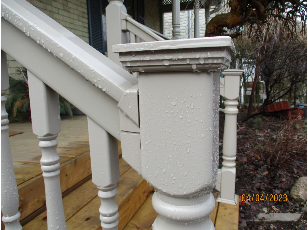
Image 6: Photograph showing detail of the vinyl (plastic) porch materials used for the replacement of the porch at 27 Bruce Street within the Wortley Village-Old South Heritage Conservation District.
