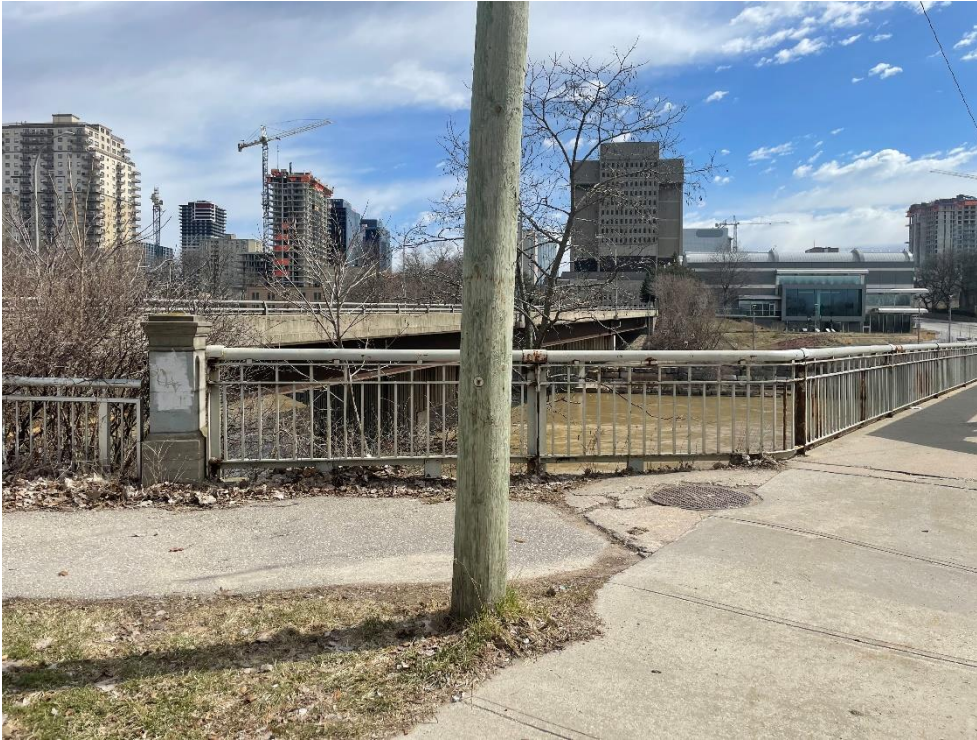
Photograph 10: Northwest concrete post and handrailing (AECOM April 2023)
