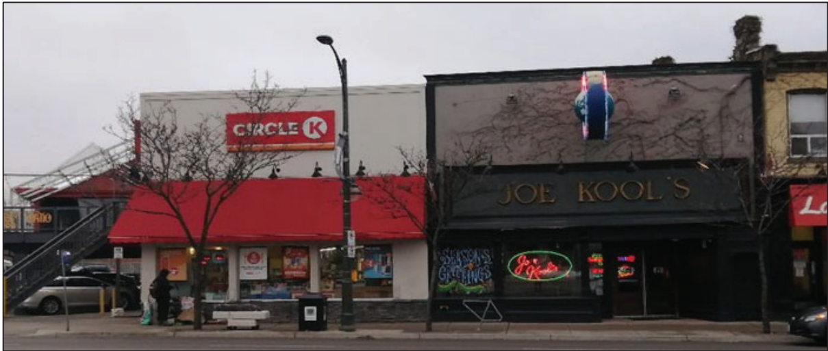
Figure 37: View of front façade of 595 Richmond Street including restaurant “Joe Kool’s” to the north and “Circle K” to the south; red box indicates location of access between 595 and 599 Richmond Street to rear ancillary brick structure (Source: MHBC, 2020).
