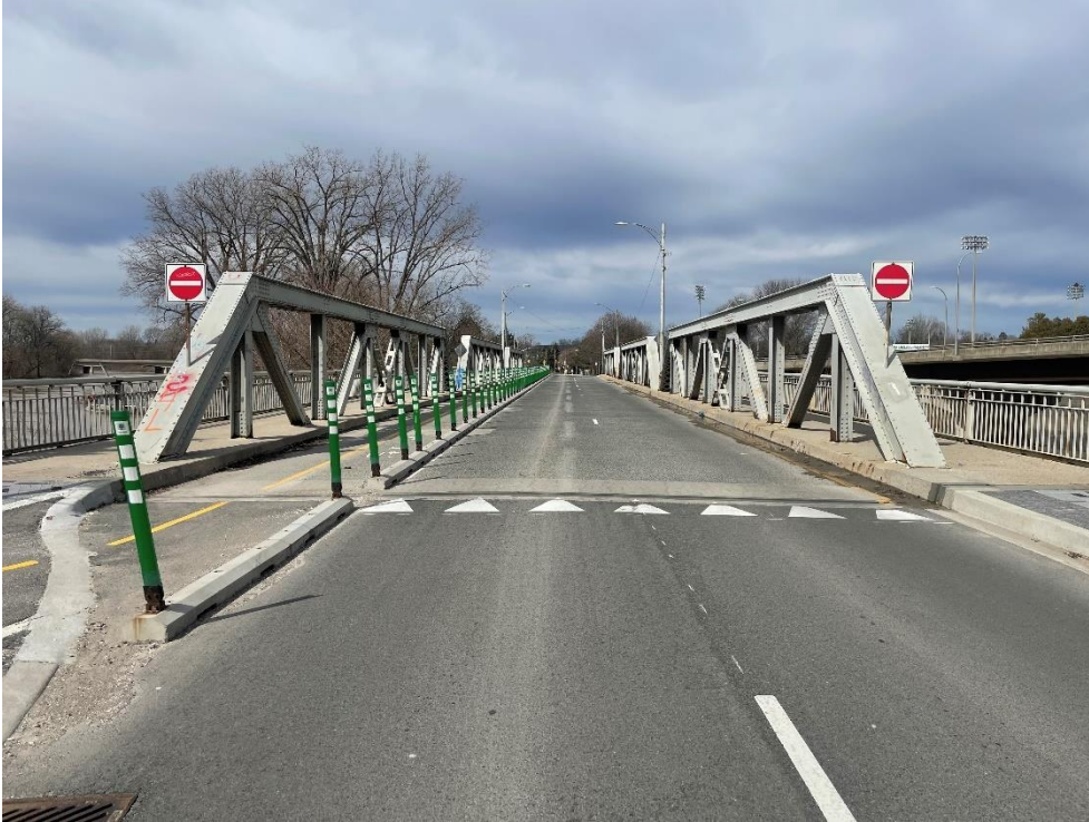
Photograph 4: East end portal view (AECOM, April 2023)
