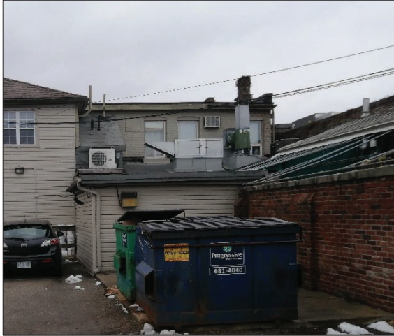
Figure 23: View of west elevation (Source: MHBC, 2020).
