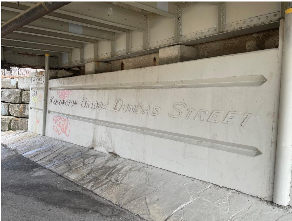
Photograph 21: Close-up of the east abutment (AECOM, 2021)
