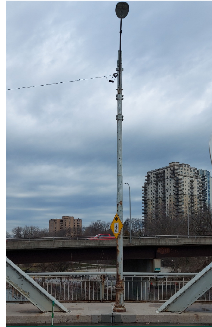
Kensington Bridge Existing Light Standard
