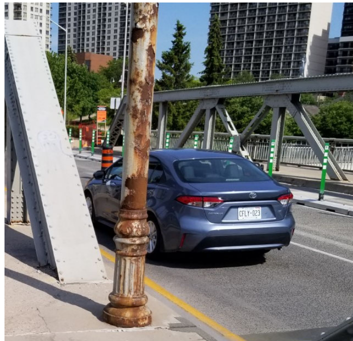
Kensington Bridge Existing Light Standard Base
