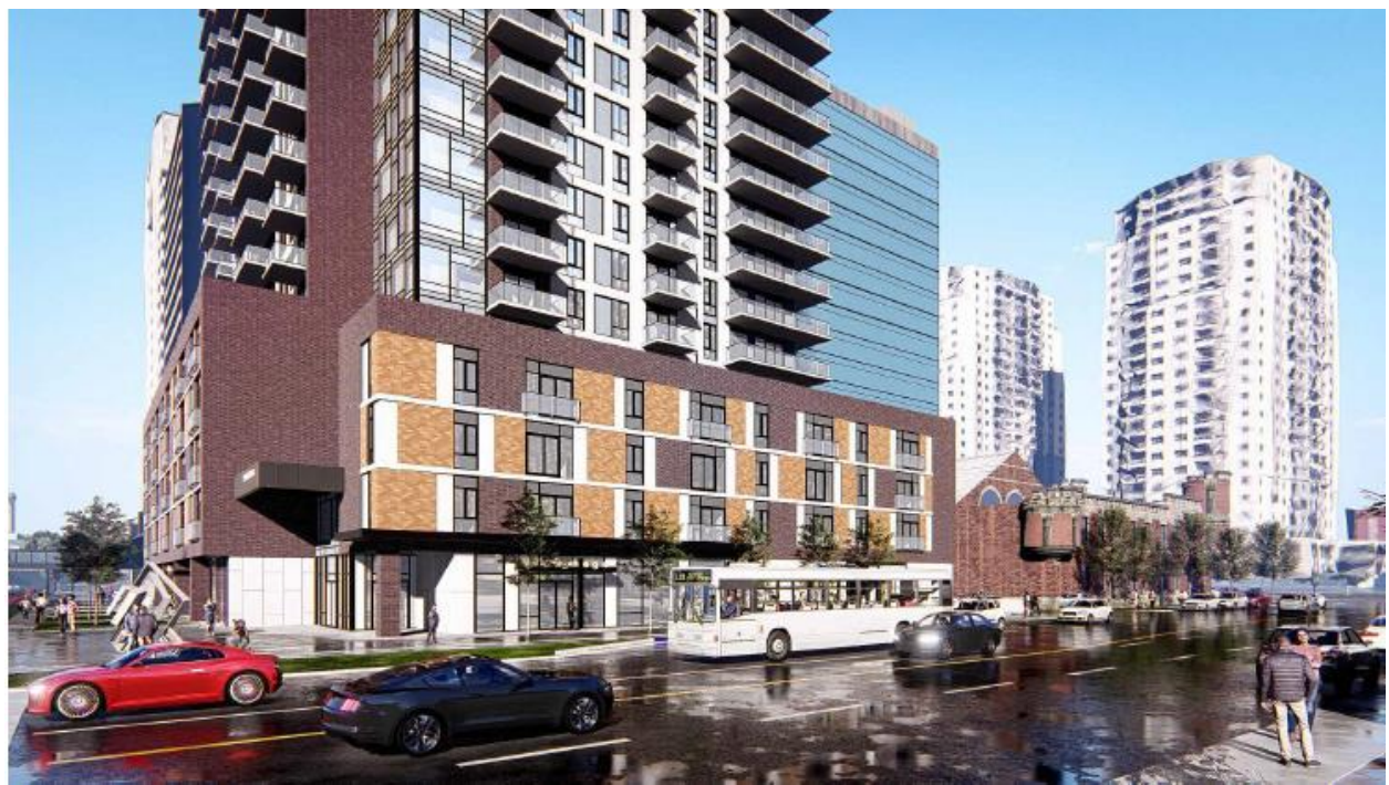
Figure 8: Tower base (corner view from Waterloo Street)
