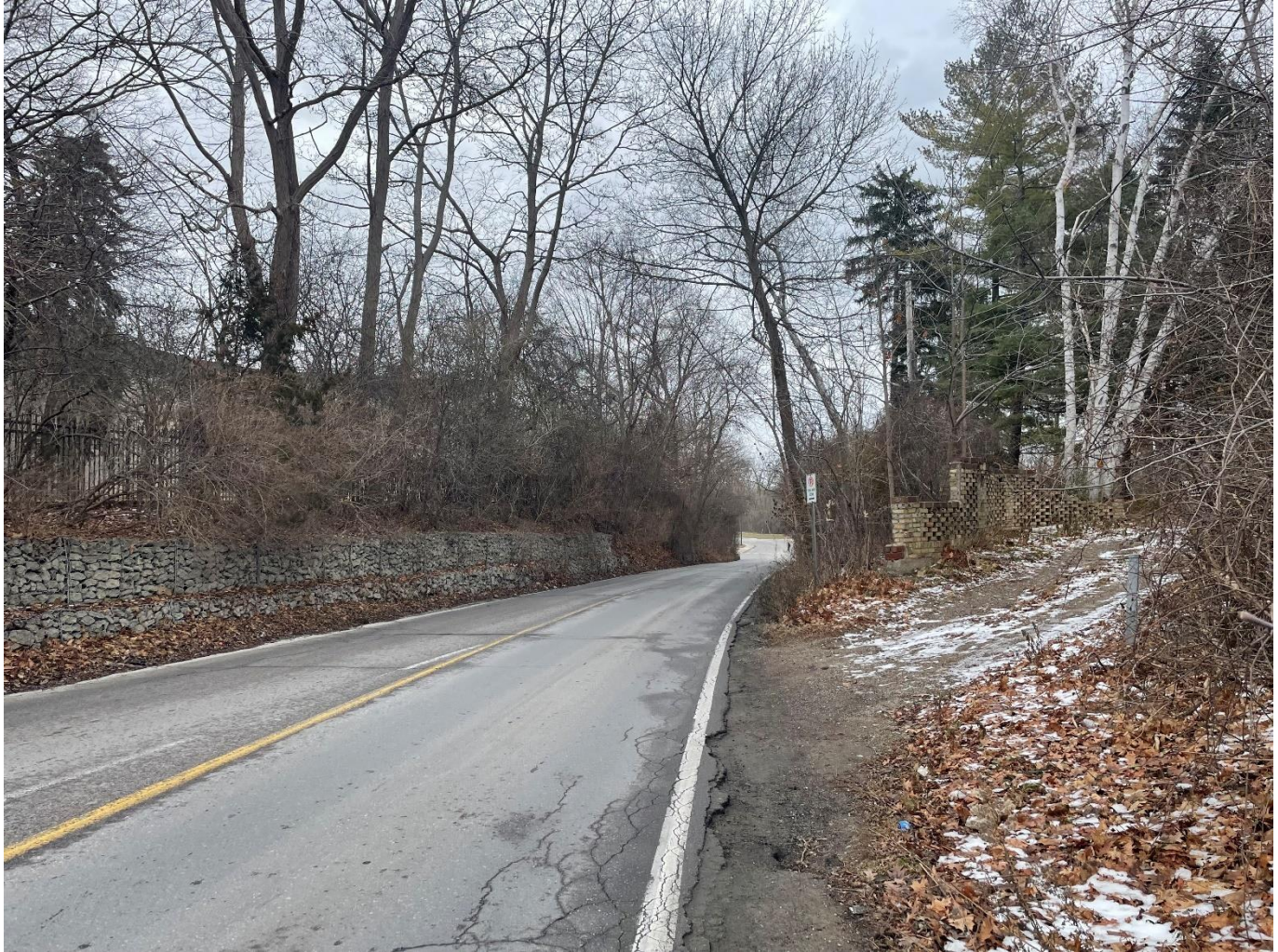
Photograph 1: A view of Philip Aziz Avenue, looking east
