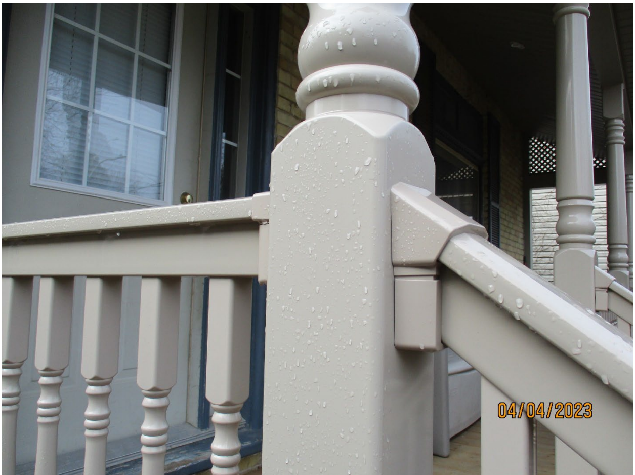
Image 8: Photograph showing detail of the vinyl (plastic) porch materials used for the replacement of the porch at 27 Bruce Street within the Wortley Village-Old South Heritage Conservation District.
