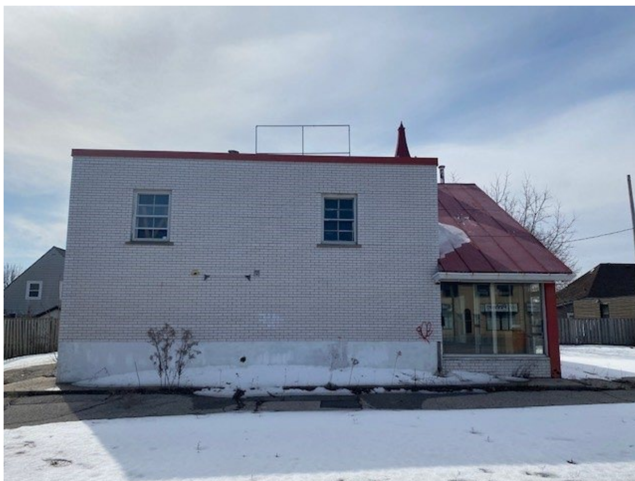
689 Hamilton Road – East side
