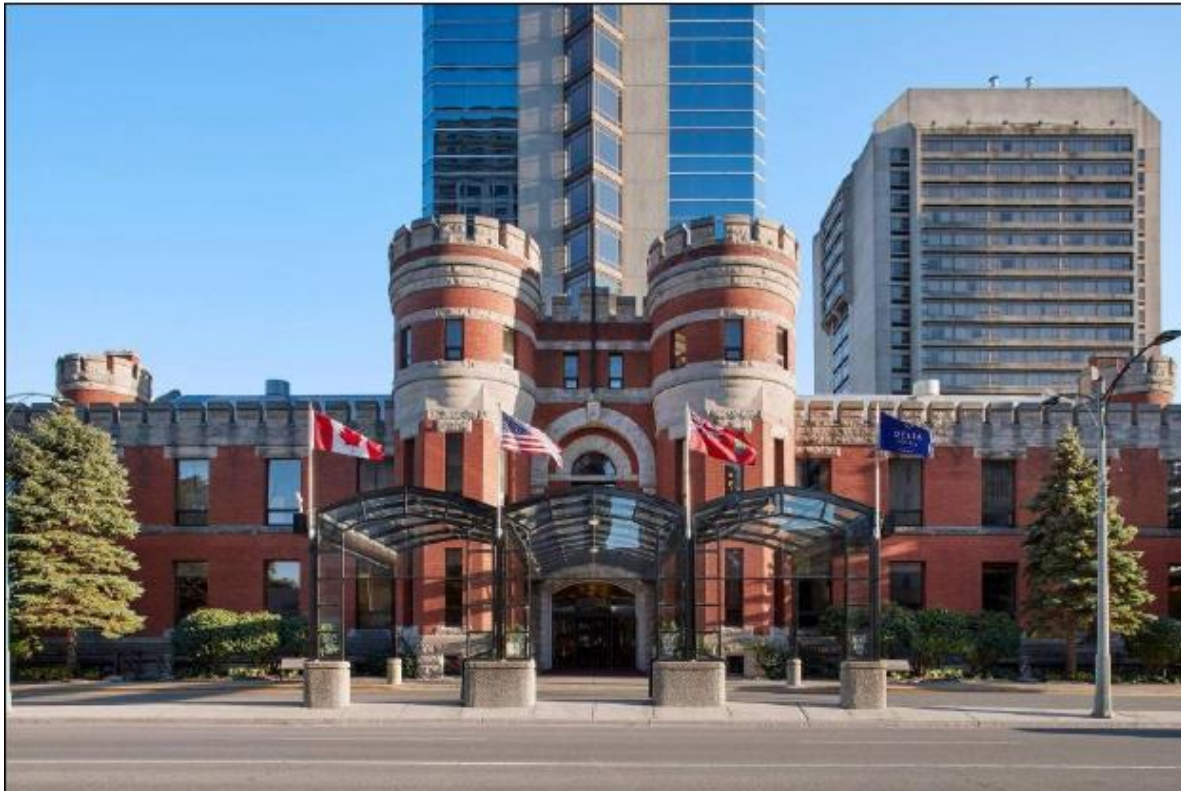
Figure 13 – Photo of the existing heritage building – The Delta Armouries Hotel
