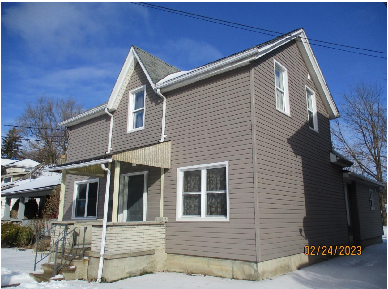
Image 4: Photograph of the subject property at 19 Blackfriars Street, within the Blackfriars/Petersville Heritage Conservation District after the dwelling had been re-clad with vinyl siding (2023).
