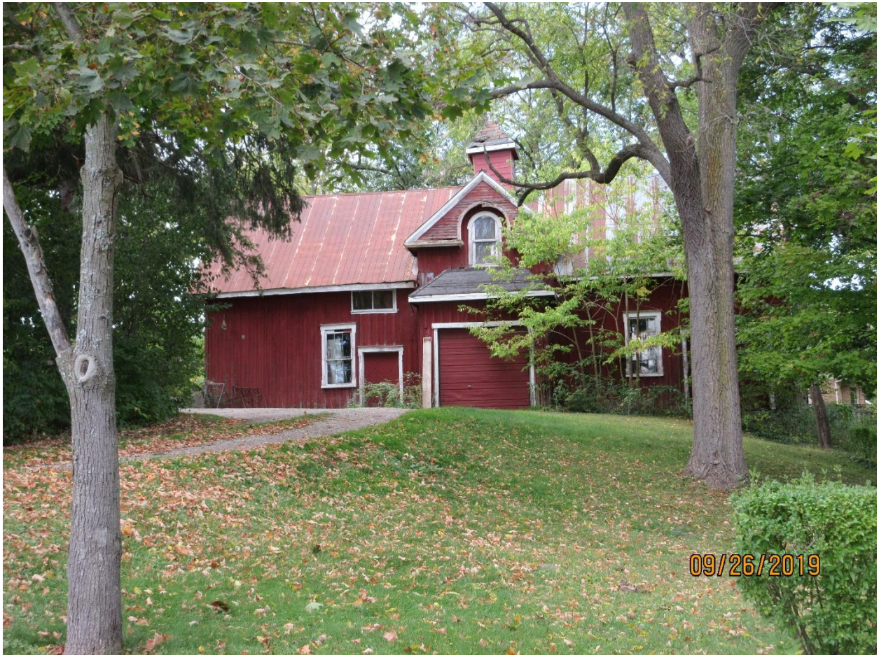
Image 1: Photograph showing the accessory building in September 2019.
