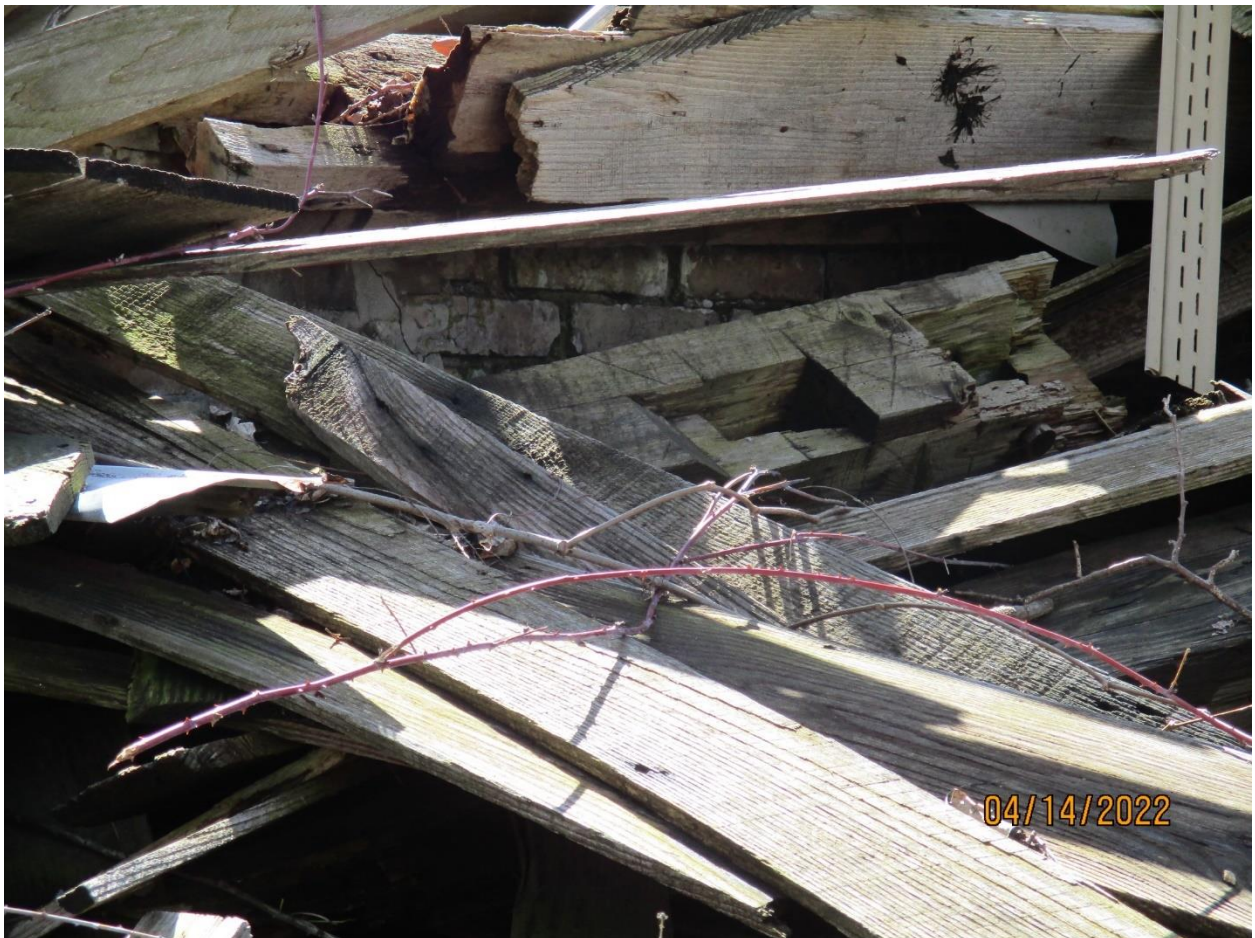
Image 12: Photograph showing debris from the former accessory building, shown in April 2022. Note, a portion of the buff brick foundation can be seen buried under the debris.
