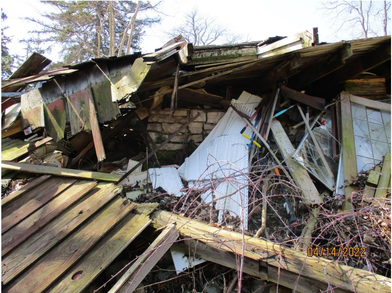
Image 13: Photograph showing debris from the former accessory building, shown in April 2022. Note, a portion of the rubble stone foundation can be seen buried under the debris.
