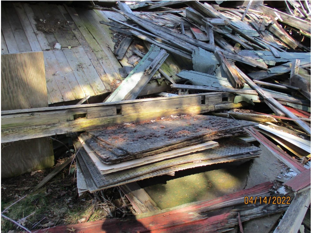
Image 15: Photograph showing debris from the former accessory building, shown in April 2022.
