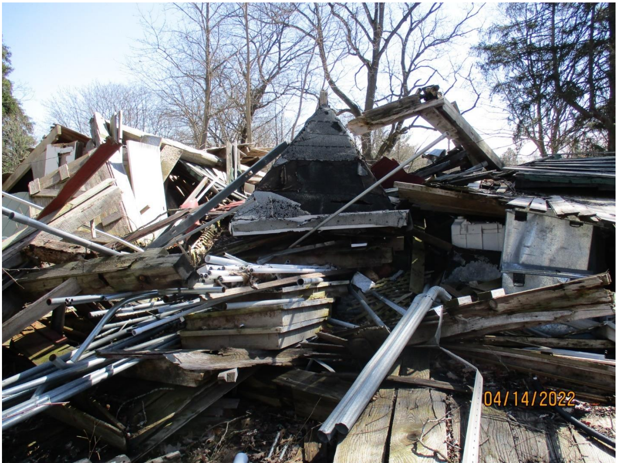
Image 16: Photograph showing debris from the former accessory building, shown in April 2022.
