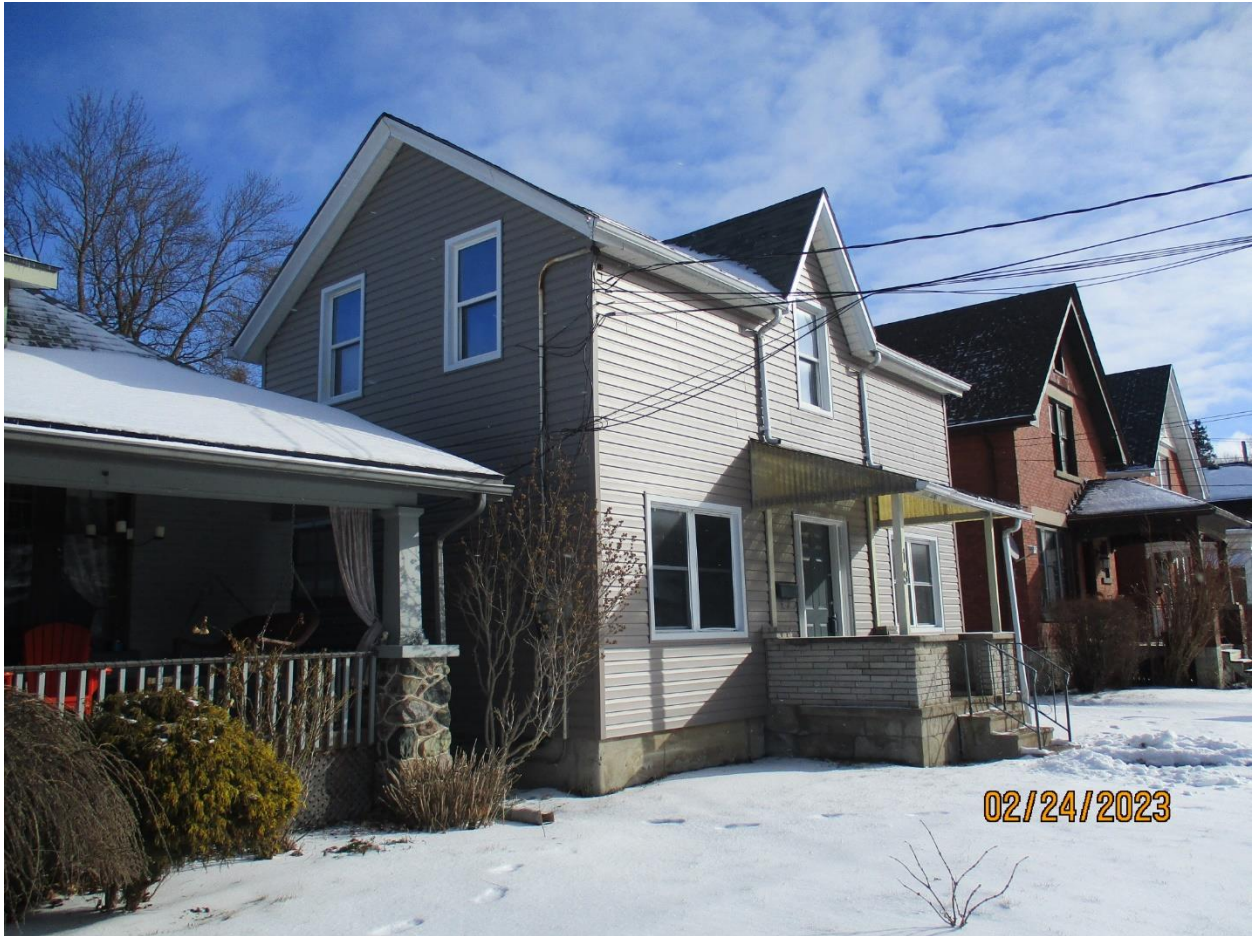
Image 3: Photograph of the subject property at 19 Blackfriars Street, within the Blackfriars/Petersville Heritage Conservation District after the dwelling had been re-clad with vinyl siding (2023).
