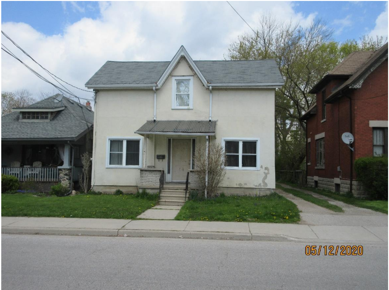
Image 1: Photograph of the subject property at 19 Blackfriars Street, within the Blackfriars/Petersville Heritage Conservation District prior to the installation of the new vinyl siding (2020).
