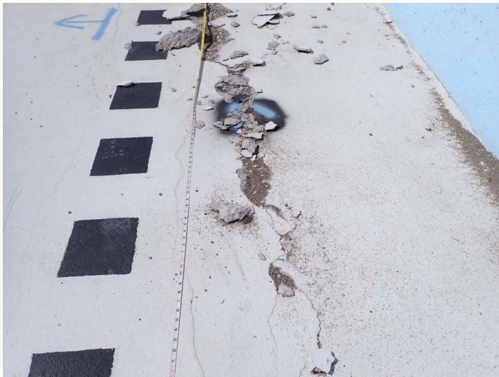
Photo 7 – Subgrade Deterioration
