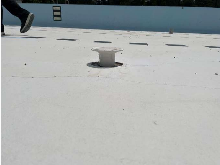
Photo 4 – Spalling of concrete along the crack line evident in the pool slab
