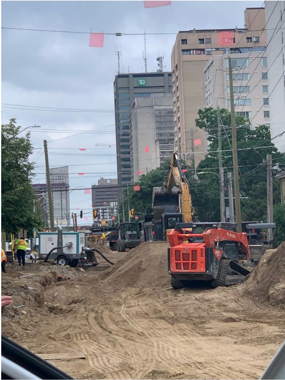
Above: East London Link Phase 1 construction site at King Street.
