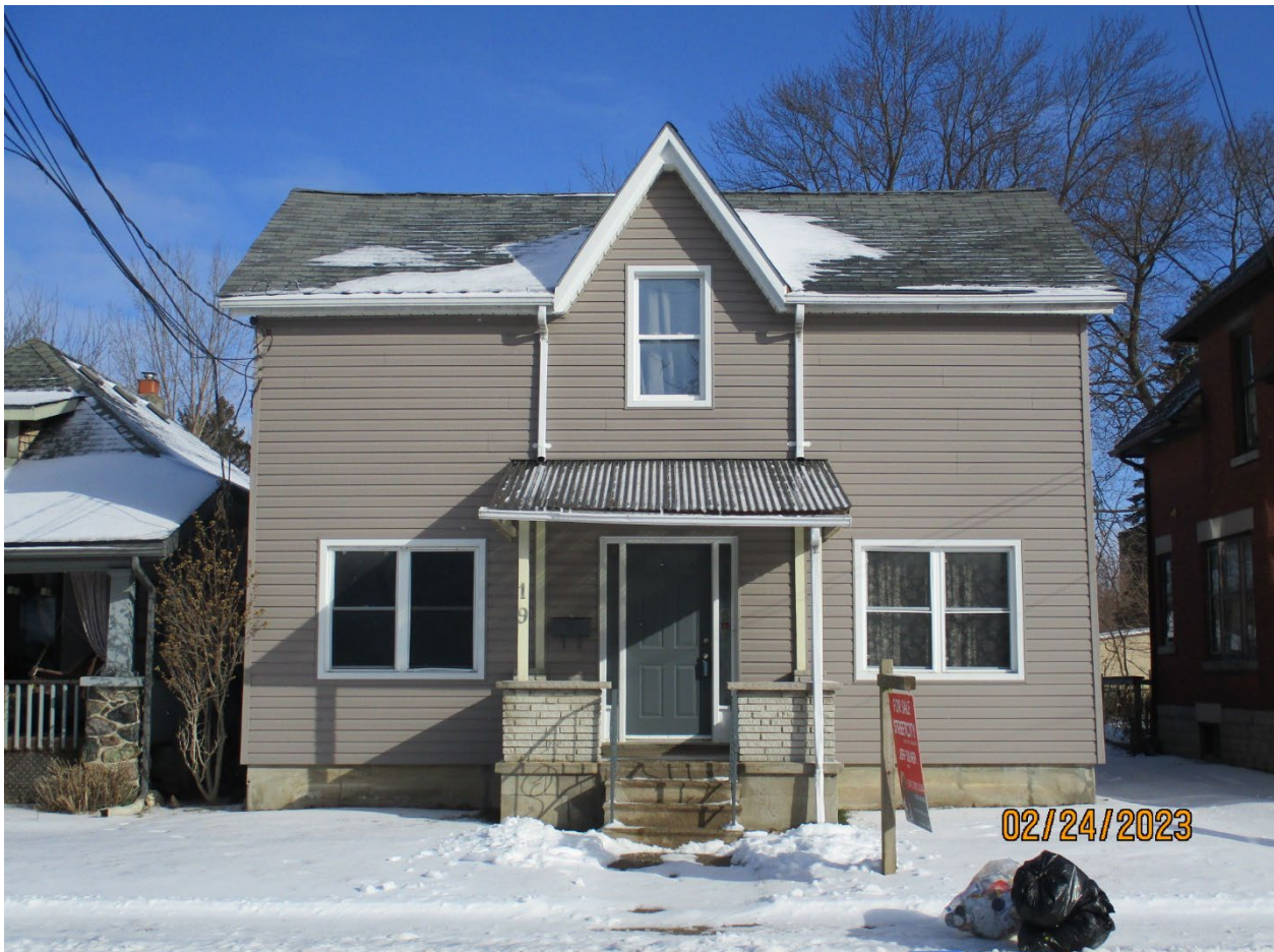
Image 2: Photograph of the subject property at 19 Blackfriars Street, within the Blackfriars/Petersville Heritage Conservation District after the dwelling had been re-clad with vinyl siding (2023).
