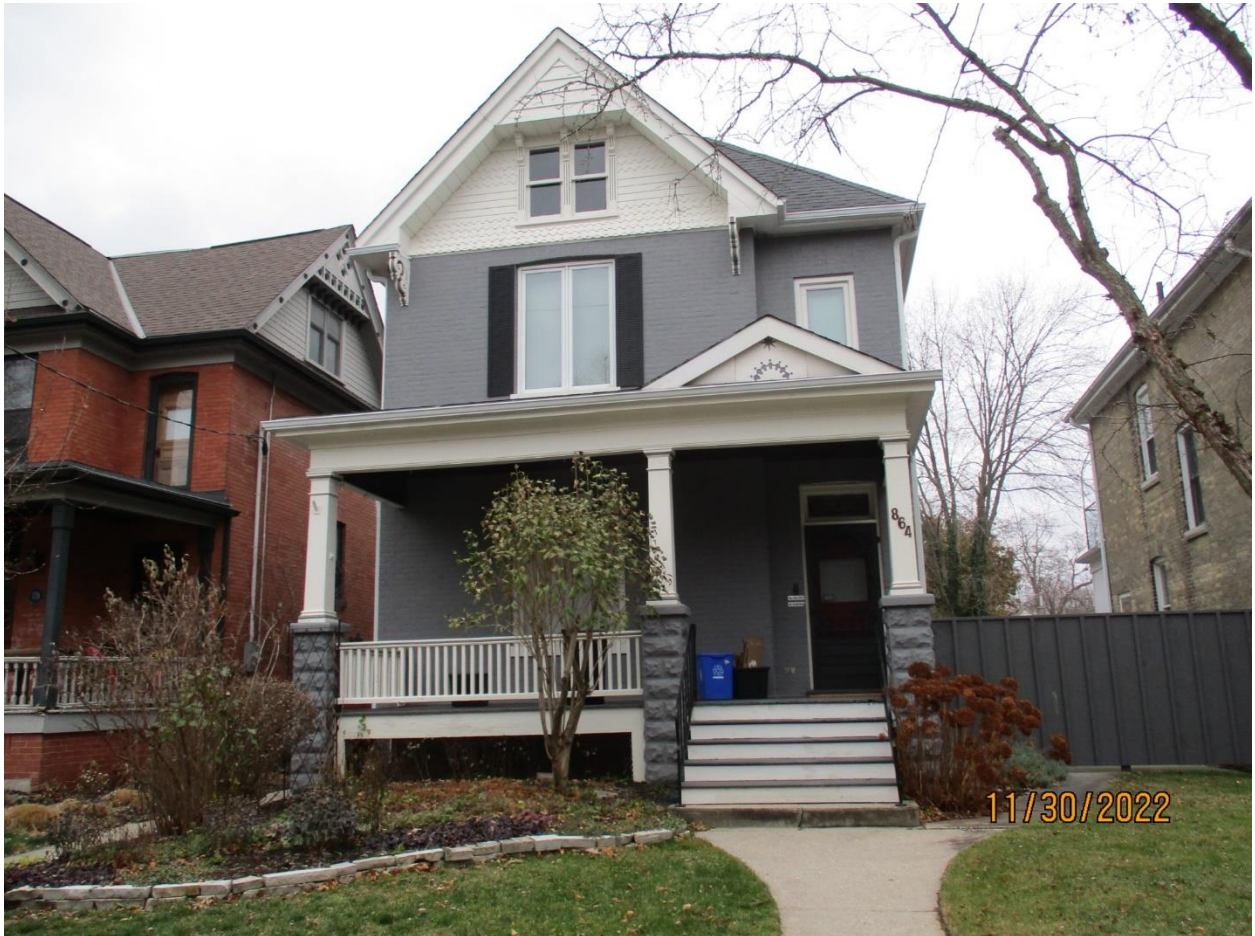
Image 1: Photograph showing the dwelling located at 864 Hellmuth Avenue.
