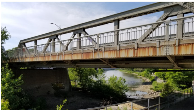
Kensington Bridge – South Elevation
