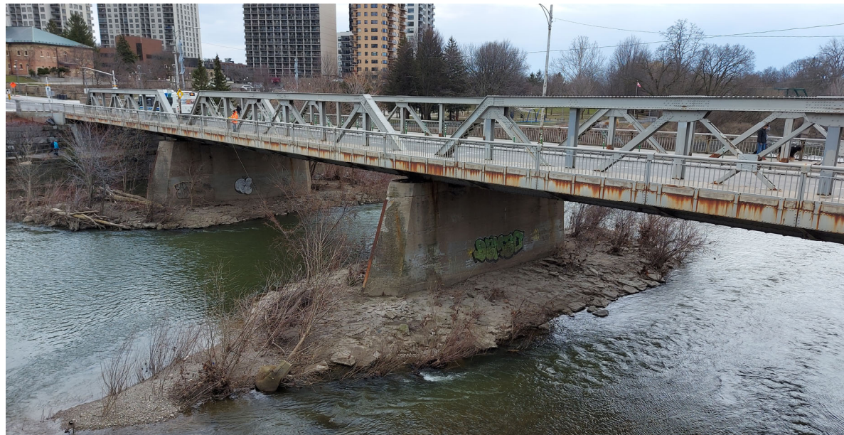
Kensington Bridge – North Elevation
