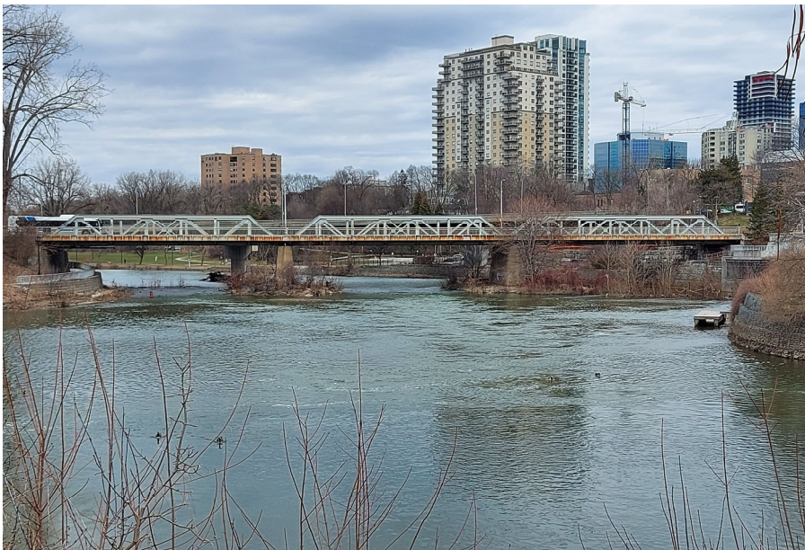
Kensington Bridge – South Elevation
