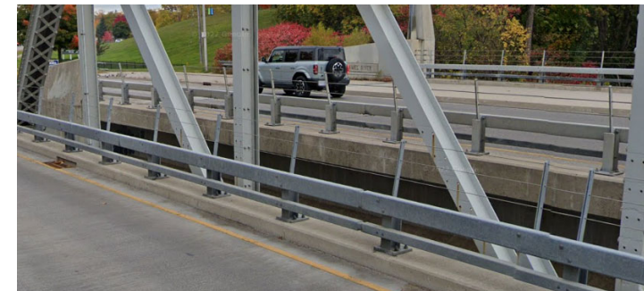
West Brough's Bridge – Example of two tube system
