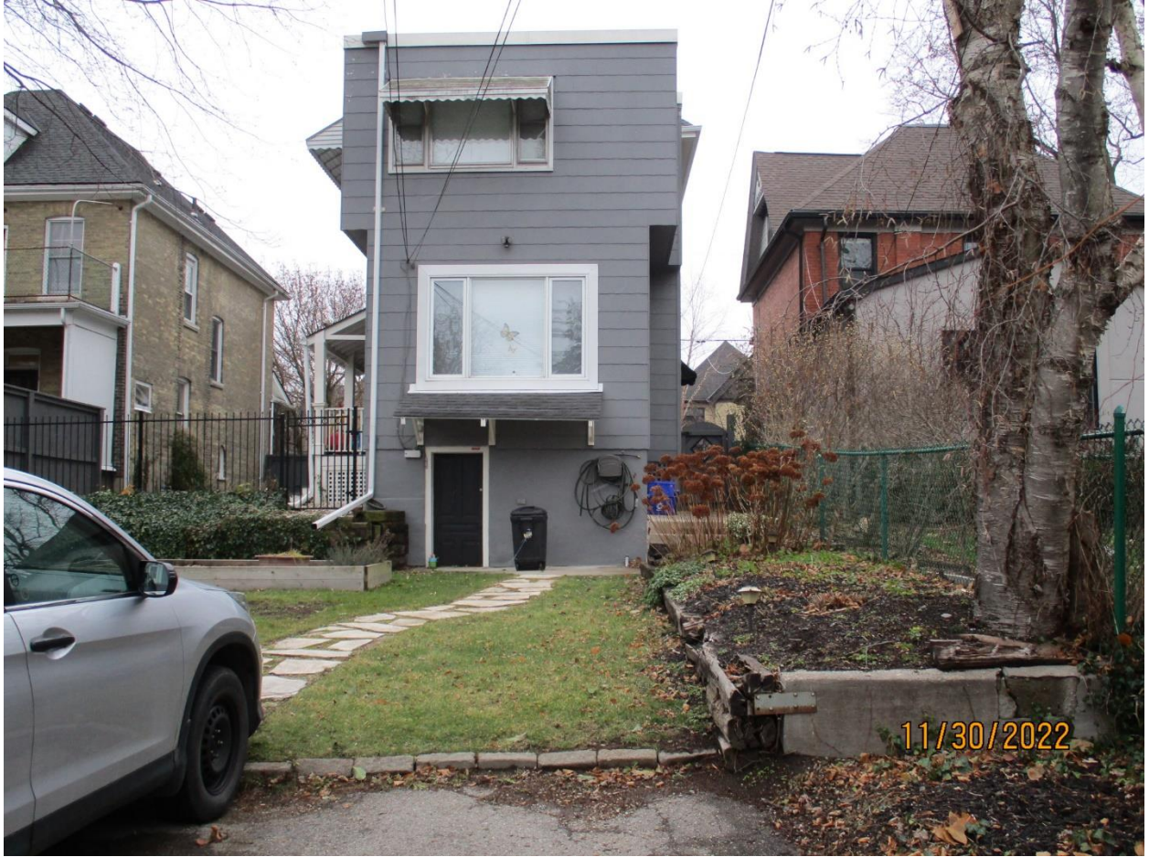
Image 6: Photograph showing at grade entry to the rear of the property at 864 Hellmuth Avenue.
