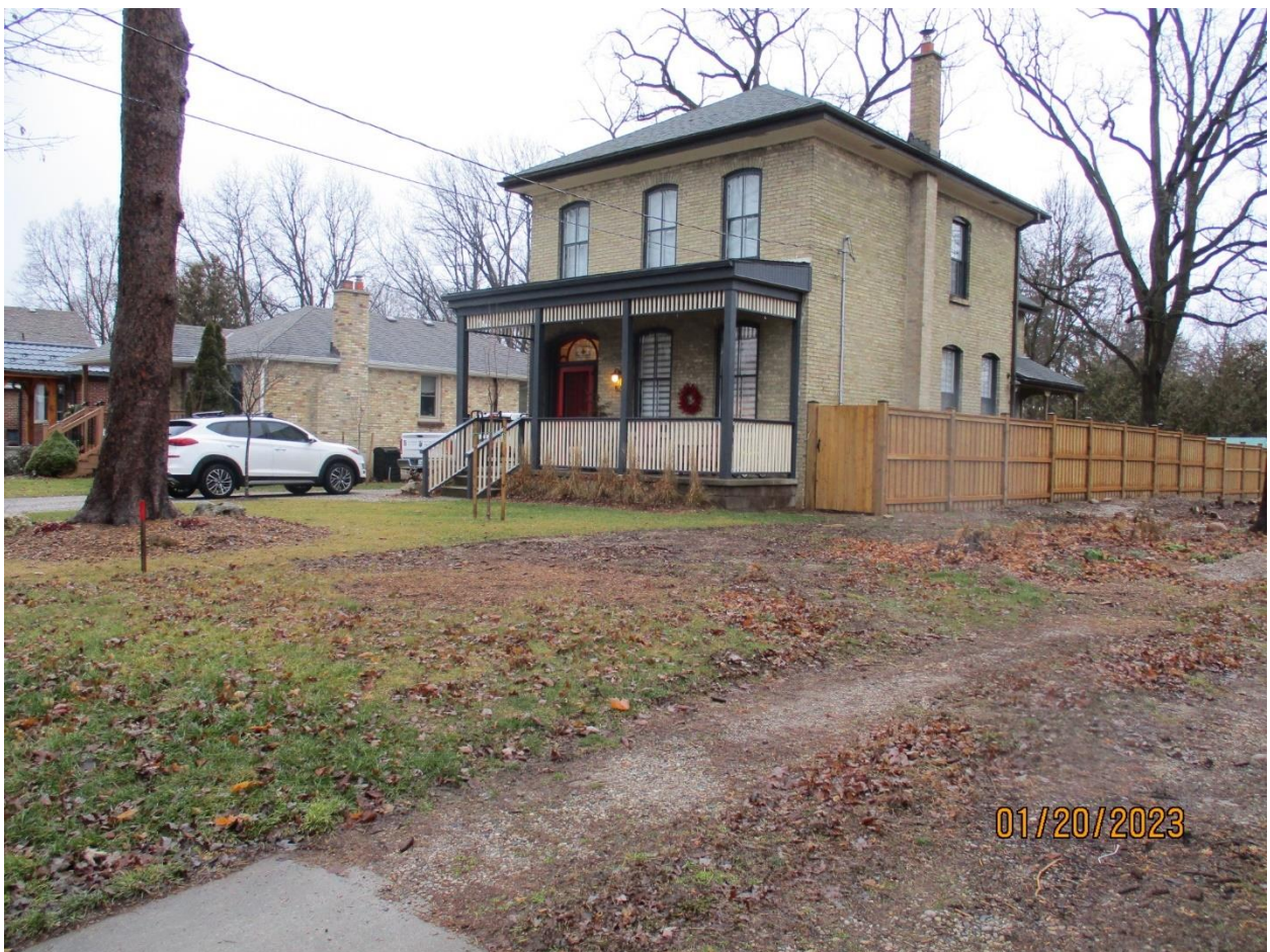
Image 4: Photograph showing the adjacent property at 52 Duchess Avenue, which includes a 2-storey vernacular dwelling with Italianate influences.
