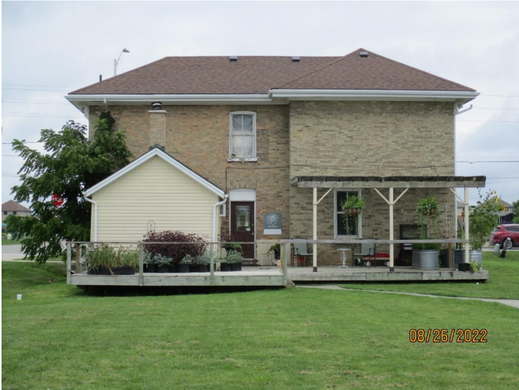
Image 15: Photograph showing the rear (west) façade of the Routledge Farmhouse at 1656 Hyde Park Road, August 26, 2022.
