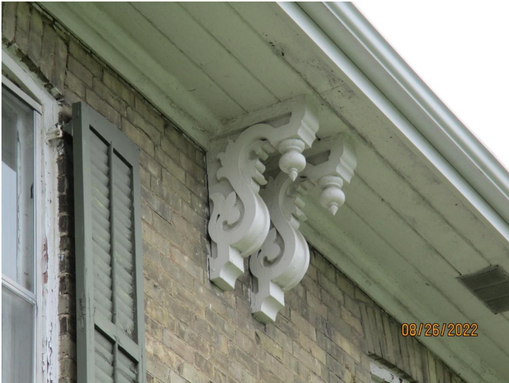
Image 13: Detail showing deep eaves, wood soffit and paired brackets with relief scrollwork and pendant finials, on the Routledge Farmhouse, August 26, 2022.
