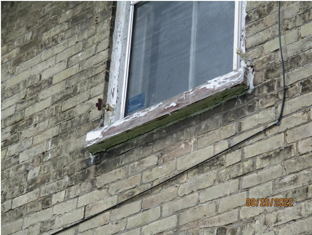
Image 11: Detail showing buff brick and existing wood sills on the Routledge Farmhouse at 1656 Hyde Park Road, August 26, 2022.
