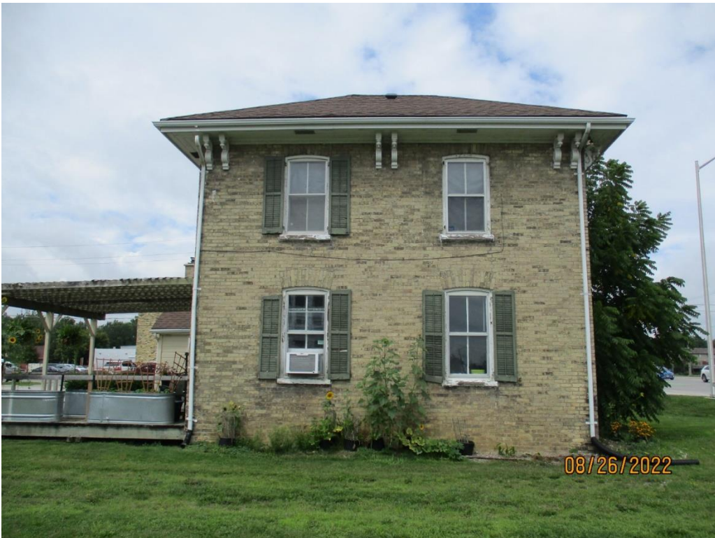
Image 10: Photograph looking north showing the south façade of the Routledge Farmhouse at 1656 Hyde Park Road, August 26, 2022.
