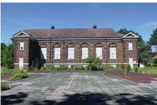
Photo 20: Recreation Hall east elevation looking west
