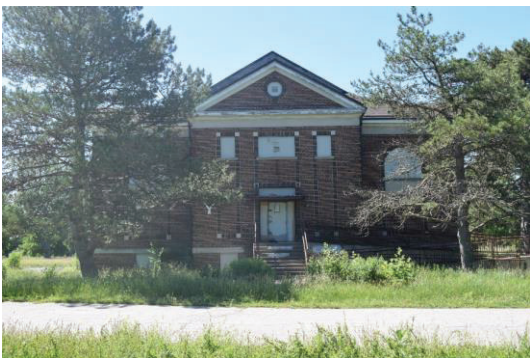
Photo 18: Recreation Hall front (north) elevation looking south
