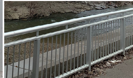
TVP - Existing Railing
