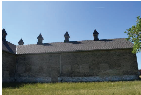
Photo 4: Horse Stable looking south
