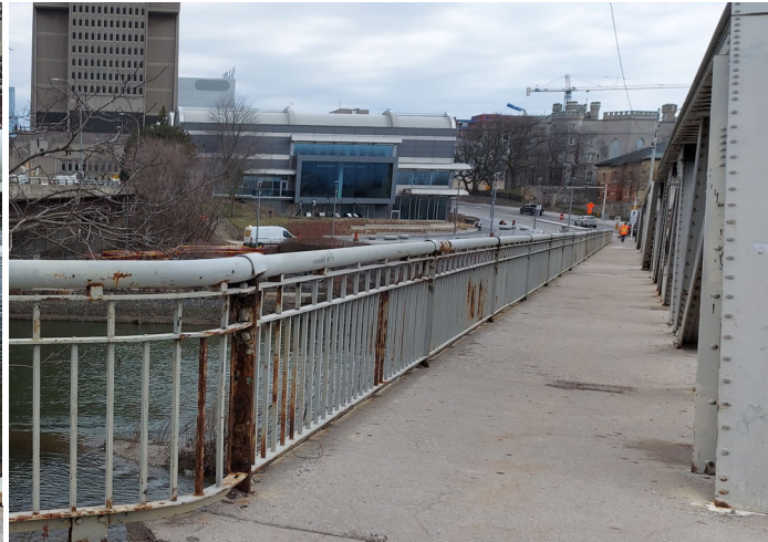
17 Kensington Bridge Existing Railing
