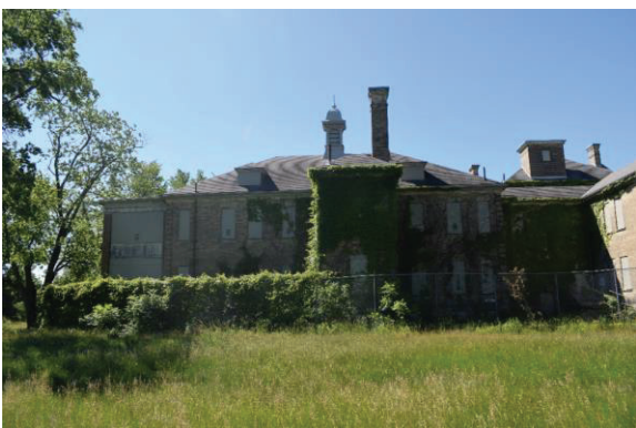
Photo 16: Infirmary rear elevation of east wing looking south
