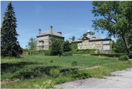
Photo 10: Infirmery south elevation looking northwest
