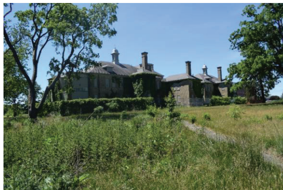
Photo 15: Infirmary north (rear) elevation looking southwest
