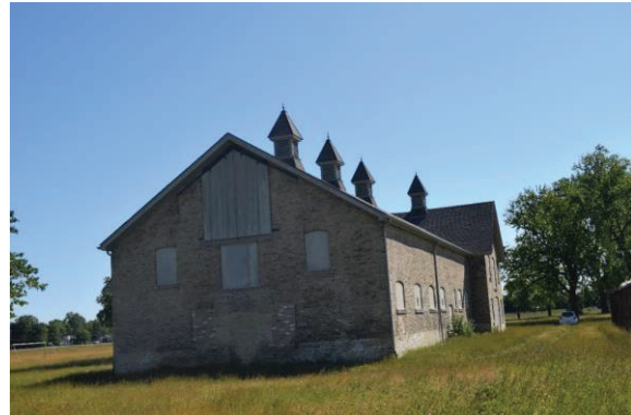
Photo 2: Horse Stable looking northeast
