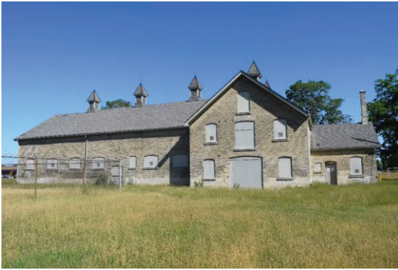
Photo 1: Horse Stable looking northwest
