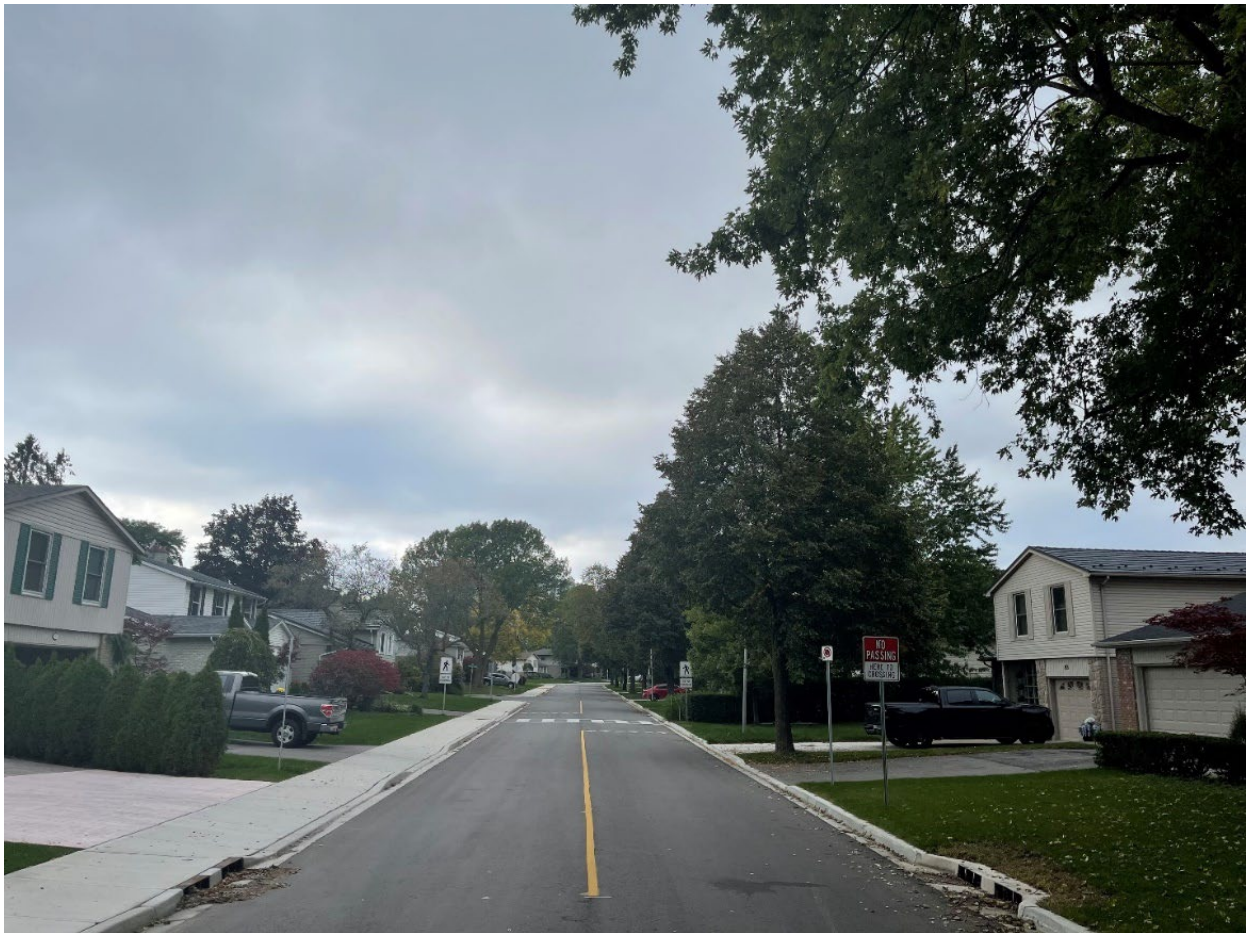
Figure 1: Photo of a completed Local Road Reconstruction Program with a new sidewalk
