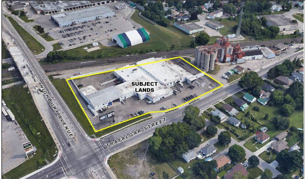
Figure 2: Existing Site Conditions (Aerial View)
