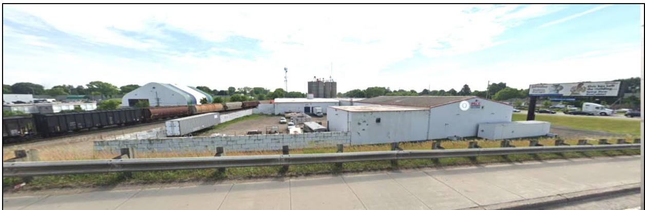
Figure 2: Photo of 1350 Trafalgar Street from Highbury Avenue North (frontage)
