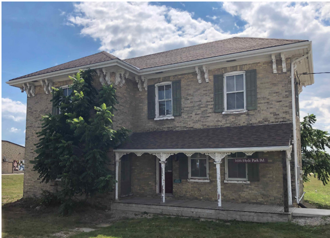
1656 Hyde Park Road- East Elevation (Street Front)
