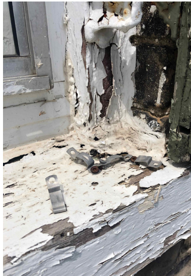
Decay at heritage wood windows, frames, sills and shutters. Photo by: a+LiNK Architecture Inc., 2020
