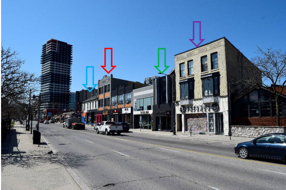
Figure 13: Looking south down Richmond Street, Subject Property located behind structures, 565-569 Richmond Street (blue arrow), 571-575 Richmond Street (red arrow), 579 Richmond Street (green arrow), 581-583 Richmond Street (purple arrow)
