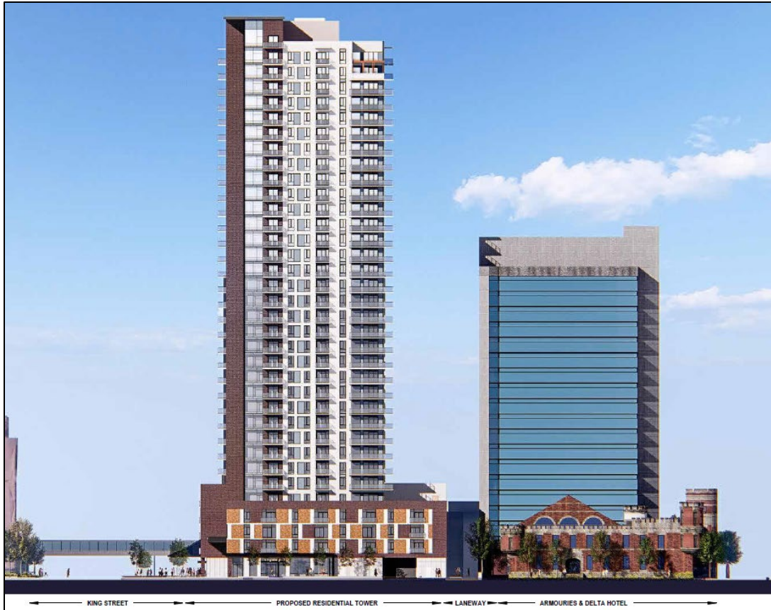
Image 10 – Elevation along Waterloo Street
