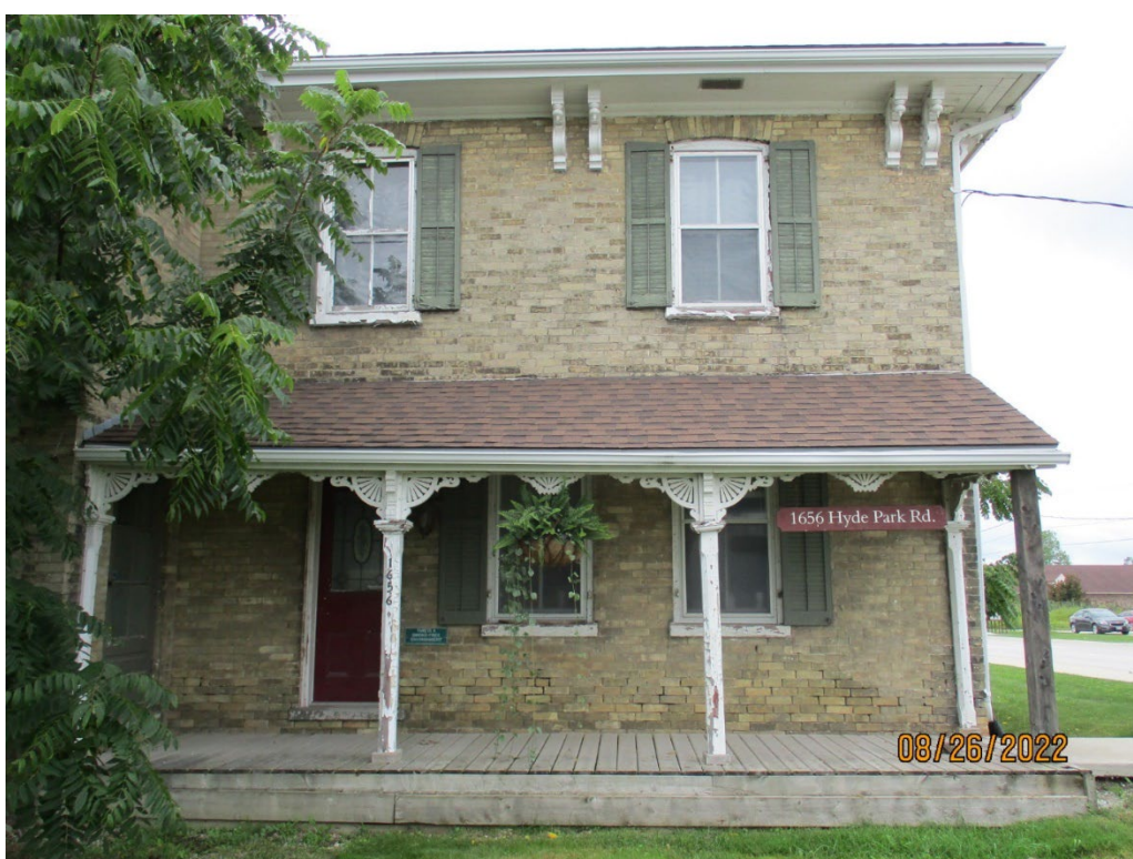
Image 2: View of the Routledge Farmhouse, showing the front (east) façade including verandah, August 26, 2022.
