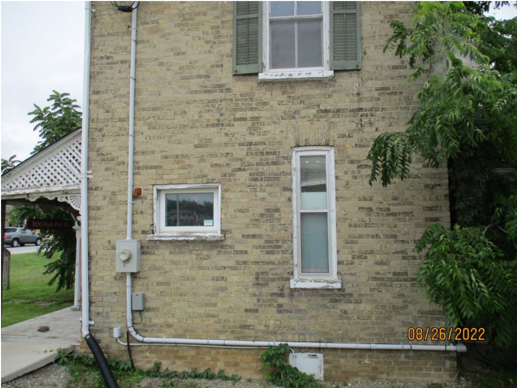
Image 17: Photograph looking south showing the north façade of the Routledge Farmhouse, August 26, 2022.
