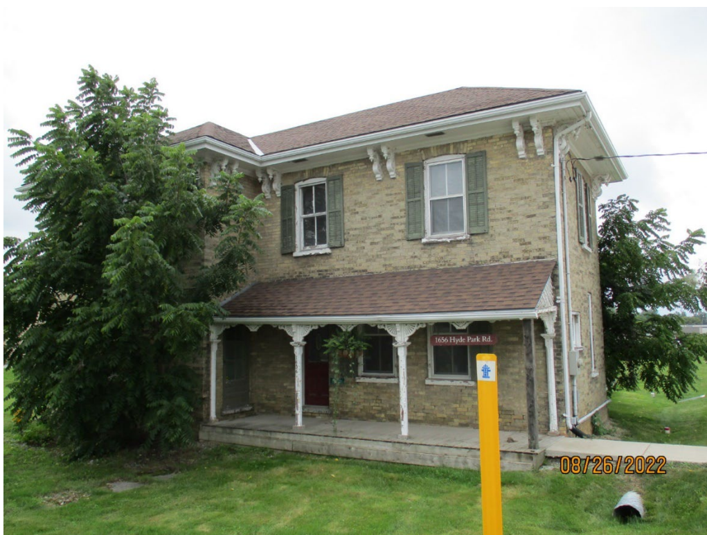
Image 1: View of the property at 1656 Hyde Park Road, looking west to the front (east) facade of the Routledge Farmhouse, August 26, 2022.
