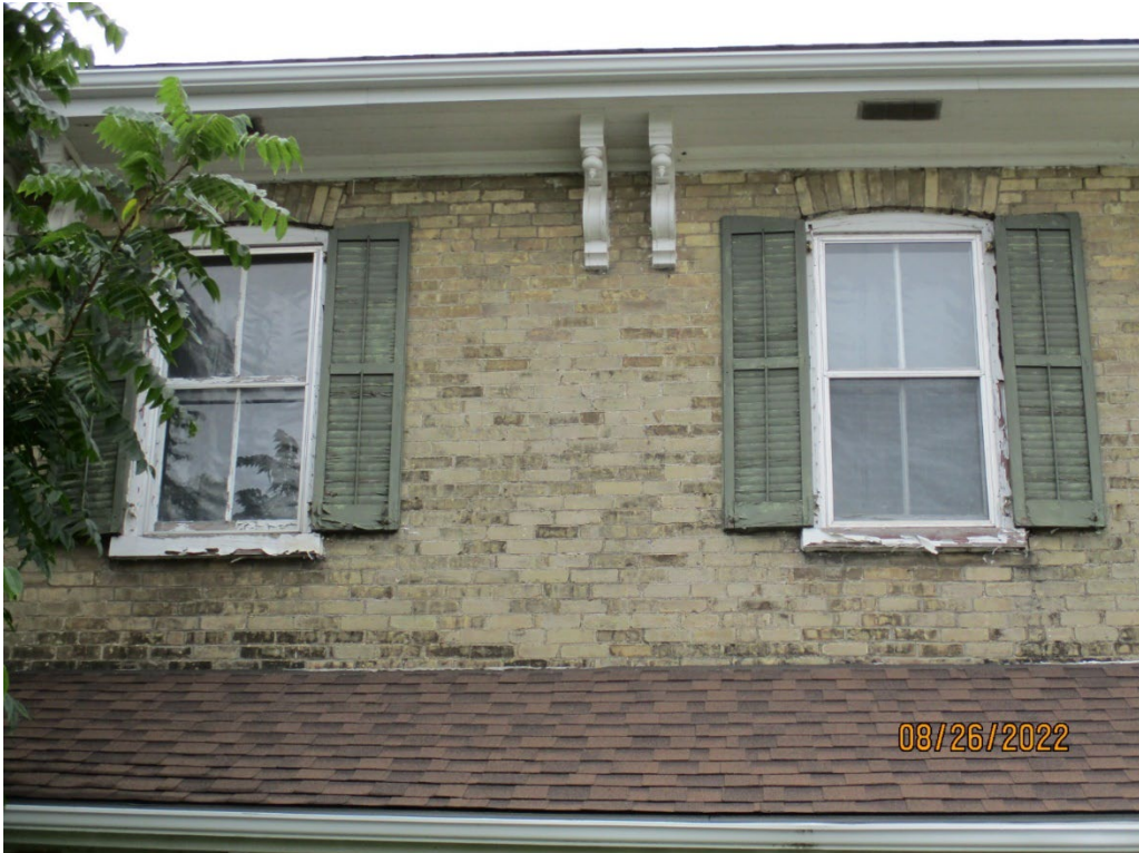
Image 3: View showing the existing double-hung wood windows, with wood shutters, as well as the deep eaves and paired brackets on the Routledge Farmhouse, August 26, 2022.
