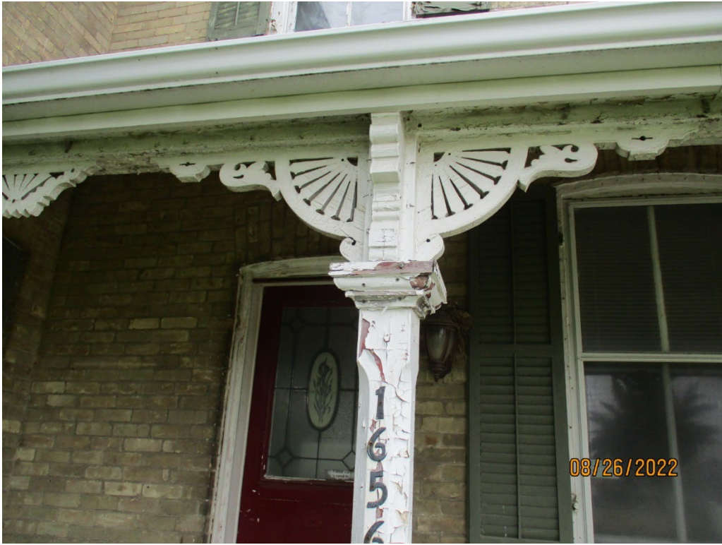
Image 7: Detail showing the chamfered posts, capitals, and fretwork found on the porch on the Routledge Farmhouse, August 26, 2022.
