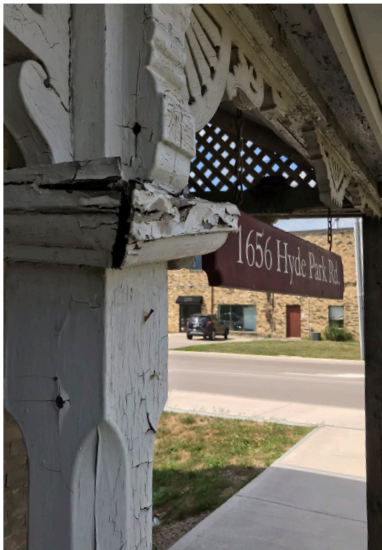
Existing front porch, east elevation. Photo by: a+LiNK Architecture Inc., 2020
