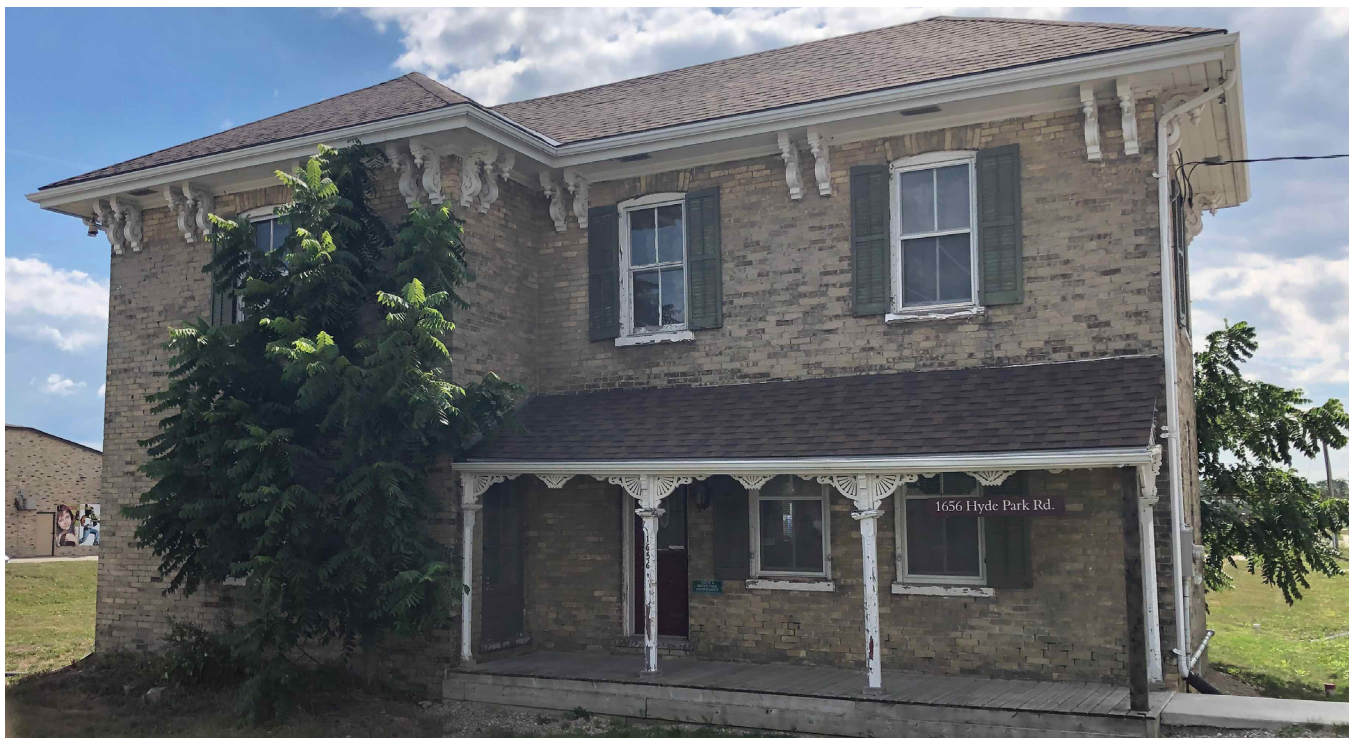
1656 Hyde Park Road. Main/East elevation. Photo by: a+LiNK Architecture Inc., 2020
