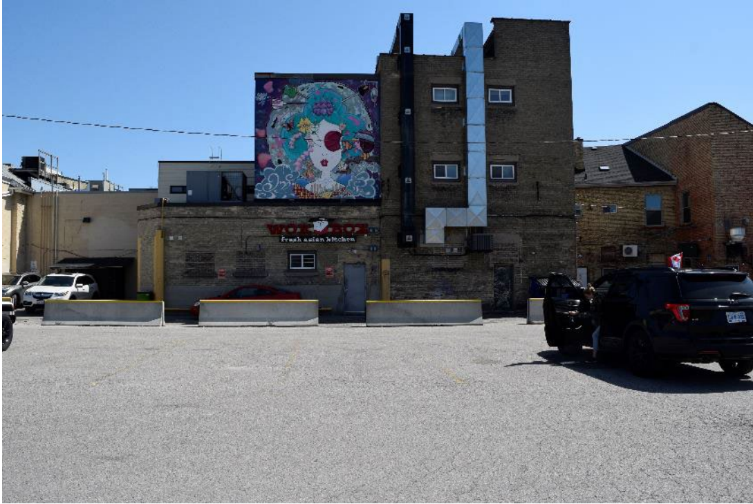
Figure 18: Looking east from centre of 200 Albert Street
