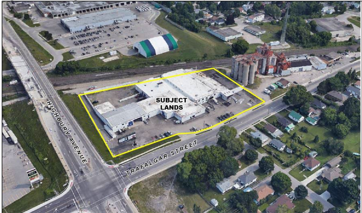
Figure 2: Existing Site Conditions (Aerial View)
