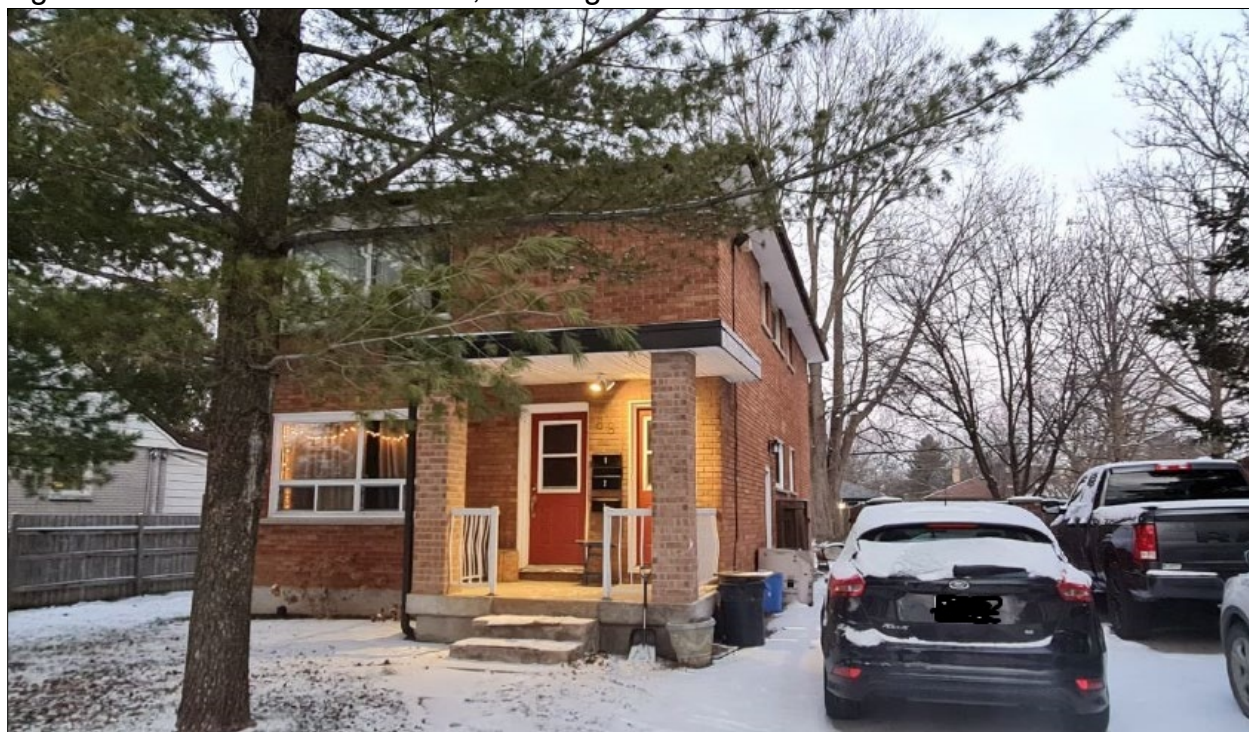
Figure 1: 88 Chesterfield Avenue, Looking Southwest
