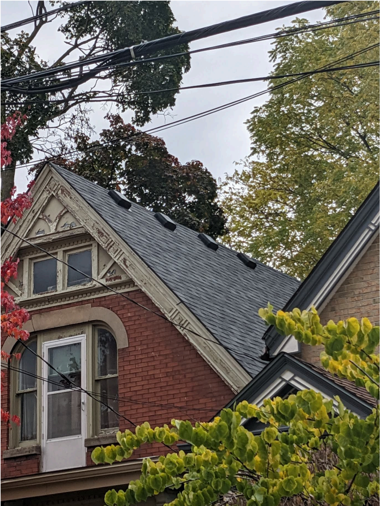
Image 6: Photograph submitted as a part of the pre-consultation process for the Heritage Alteration Permit application showing the unapproved asphalt shingles.
