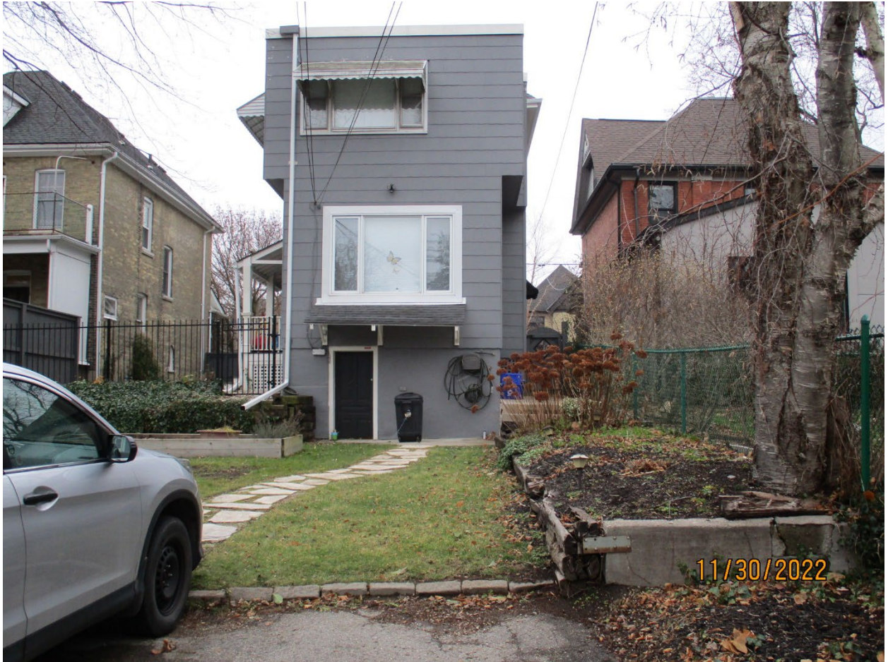
Image 6: Photograph showing at grade entry to the rear of the property at 864 Hellmuth Avenue.
