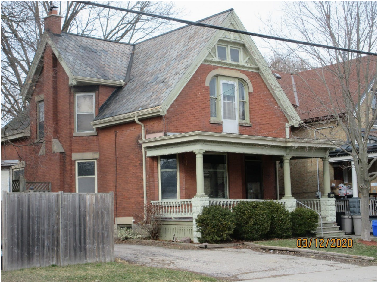
Image 3: Photograph showing the dwelling located at 892 Princess Avenue, showing original slate roof (2020).
