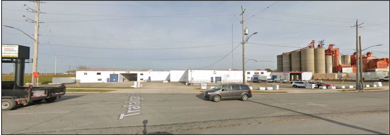
Figure 1: Photo of 1350 Trafalgar Street from Trafalgar Street
