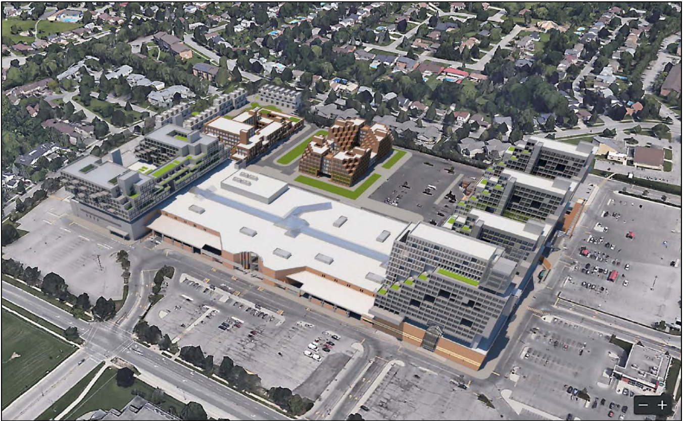
Overall Site View
