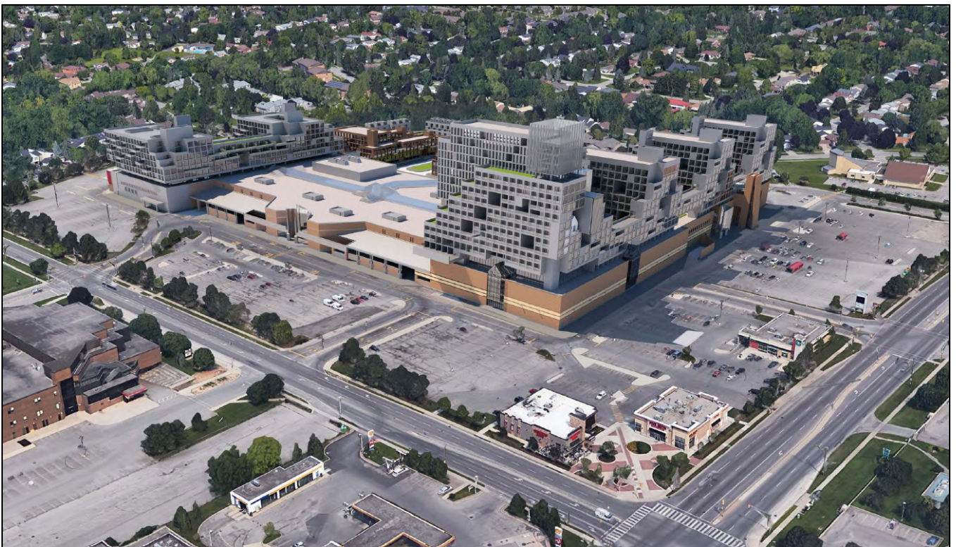
Northwest View – Wonderland Road South
