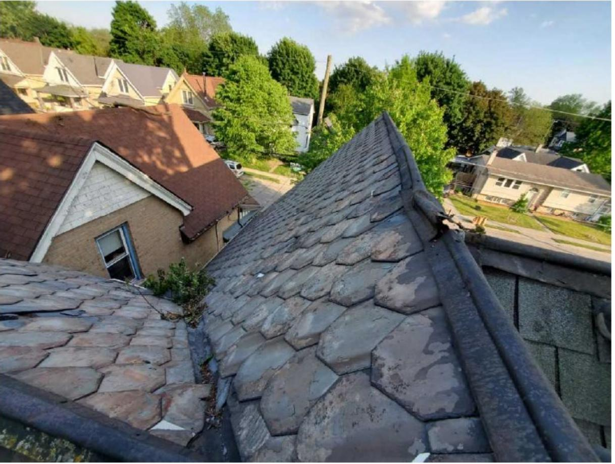
*Image 12: Photograph submitted as a part of an inspection report showing extent of damage to the slate roof.*
