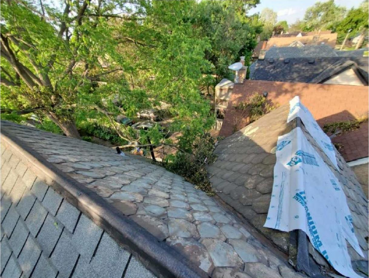
*Image 11: Photograph submitted as a part of an inspection report showing extent of damage to the slate roof.*
