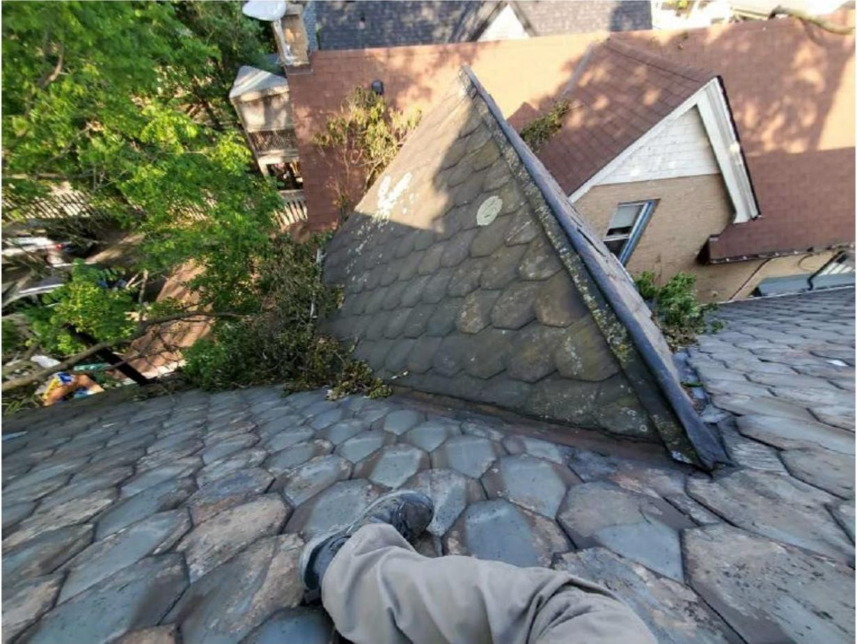
*Image 13: Photograph submitted as a part of an inspection report showing extent of damage to the slate roof.*
