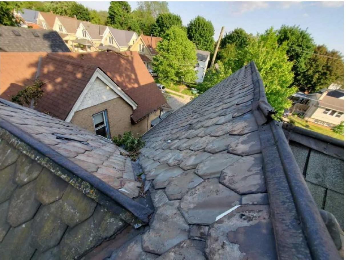
*Image 10: Photograph submitted as a part of an inspection report showing extent of damage to the slate roof.*
