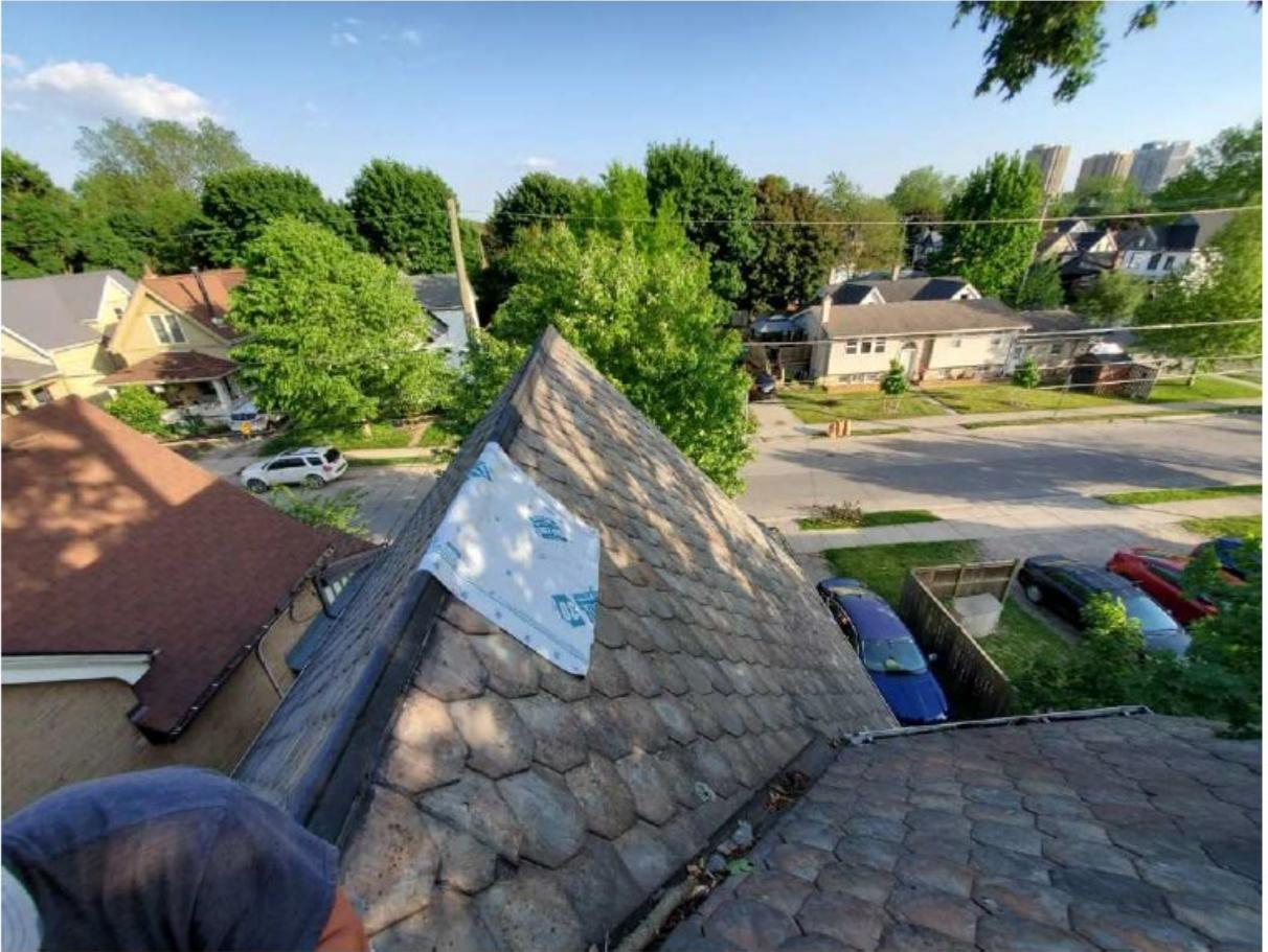
*Image 9: Photograph submitted as a part of an inspection report showing extent of damage to the slate roof.*
