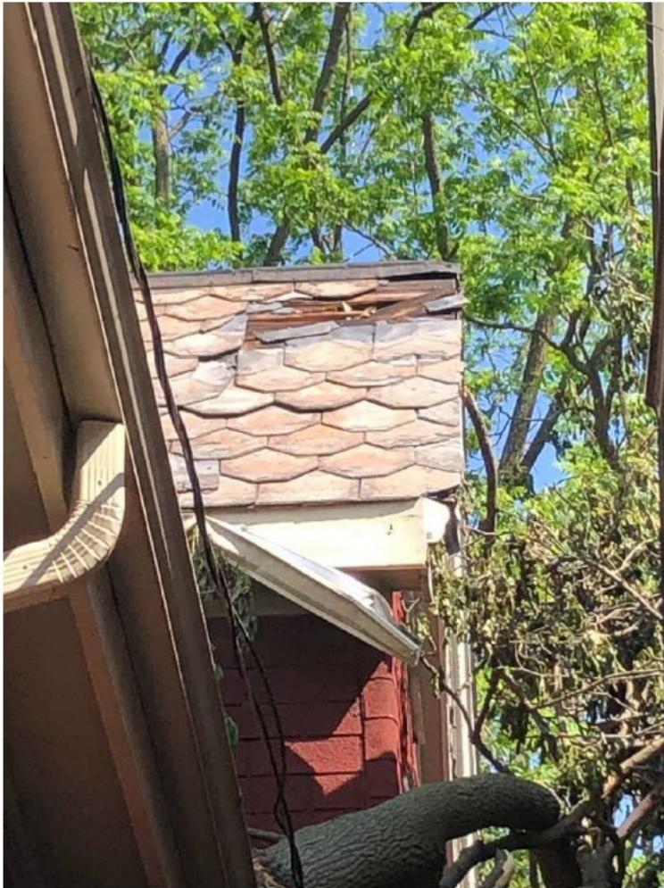
*Image 7: Photograph submitted as a part of an inspection report showing extent of damage to the slate roof.*
