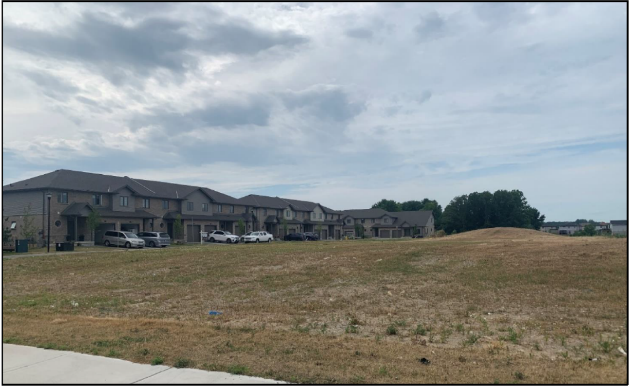
Figure 1. View of the Subject Lands, Looking Northwest on Tokala Trail, July 2022
