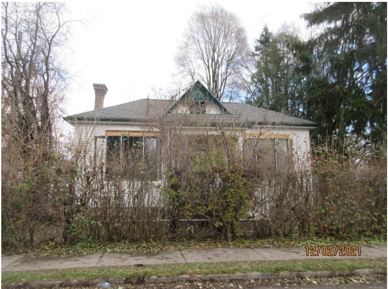
Image 2: View through the overgrown hedge at 123 Wilson Avenue, showing the alterations to the window openings on west façade.
