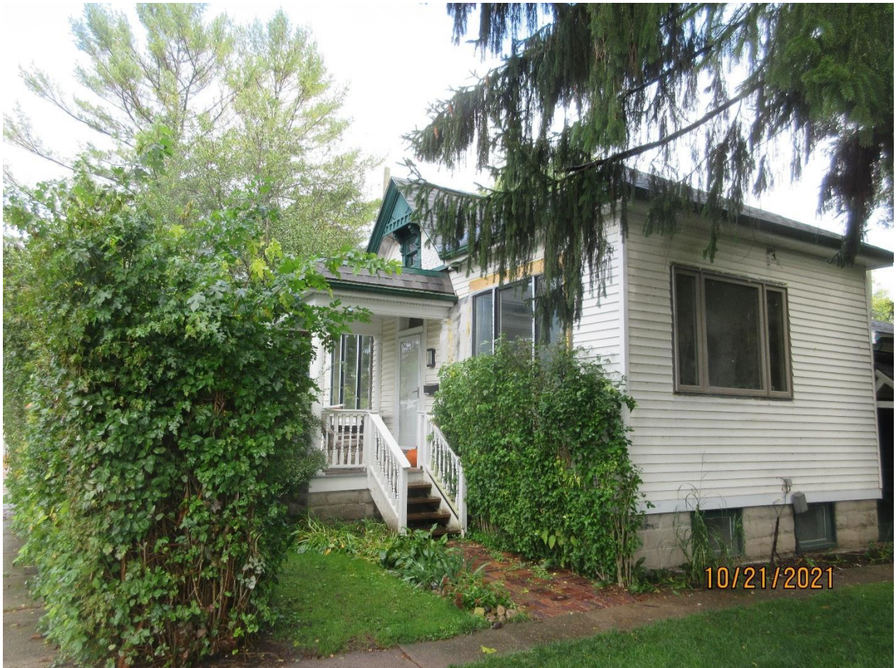
Image 4: View showing the south half of the main façade and south façade of the Contributing Resource on October 21, 2021.
