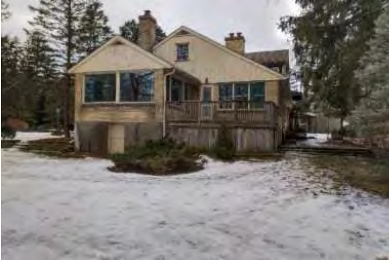
Photo 10: Existing house (back view) and backyard
