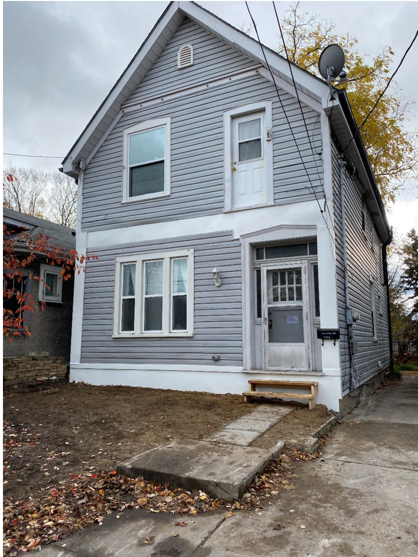
Image 3: Photograph, submitted as part of the Heritage Alteration Permit application, showing the current condition of the property at 645 Lorne Avenue.
