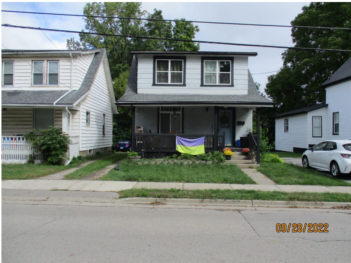
Image 2: Photograph showing the property located at 10 Moir Street, located within the Blackfriars/Petersville Heritage Conservation District. Note, the existing front yard consists of manicured grass.
