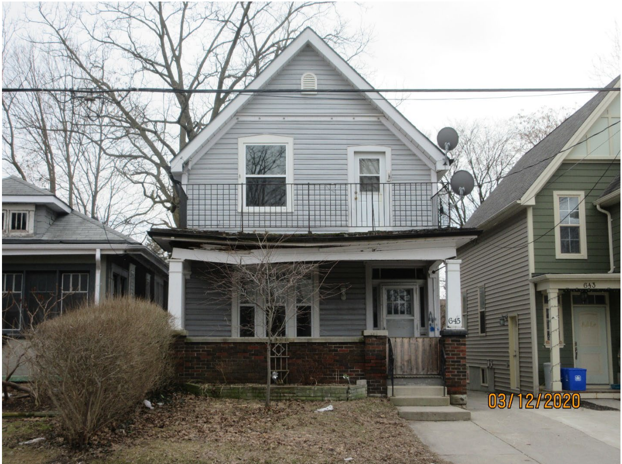
Image 1: Photograph of the heritage designated property at 645 Lorne Avenue on March 12, 2020.
