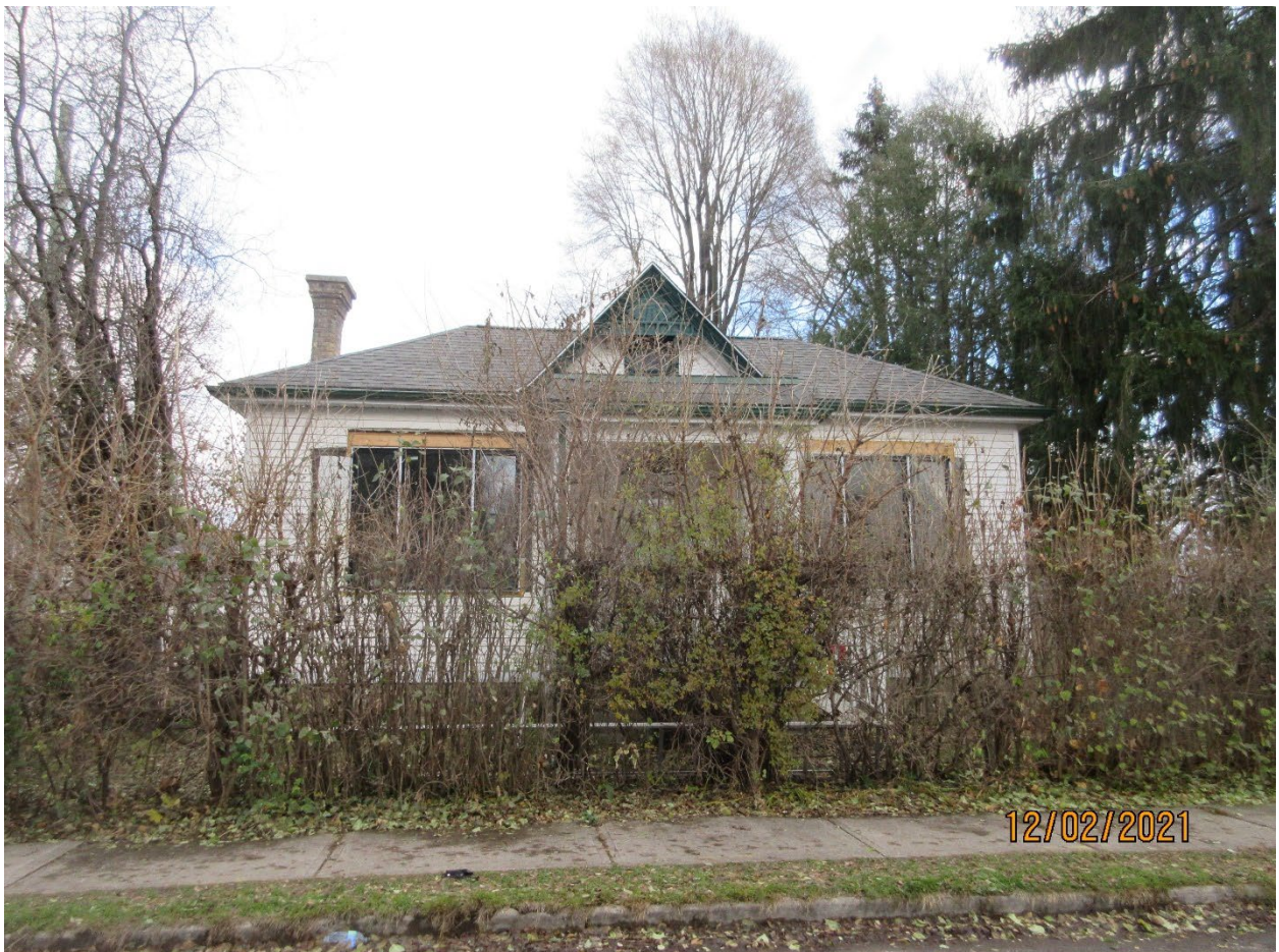
Image 2: View through the overgrown hedge at 123 Wilson Avenue, showing the alterations to the window openings on west façade.
