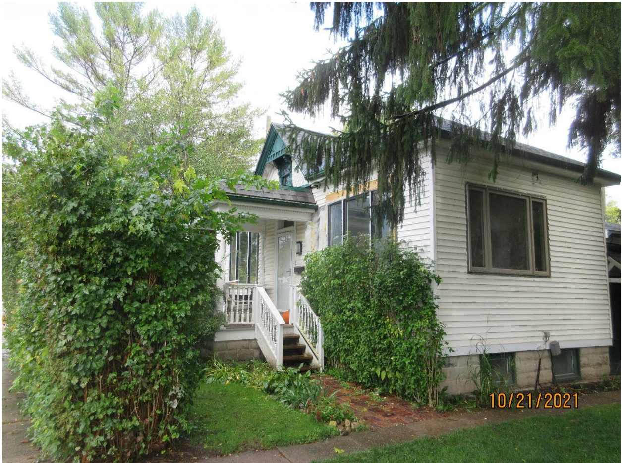
Image 4: View showing the south half of the main façade and south façade of the Contributing Resource on October 21, 2021.
