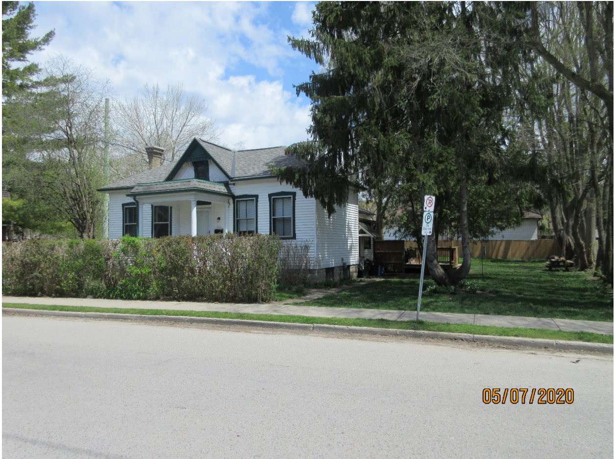
Image 3: View of the main (west) and south façades of the Contributing Resource at 123 Wilson Avenue on May 5, 2020.
