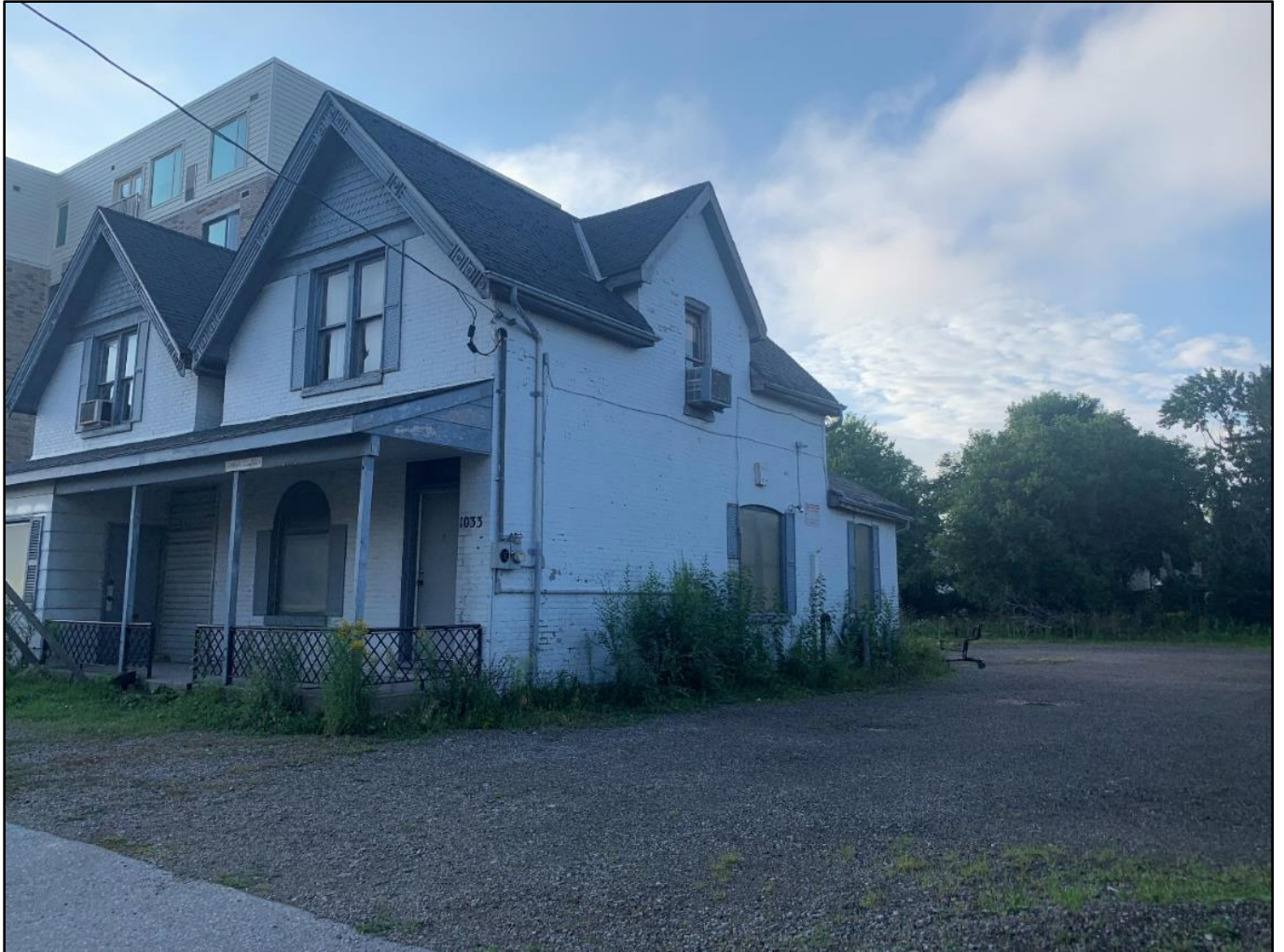
Figure 2. 1033 Dundas Street, Facing Southeast (Aug 2022)
