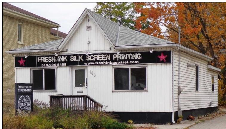
**Exterior** - The Building, which is setback 7.3 feet (2.22 metres) from the Wellington Street right-of-way, is a single detached, one storey frame structure clad in white, modern synthetic siding imitating vertical boards on the front elevation and horizontal clapboards on the side and rear elevation. The front section of the Building rests on a brick foundation that has been parged with a thin surface of mortar painted.
