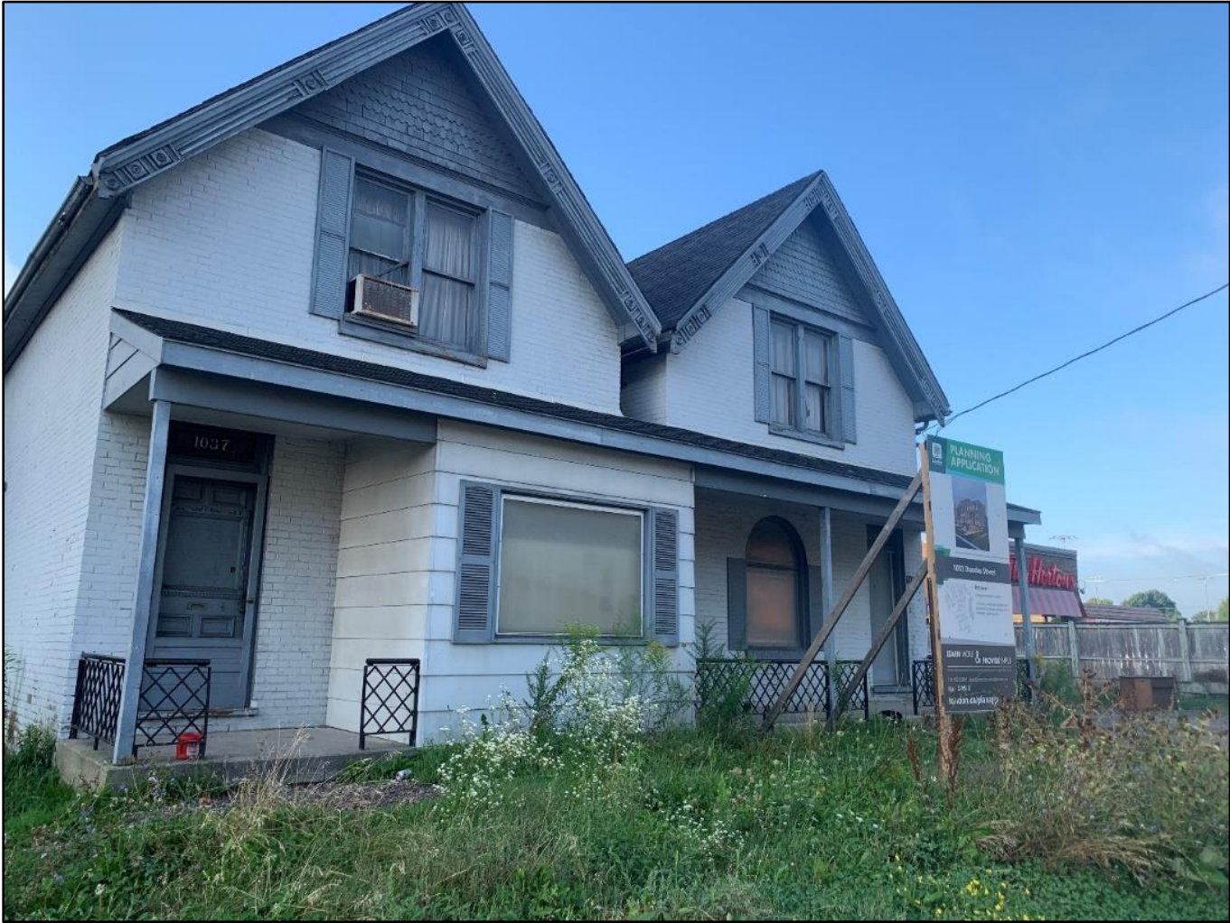
Figure 1. 1033 Dundas Street, Facing South (Aug 2022)
