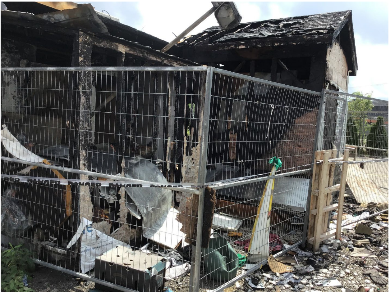
421 Wharncliffe Rd S – rear exterior
