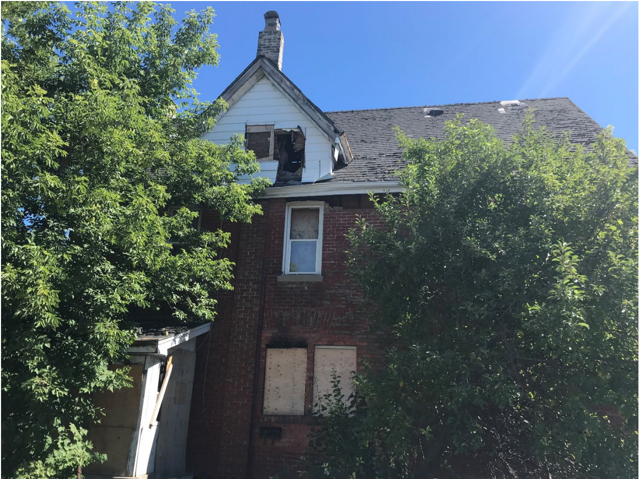
254 Hamilton Road – West Side
