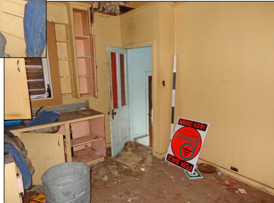
10. Room 4 – South and West Wall and Door to Basement Stairs.
