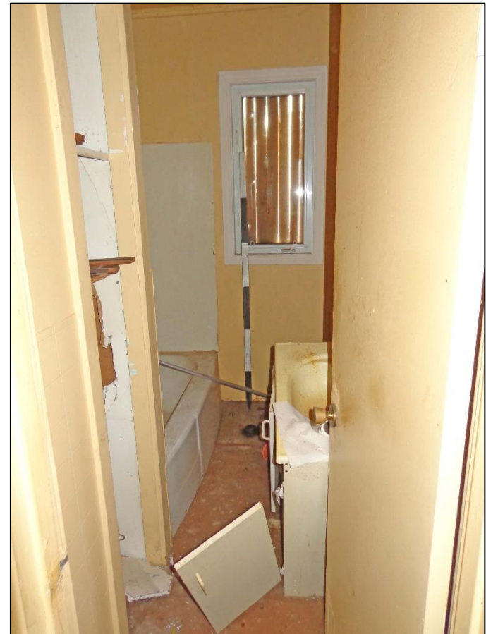
18. Room 7 – View from Hall to North Wall.
