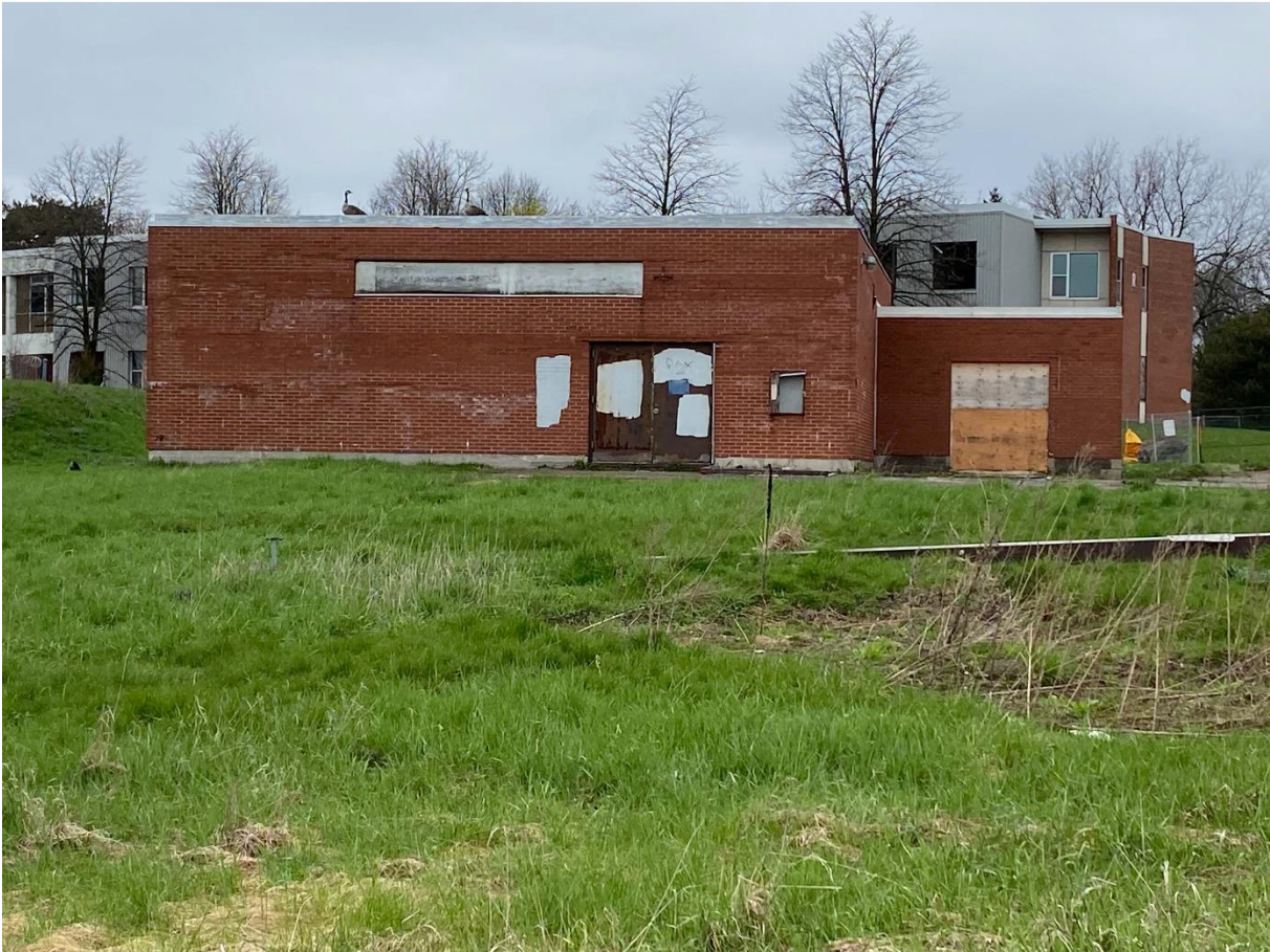
Image 4. Pump House (B12015), facing north – L. Dent, May 2022
