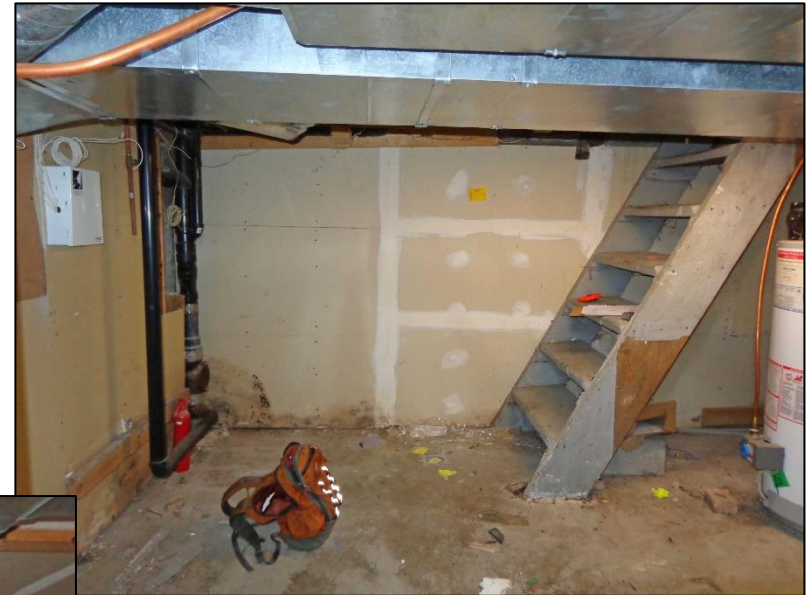
1. Room 1 – East and South Walls.
