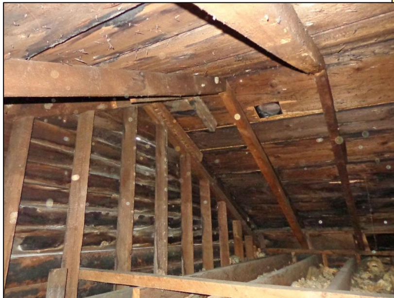
1. Attic – Front Section – View North and East.
