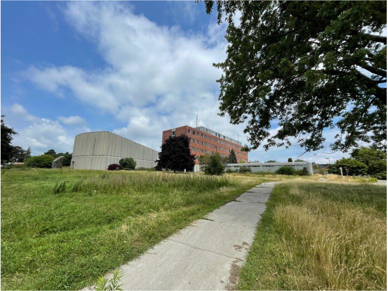
Image 5. South Pavilion Building and Extensions – as noted on project plan (including B12007, B12008, and B12012), facing northeast – Old Oak Properties, July 2022
