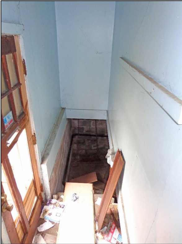
11. Room 4 – Stairs down to Basement and Door to Outside.
