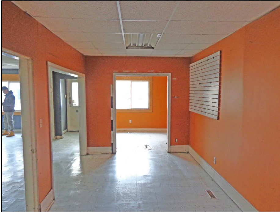
12. Room 3 – North, East and South Walls.
