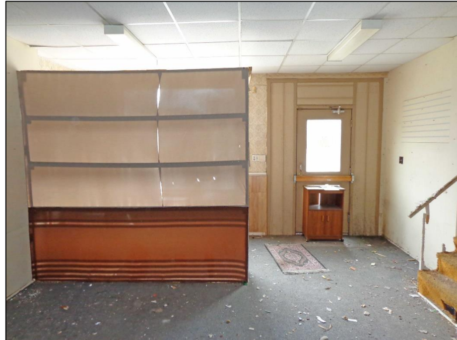
1. Room 1 – North, East and South Walls.
