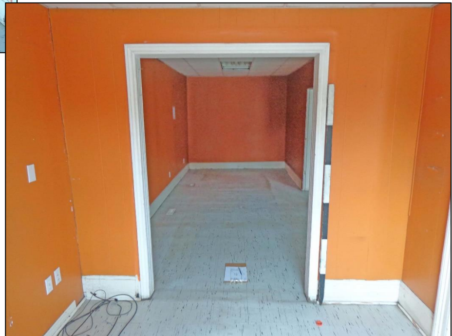
11. Room 2 – West Wall.
