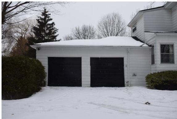
Plate 30: Garage and shed roof addition, looking east
