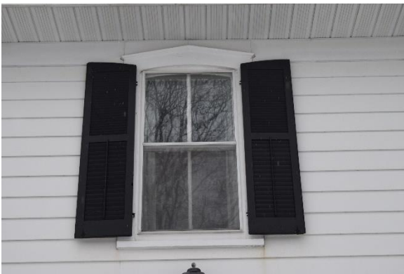
Plate 19: Window details, looking south
