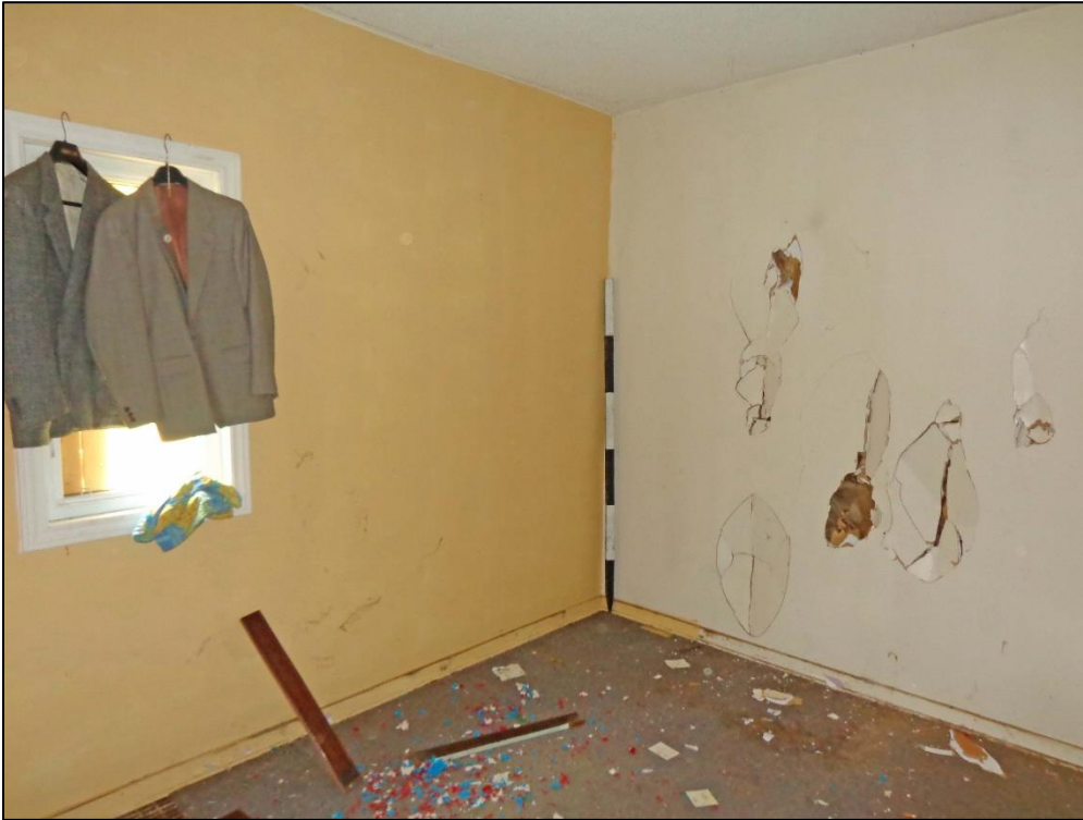
17. Room 6 – West and North Wall.
