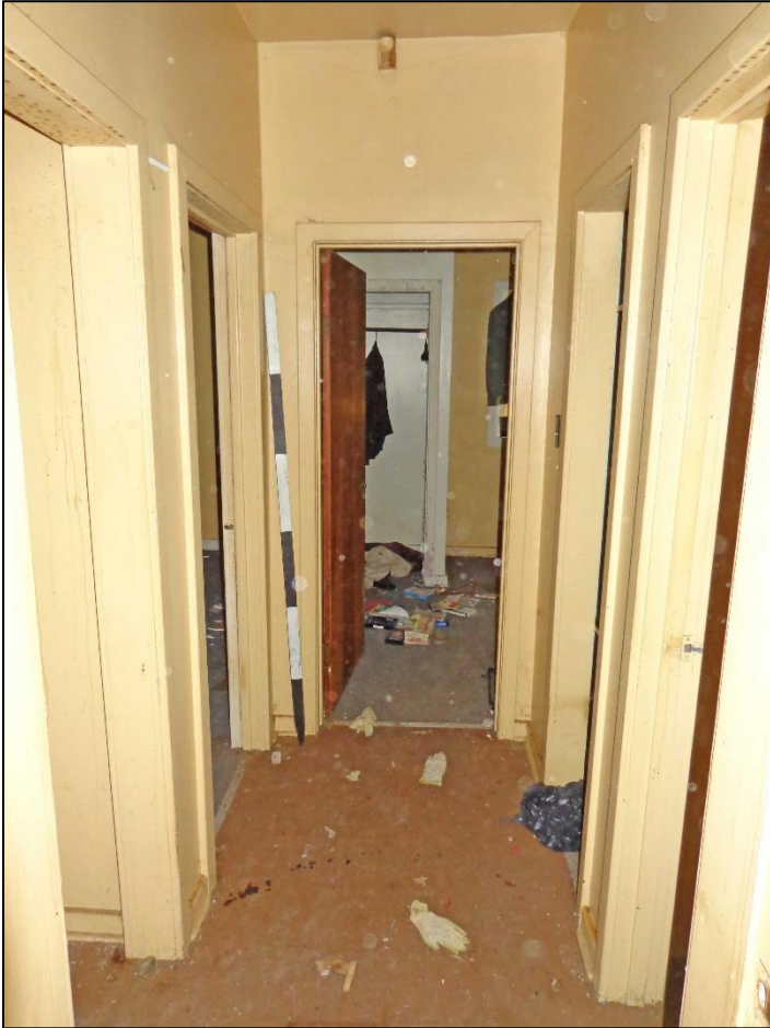
15. Hall – View West to Room 6.
