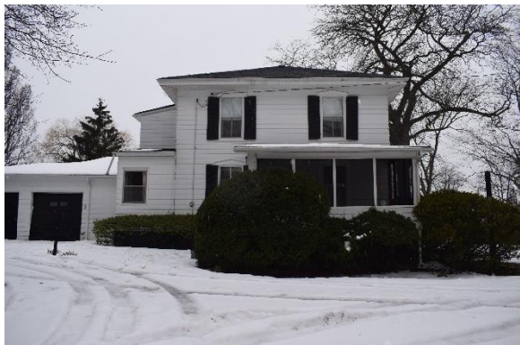
Plate 29: East elevation, looking west
