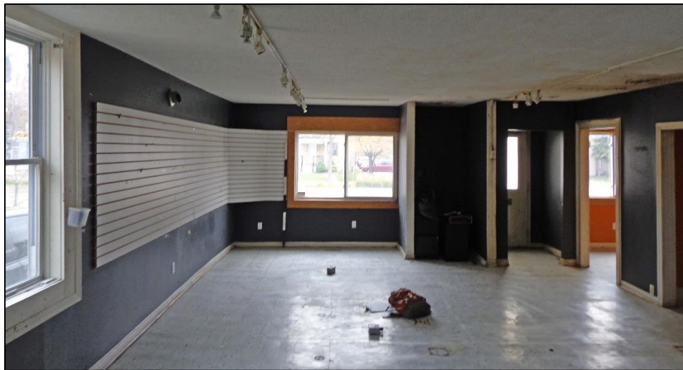
2. Room 1 – North, East and South Walls.
