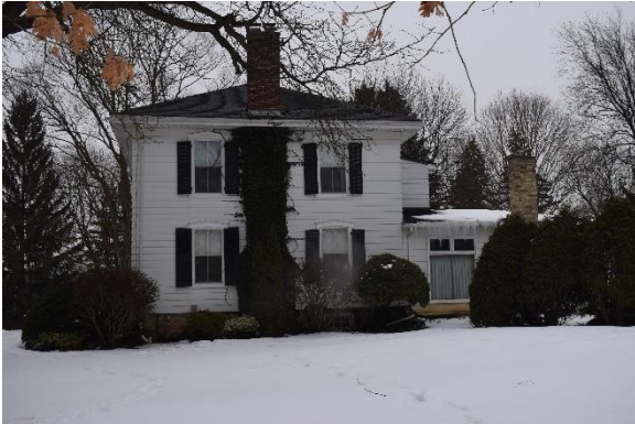
Plate 23: West elevation, looking east
