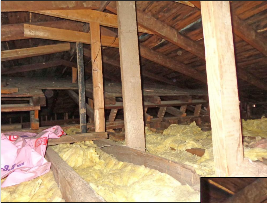
3. Attic – Tail Wing – View East to Front Section.
