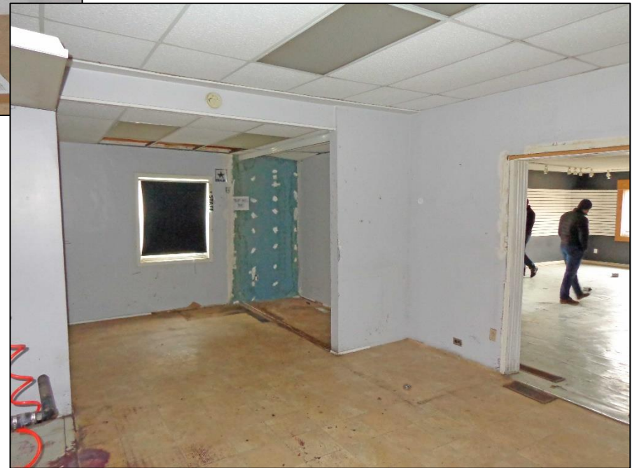
15. Room 4 – North and East Walls.
