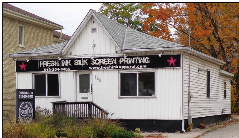
Figure 5.1 185 Wellington Street, East and North Elevations, 2020
