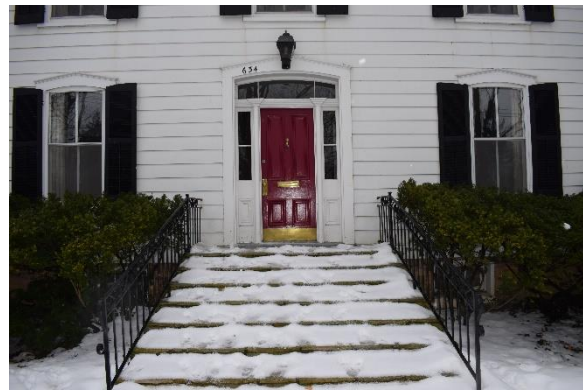
Plate 20: First storey showing windows and doors
