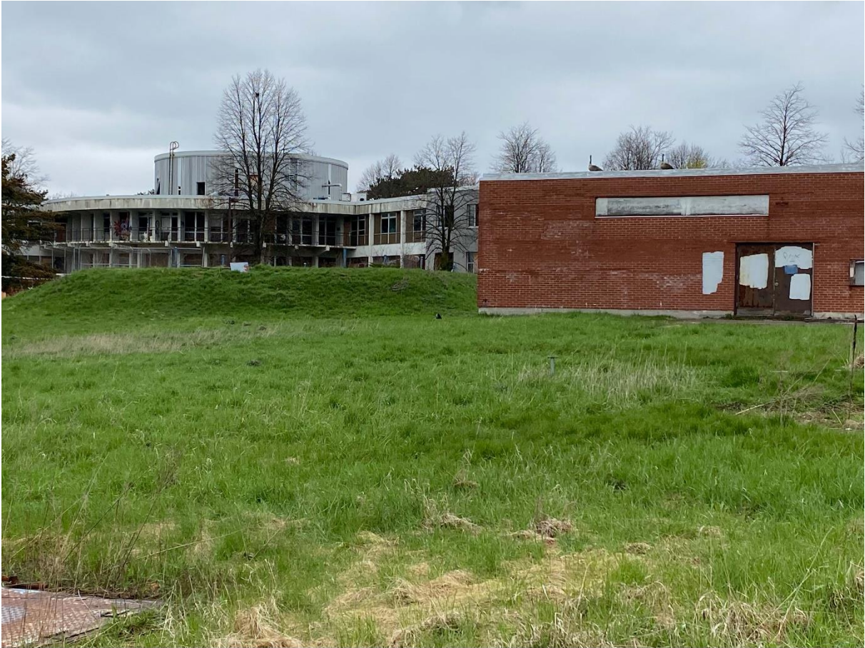
Image 3. Pump House & Underground Water Storage Tank (B12015, B16184), facing northwest – L. Dent, May 2022
