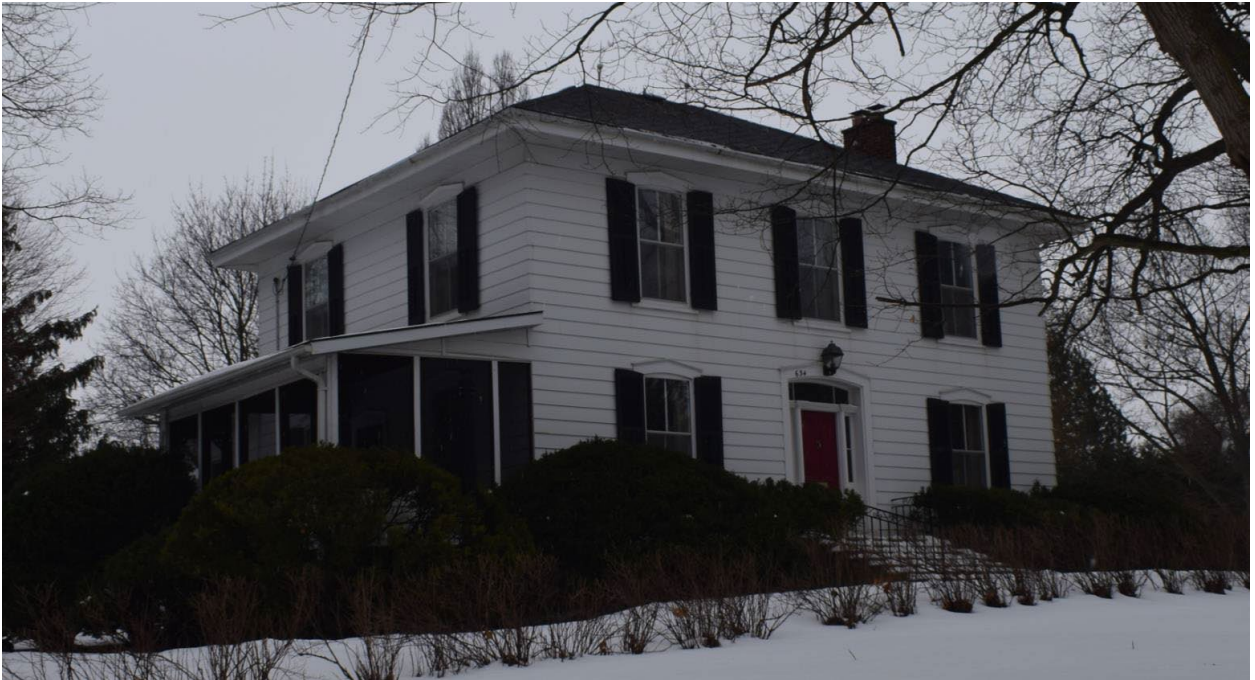
Image 5: Looking northeast showing hip roof, brick chimney, siding, and square plan (Stantec, 2022 p28-plate 14)
