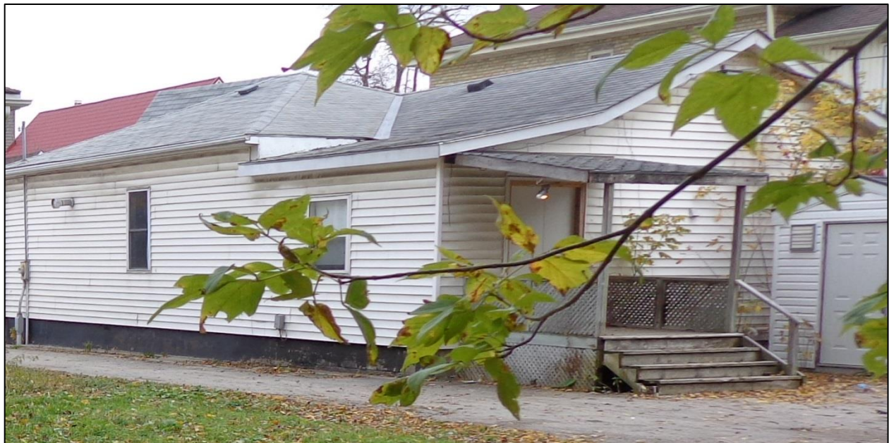
North and West Elevations
