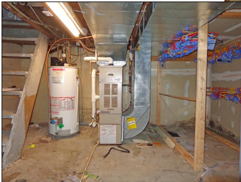
2. Room 1 – West and North Walls.
