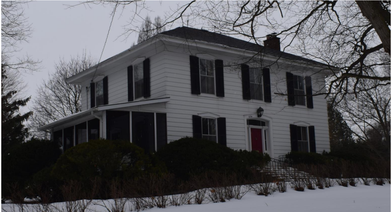
Plate 14: Looking northeast showing hip roof, brick chimney, siding, and square plan
