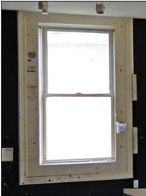
5. Room 1 – Window, North Wall, Detail - new mouldings.
