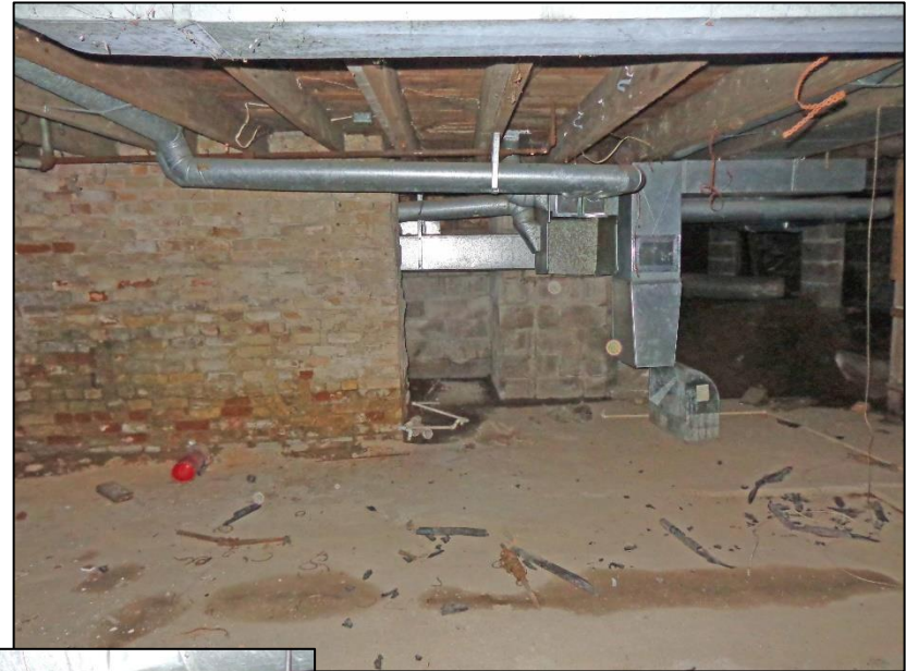
4. Room 1 – East Wall and access to Crawl Space..
