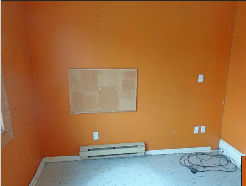
10. Room 2 – South Wall.
