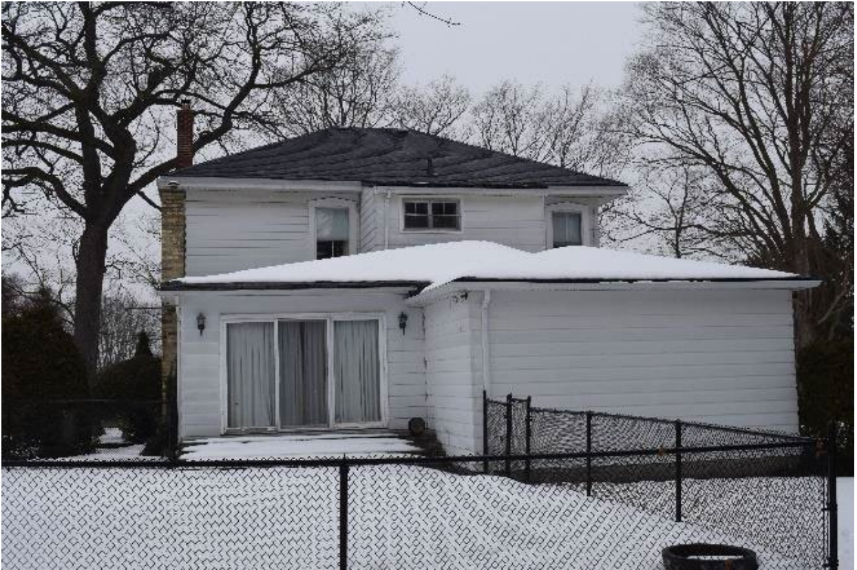
Image 7: South elevation, looking north (Stantec, 2022 p30-plate 26)
