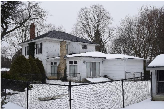
Plate 27: Hip roof addition, looking northeast
