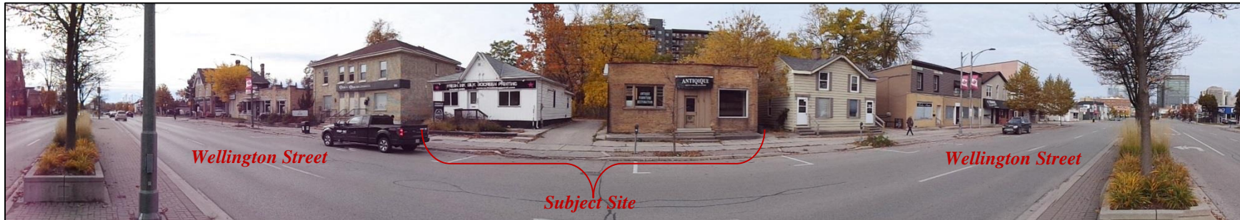
West side of Wellington Street, including subject site.
