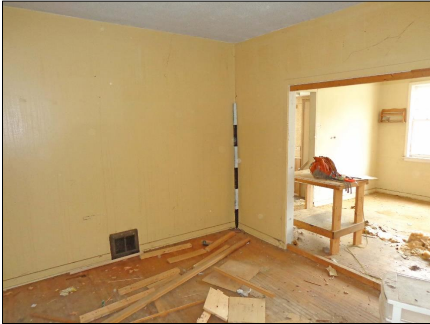
7. Room 3 –North and East Walla and Entrance to Room 2.
