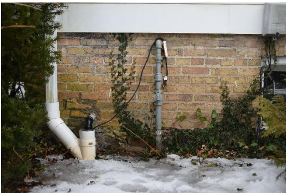
Plate 15: General view of foundation, looking west
