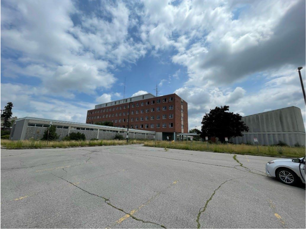
Image 6. South Pavilion Building and Extensions – as noted on project plan (including B12007, B12008, and B12012), facing southeast – Old Oak Properties, July 2022
