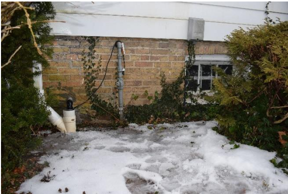
Plate 25: Basement window, looking east
