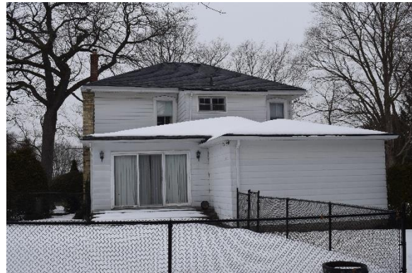
Plate 26: South elevation, looking north
