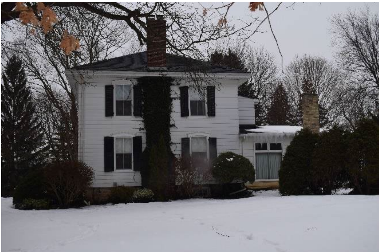
Image 2: West elevation looking east (Stantec, 2022 p30-plate 23)
