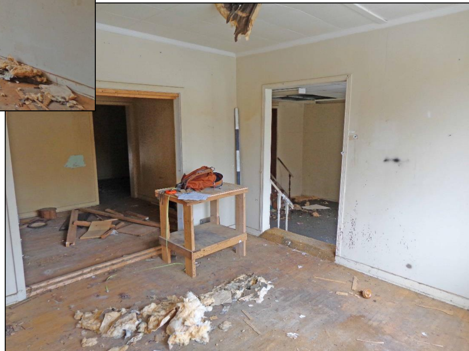
6. Room 2 – West and North Walla and Entrance to Rooms 3 and 1.
