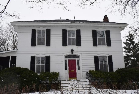
Plate 17: Main elevation, looking south
