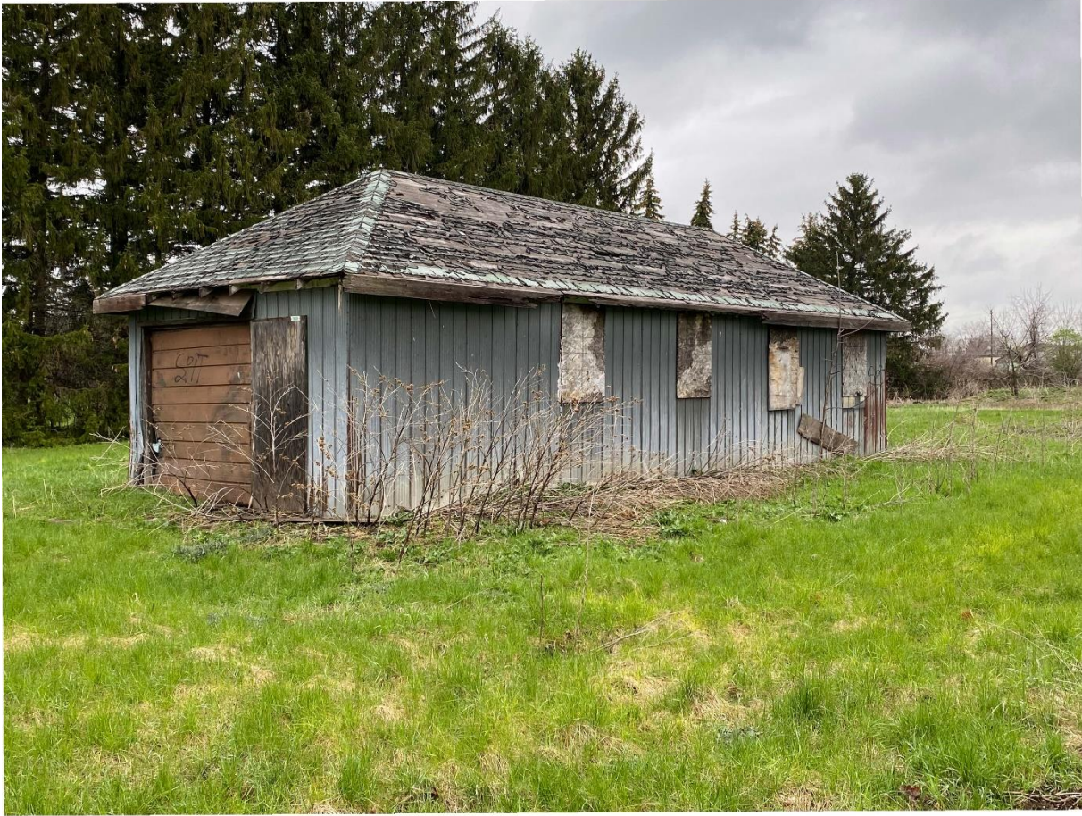
Image 1. Garage (B12001), facing northeast – L. Dent, May 2022
