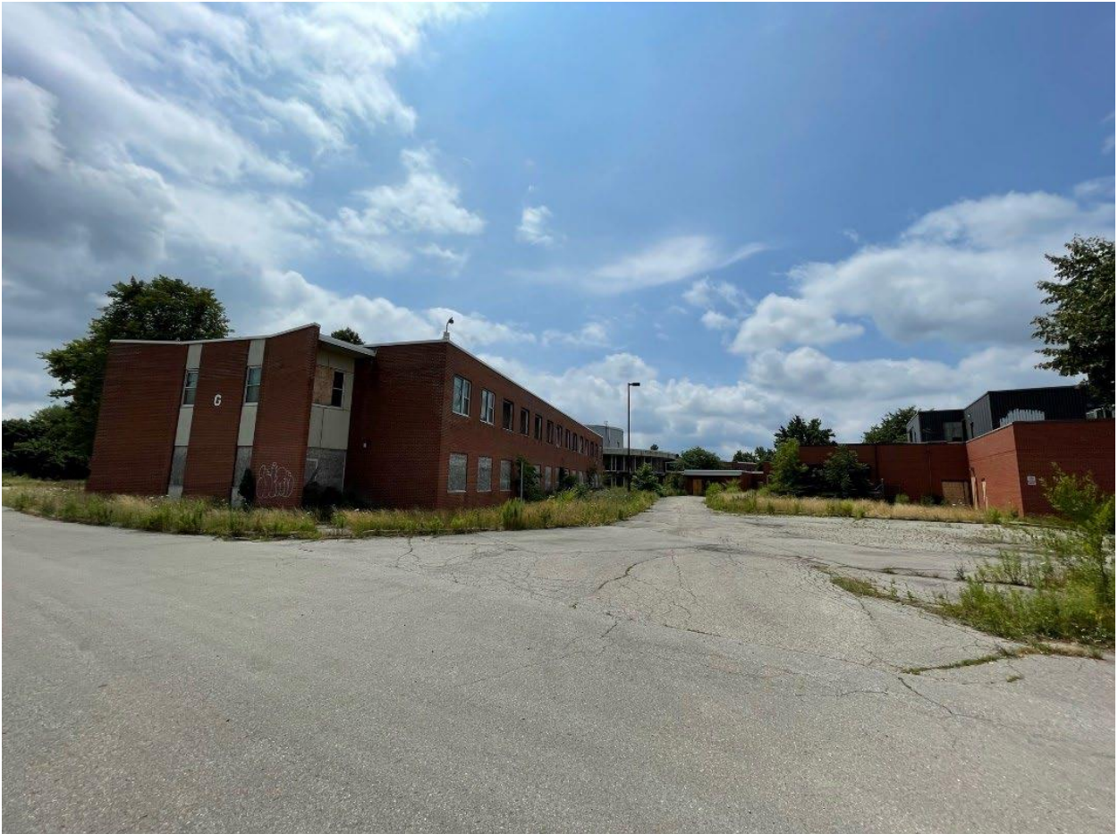
Image 9. South Pavilion Building and Extensions – as noted on project plan (including B20794, B12009, B12011, and B12014), facing southwest – Old Oak Properties, July 2022
