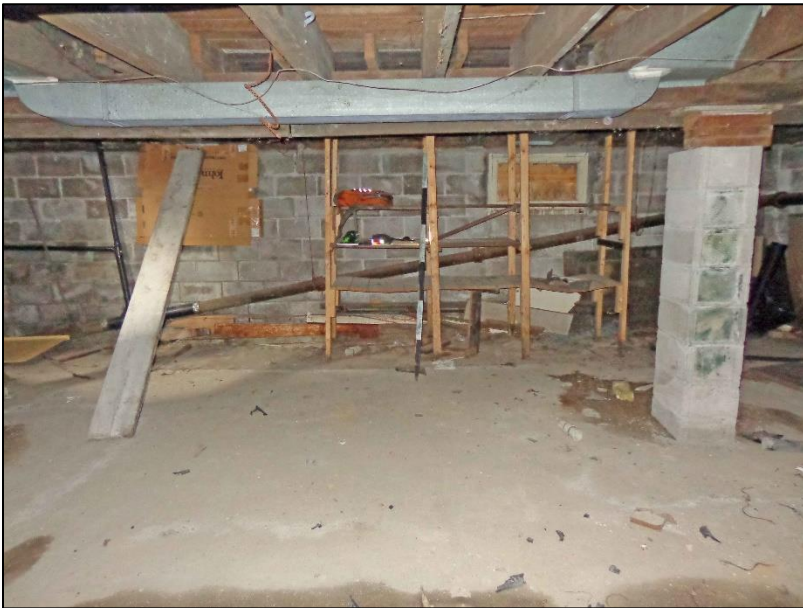
2. Room 1 – West Wall.
