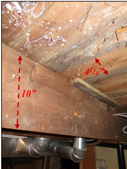
5. Room 1 – Ceiling joists and floorboards.
