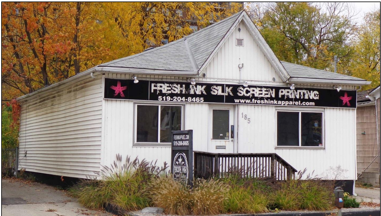
South and East Elevations
