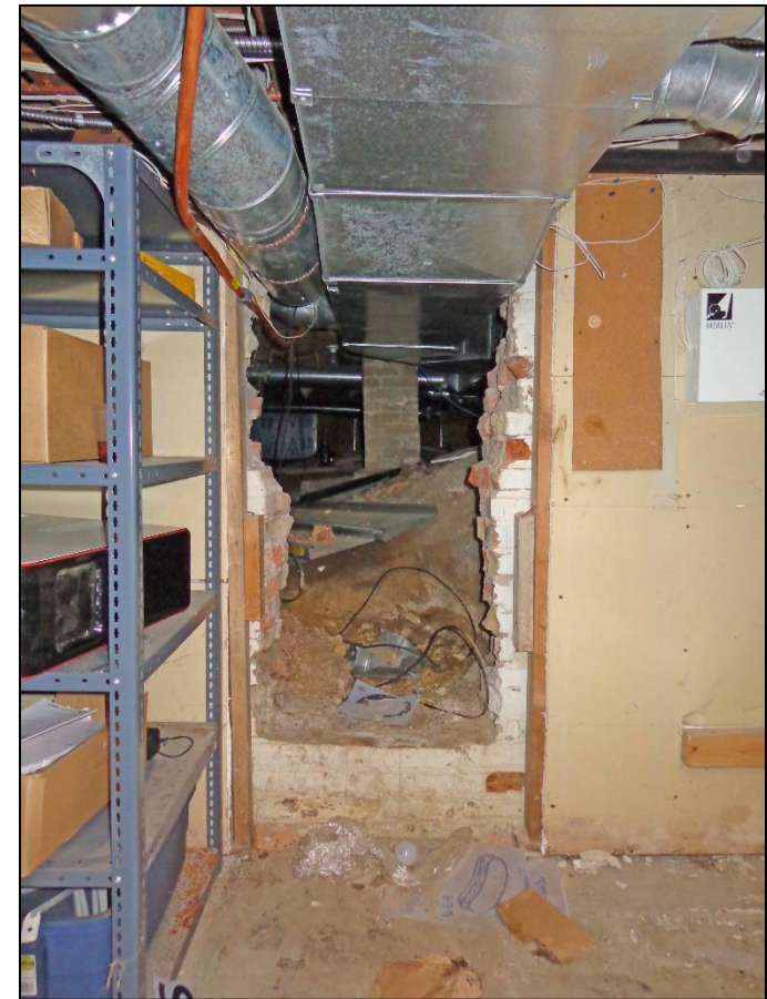
4. Room 1 – East Wall and access to Crawl Space.
