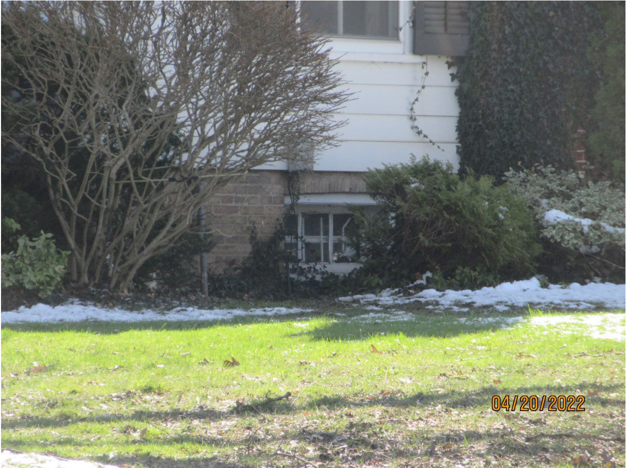
Image 8: General view of foundation and basement window
