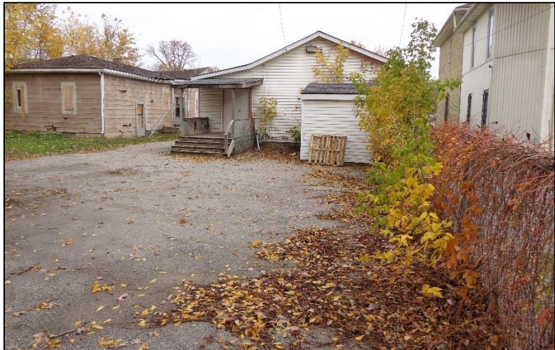
Rear Yard – View northeast from the southwest corner.
