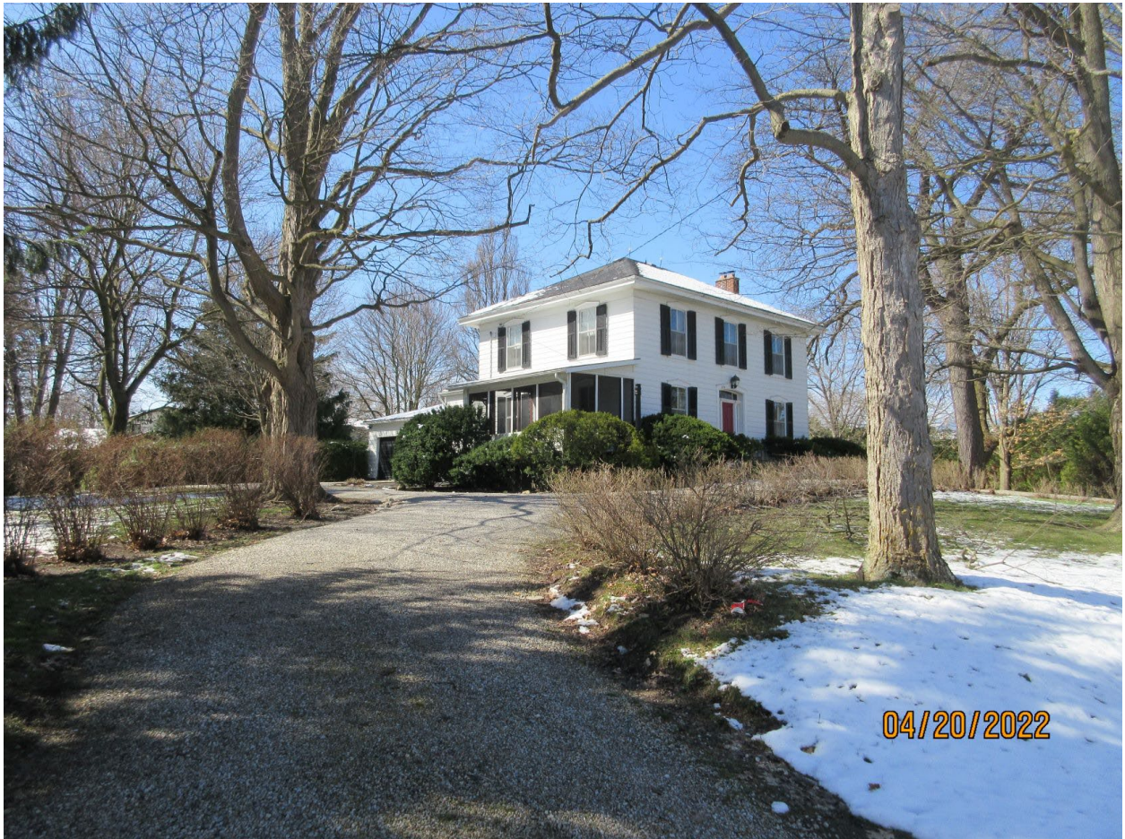
Image 4: View along curved entrance drive, looking southwest
