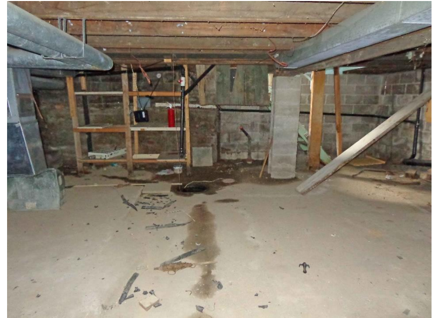
1. Room 1 – South Wall and Staircase up.
