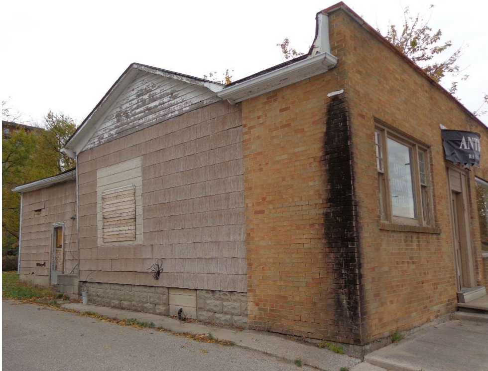
Image 5. 189 Wellington Street, façade detail-facing northeast – W. Morgan (CHIS, Jan 2021)
