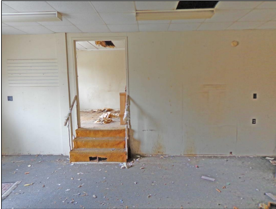
3. Room 1 – South Wall and Entrance to Room 2.
