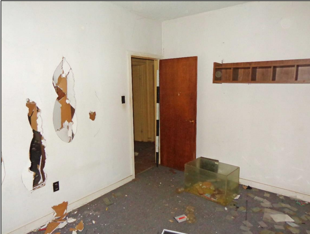
13. Room 5 – North and East Wall and Door to Hall.
