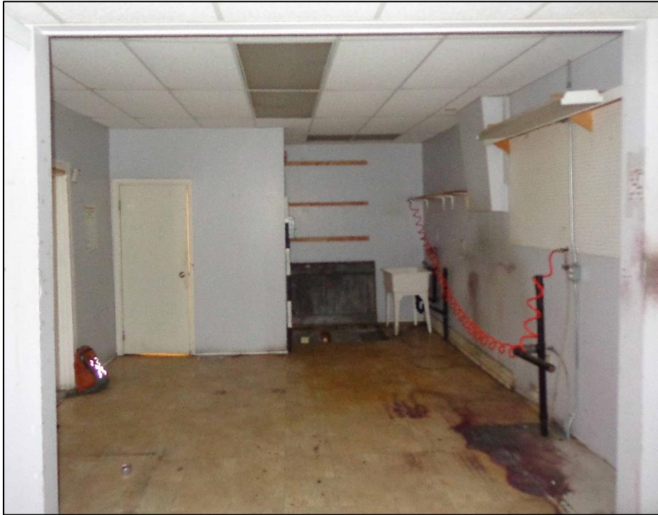
16. Room 4 – East, South and West Walls.
