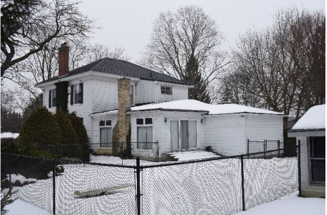
Image 6: Hip roof addition, looking northeast (Stantec, 2022 p30-plate 27)
