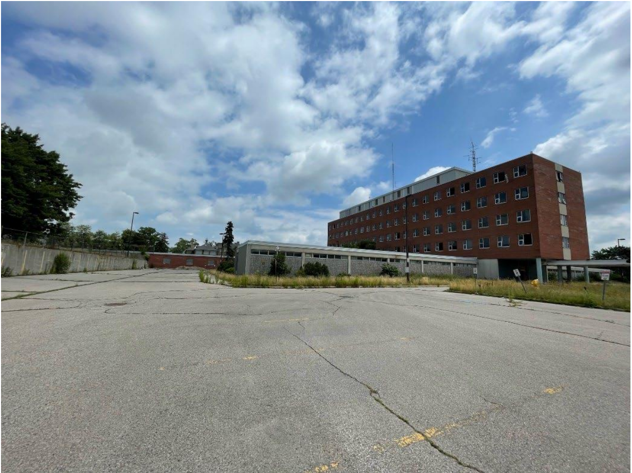
Image 7. South Pavilion Building and Extensions – as noted on project plan (including B12007, B12008, and B12010), facing east – Old Oak Properties, July 2022
