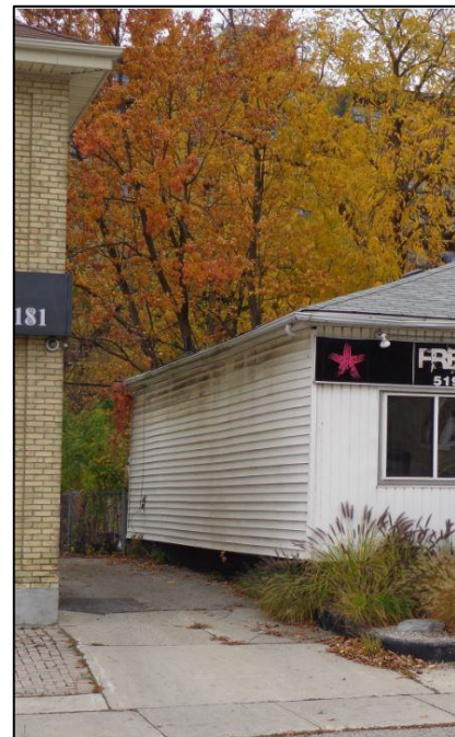
Figure 8.2 181 – 185 Wellington Street, Shared Side Yard Conditions, 2020
