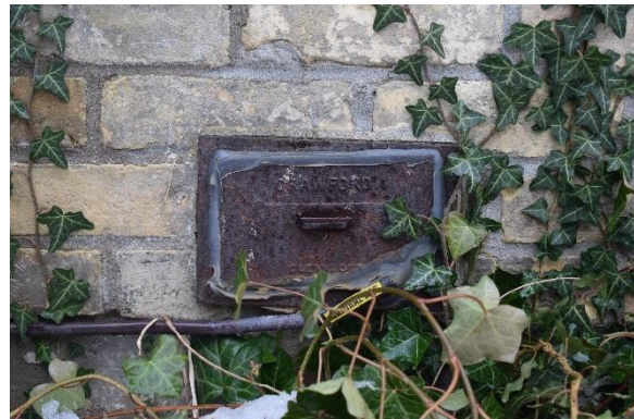
Plate 28: Clean out door, looking east
