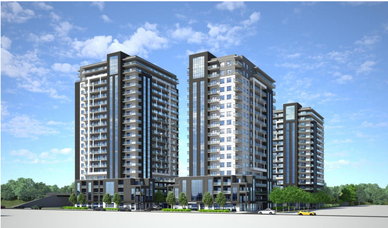
View looking southwest (Building "B" in centre).
