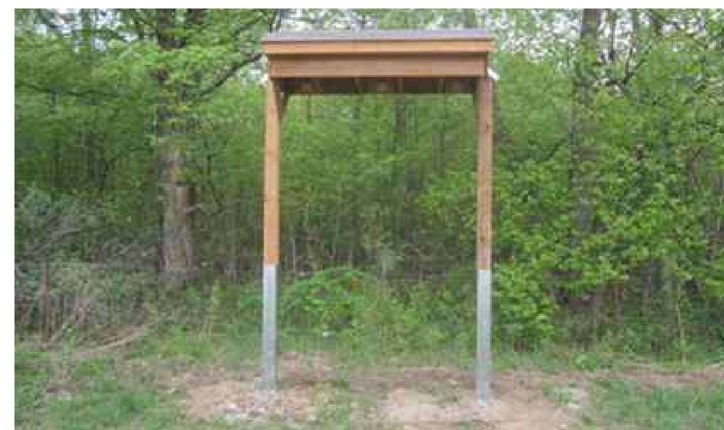
D 5 BARN SWALLOW NESTING STRUCTURE INSTALLED APRIL 2015 N.T.S.
